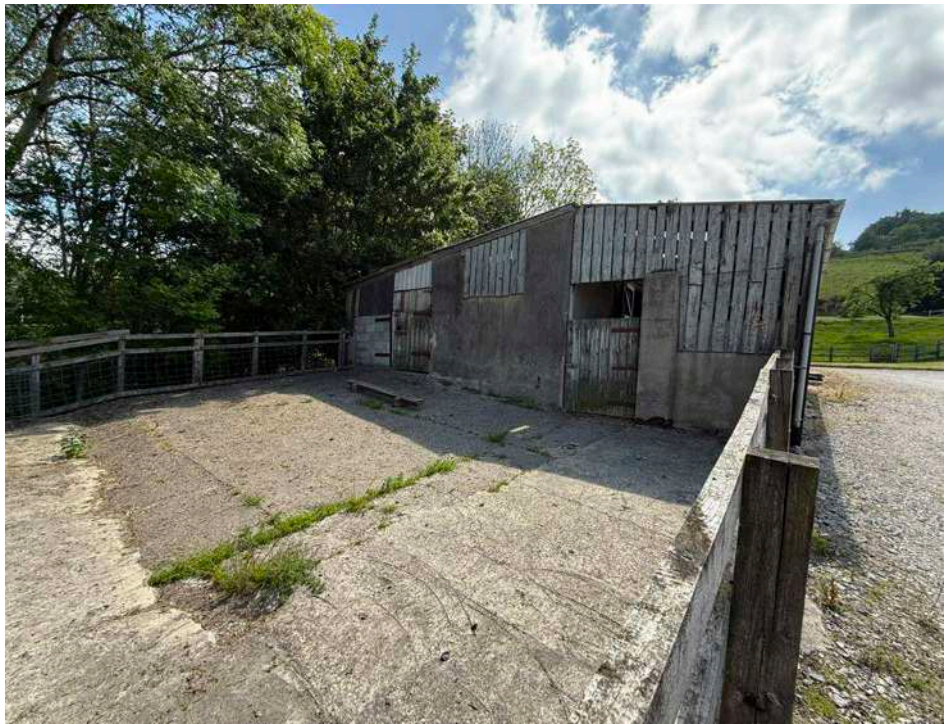
Outbuilding and stable yard.
