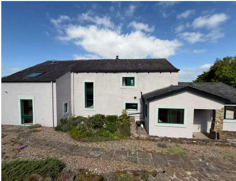
South-East elevation and rear entrance porch.
