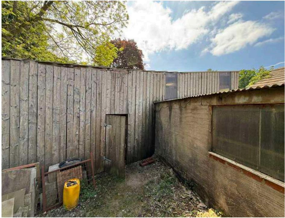
Rear of outbuilding.
