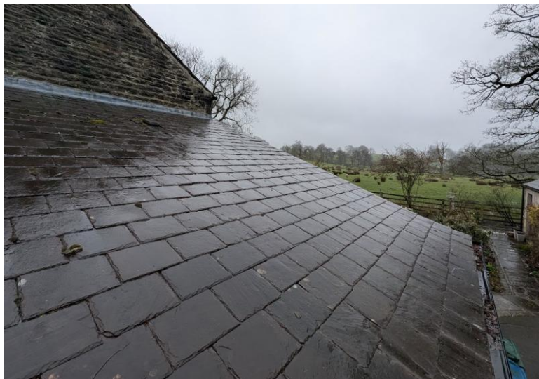
Photo 4. View of roof.
