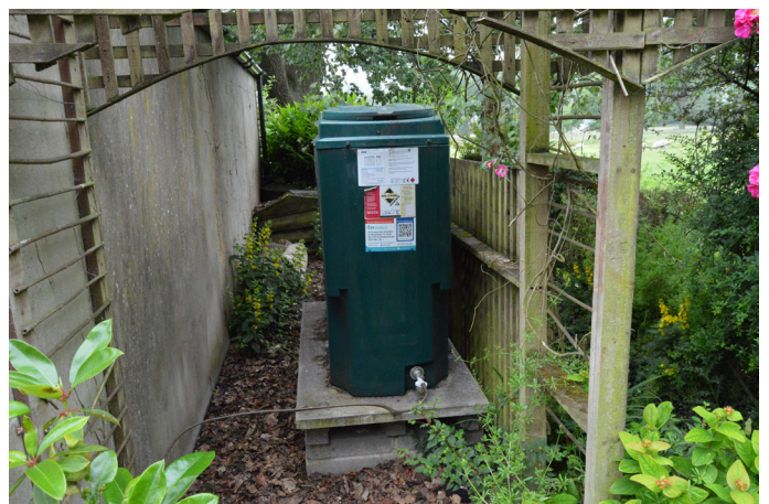
Images Showing Oil Tank Location Next to Existing Garage
