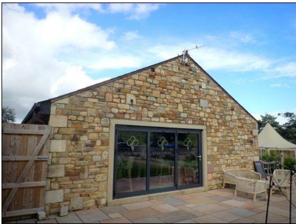
Photo 5: Building 1, southern elevation
