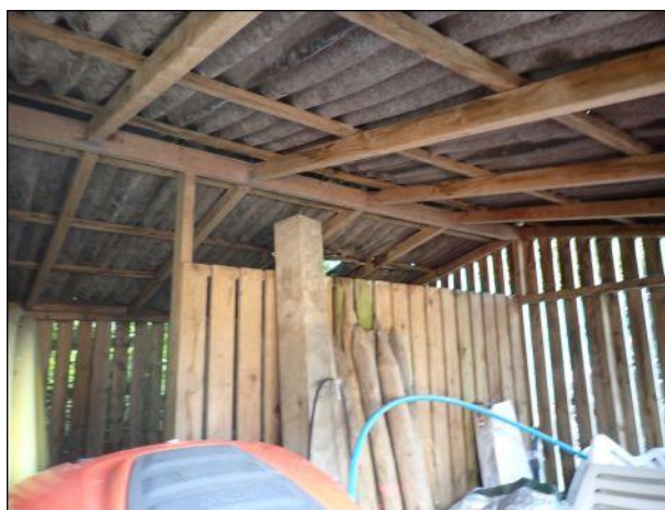
Photo 12: Building 2, internal area, northern end
