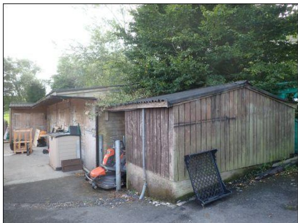
Photo 9: Building 2, northern elevation
