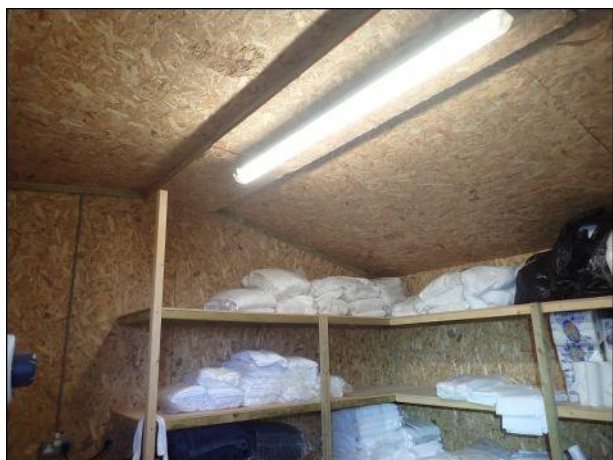
Photo 13: Building 2, middle room
