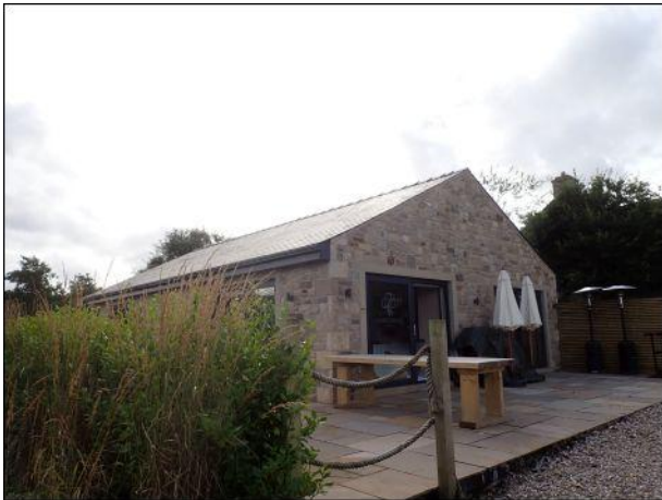
Photo 7: Building 1, northern and eastern elevations
