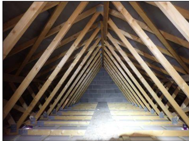
Photo 8: Building 1, roof void
