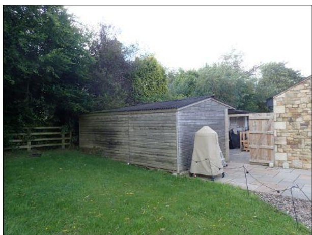
Photo 11: Building 2, southern elevation
