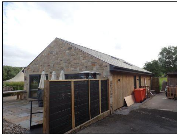
Photo 6: Building 1, western and northern elevations
