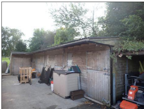
Photo 10: Building 2, eastern elevation
