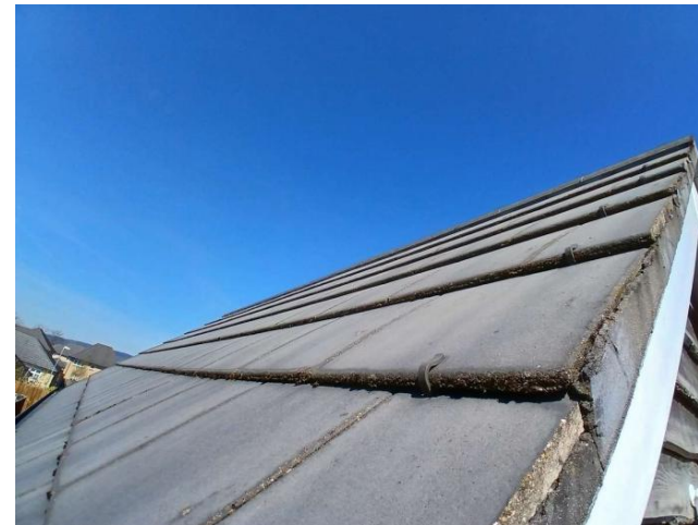
Photo 4: B2 - well sealed roof
