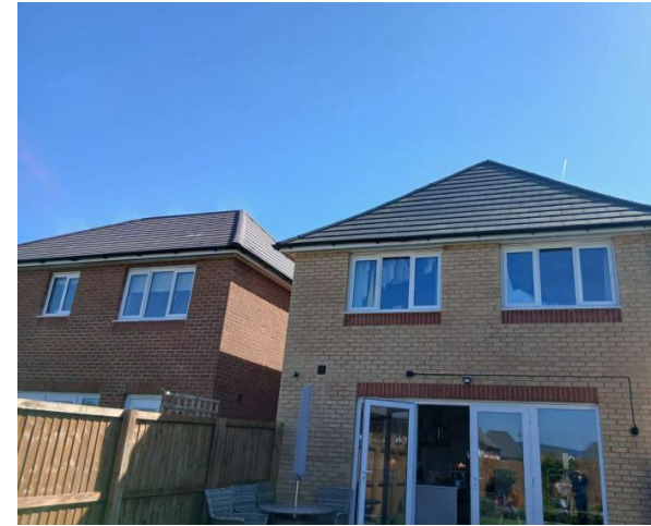
Photo 2: B1 - northwest elevation
