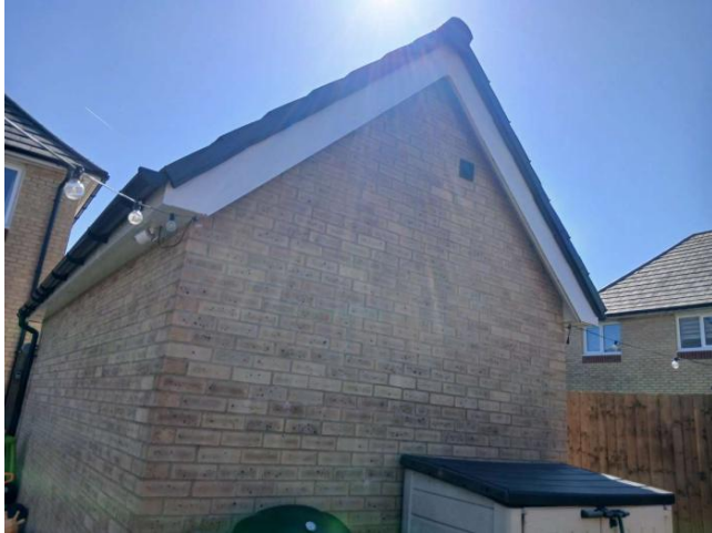
Photo 5: B2 - northwest elevation
