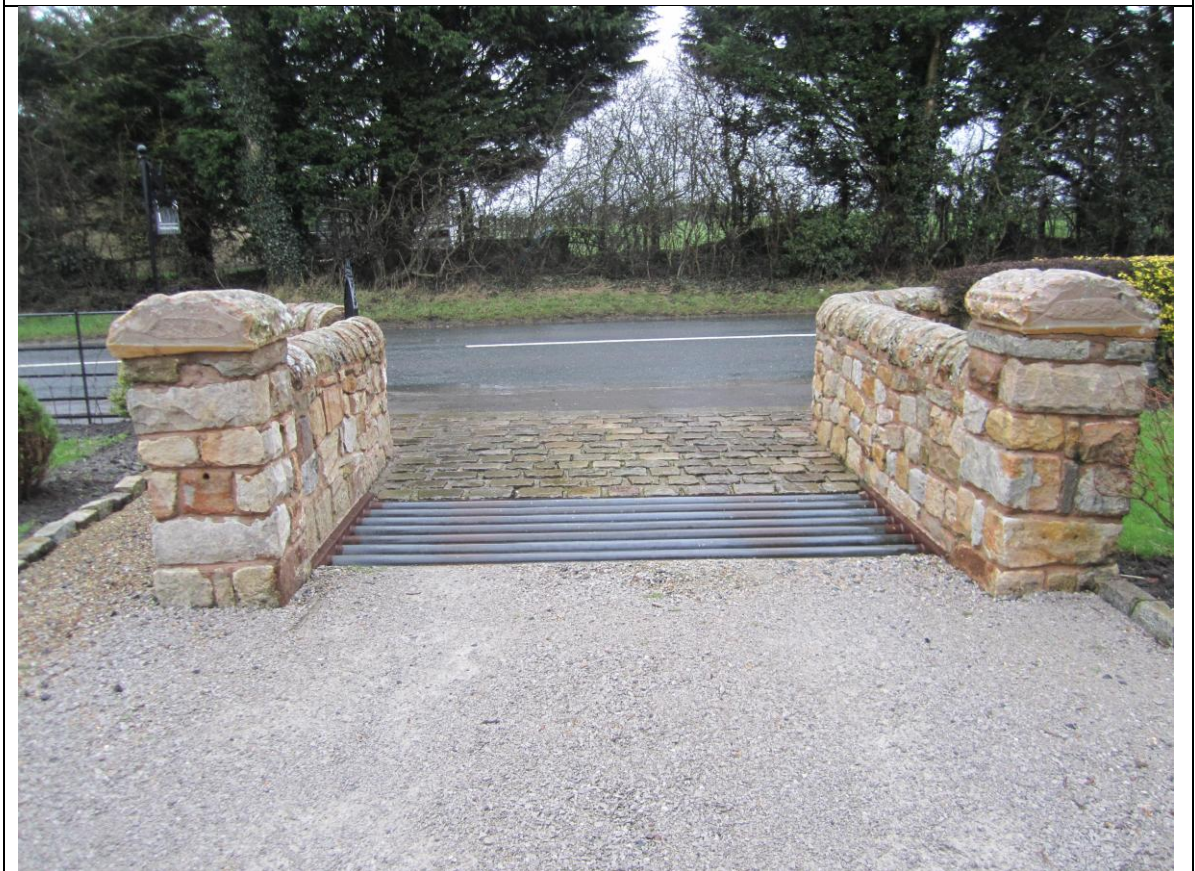
2 Setts and cattle grid at the site access onto Chipping Road
