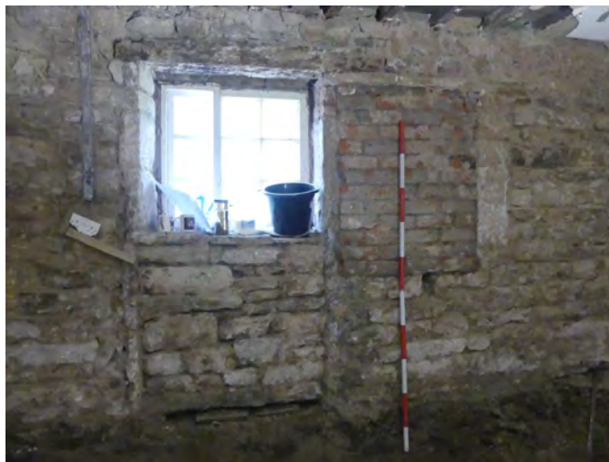
Plate 22 (left): Change in wall build of south-east elevation, Room G3, viewed from the north-west
