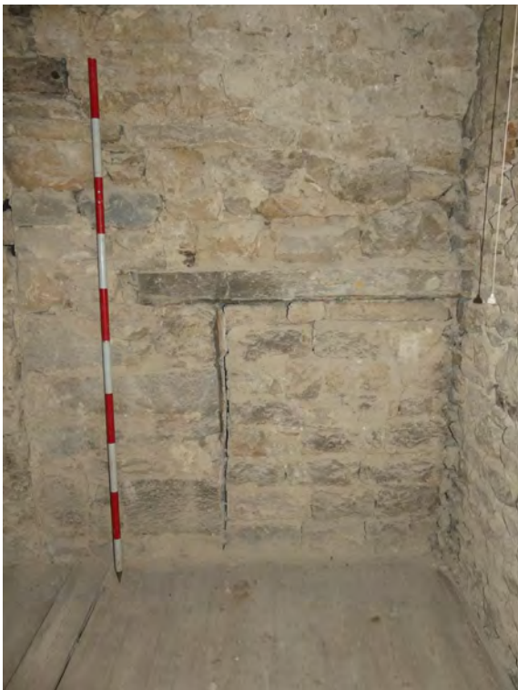
Plate 64 (left): Blocked opening, north-east of the north-west elevation, Room F6, viewed from the south-east
