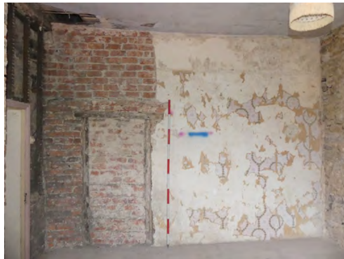
Plate 68: South-west elevation, Room F6, viewed from the north-east
