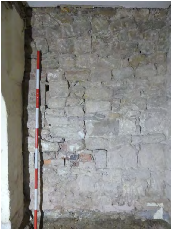
Plate 8 (left): Blocked opening on the north-east side of the north-west elevation of Room G1, viewed from the south-east
