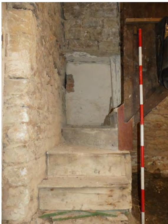
Plate 17 (left): Blocked doorway in alcove, north-east side of the south-east elevation, Room G2, viewed from the north-west
