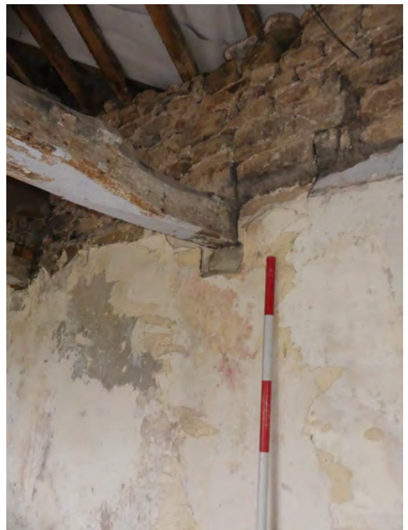
Plate 75 (left): Wall plate and raised wall line on the south-west side of the north-west elevation, Room A3, viewed from the east
