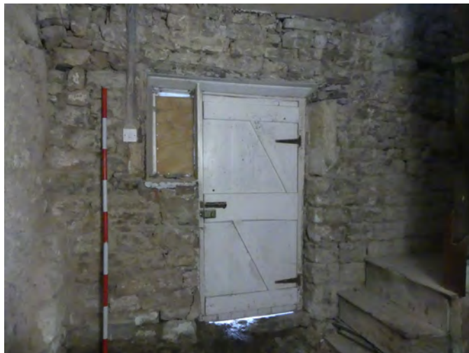
Plate 15 (left): North-west elevation, Room G2, showing blocked window, viewed from the south-east
