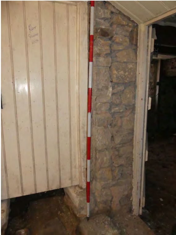
Plate 12 (left): Joining fabric visible on the north-east jamb of the doorway in the south-east elevation, Room G1, viewed from the south-west
