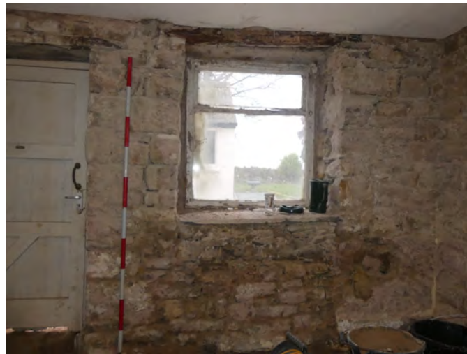
Plate 14: Window in the south-west elevation, Room G1, viewed from the north-east
