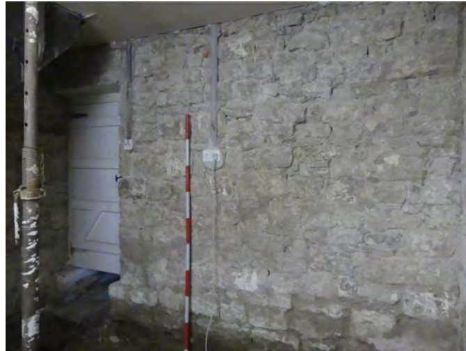
Plate 19: South-west elevation, Room G2, viewed from the north
