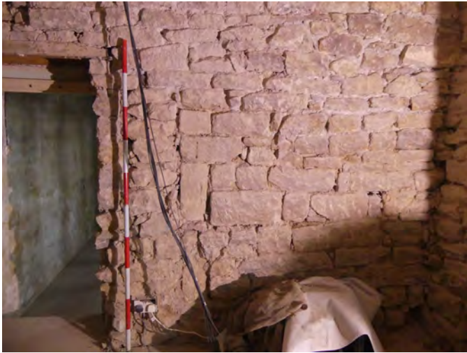
Plate 53 (left): Possible butt joint, south-west side of the south-east elevation, Room F1, viewed from the north-west
