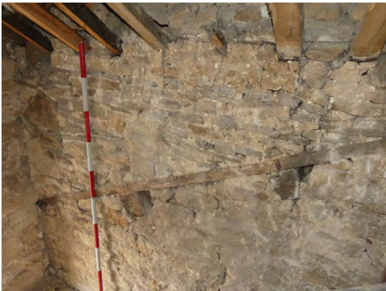
Plate 75 (left): Wall plate and raised wall line on the south-west side of the north-west elevation, Room A3, viewed from the east
