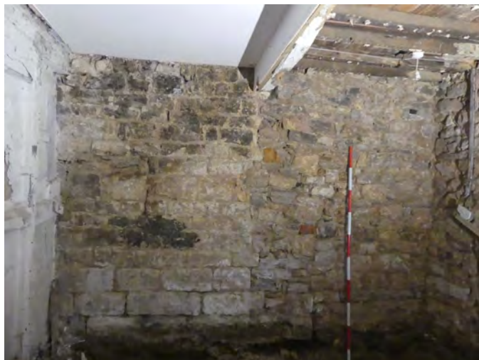
Plate 22 (left): Change in wall build of south-east elevation, Room G3, viewed from the north-west
