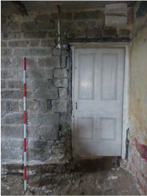
Plate 32 (left): Inserted doorway on the north-east side of the north-west elevation, Room G5, viewed from the south-east
