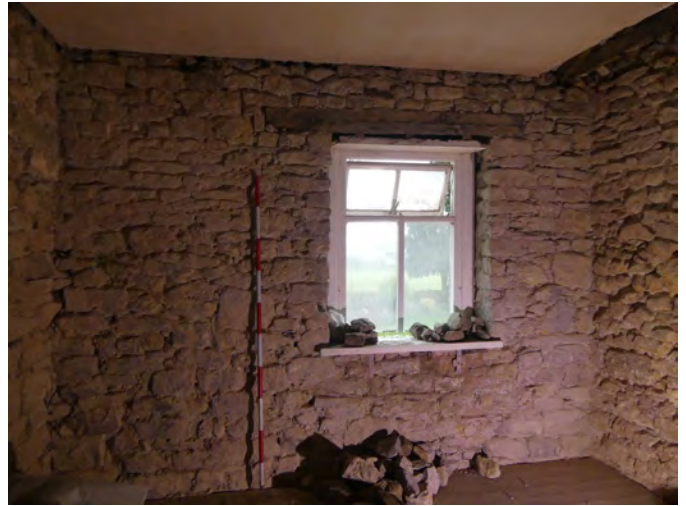
Plate 53 (left): Possible butt joint, south-west side of the south-east elevation, Room F1, viewed from the north-west
