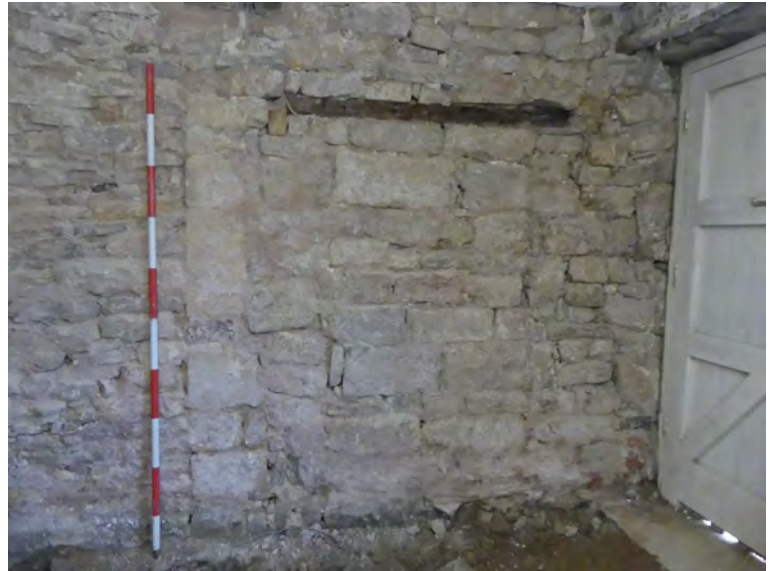
Plate 12 (left): Joining fabric visible on the north-east jamb of the doorway in the south-east elevation, Room G1, viewed from the south-west
