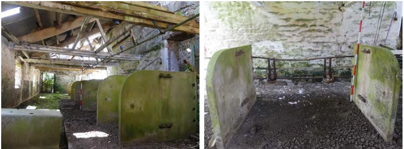
Plate 194 (left): General view of the trusses and stall in G4 from the south-east
