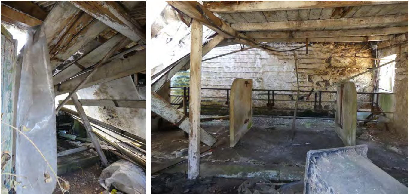
Plate 159 (left): East side of G2, viewed from the north-east
