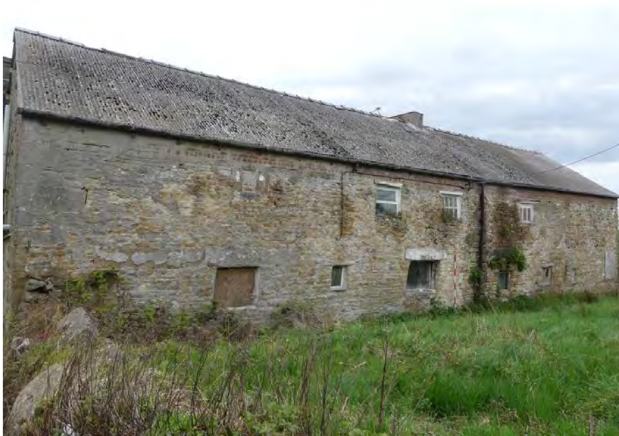
Plate 8: North external elevation of the farmhouse, viewed from the north-east
