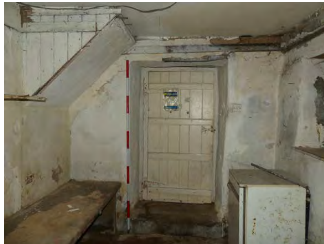
Plate 87: General view of the west elevation of G7 from the east
