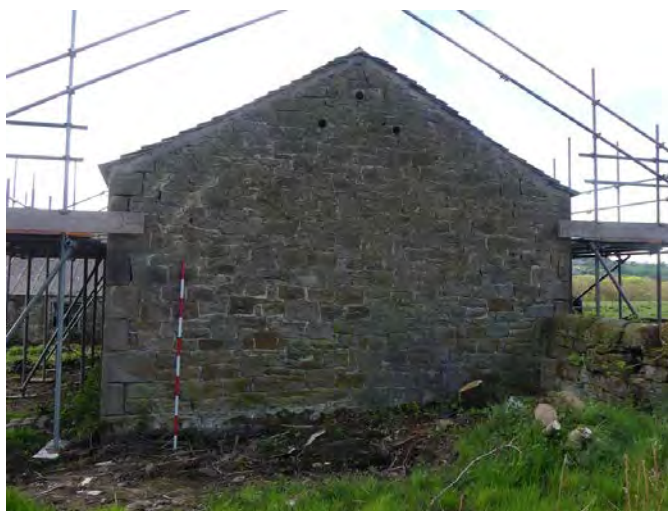
Plate 212: General view of the north external elevation of Outbuilding 1 from the north
