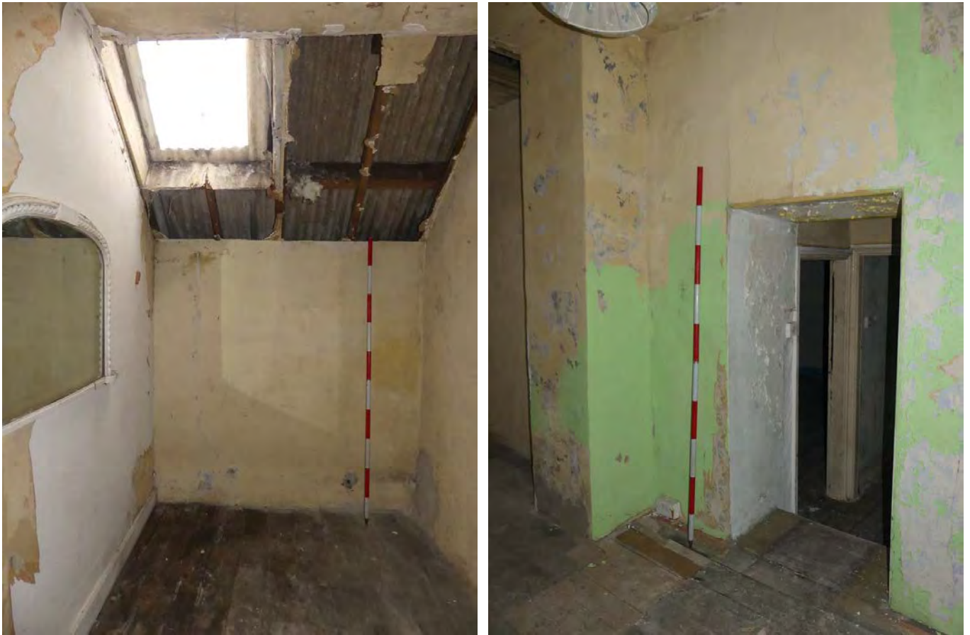
Plate 113 (left): West side of the south elevation of F4, viewed from the north
