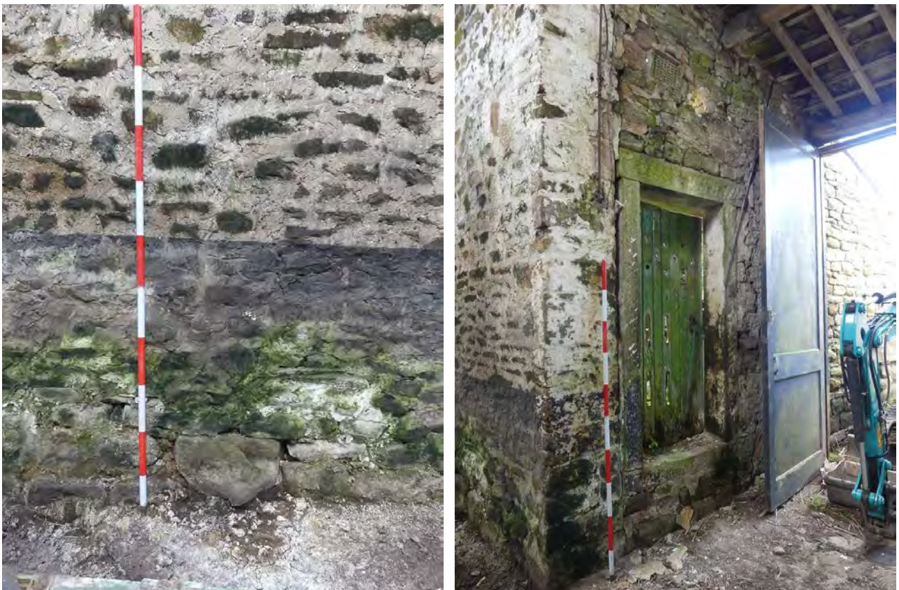
Plate 178 (left): Projecting stone at the base of the north elevation of G3, viewed from the south
