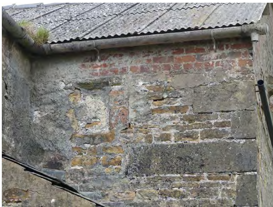
Plate 32: Small, high window in the west external elevation of the farmhouse above the outshut/porch, viewed from the west
