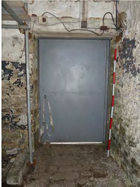
Plate 226: South door in the east elevation of G1, viewed from the west
