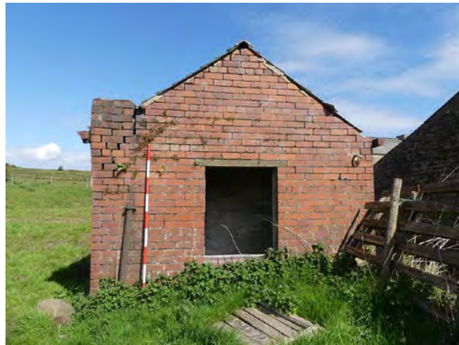
Plate 232: General view of the south external elevation of Outbuilding 2 from the south
