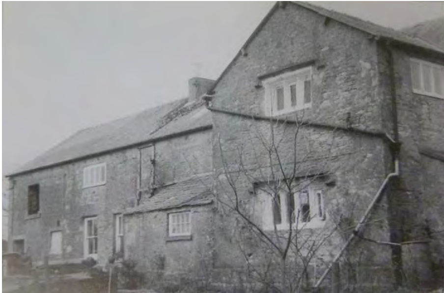
Plate 7: Photograph of the front of the farmhouse at Lower Reaps Farm (after Summersgill, facing 104)
