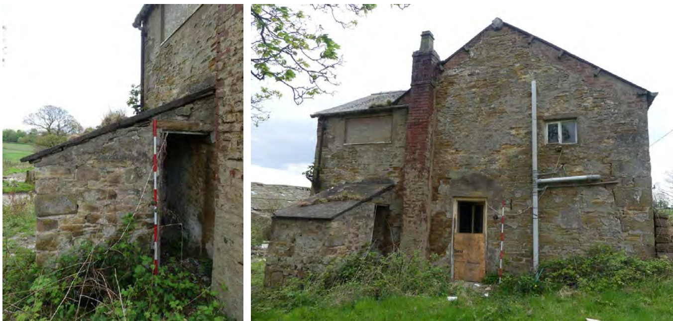
Plate 17 (left): North elevation of the outshut, viewed from the north
