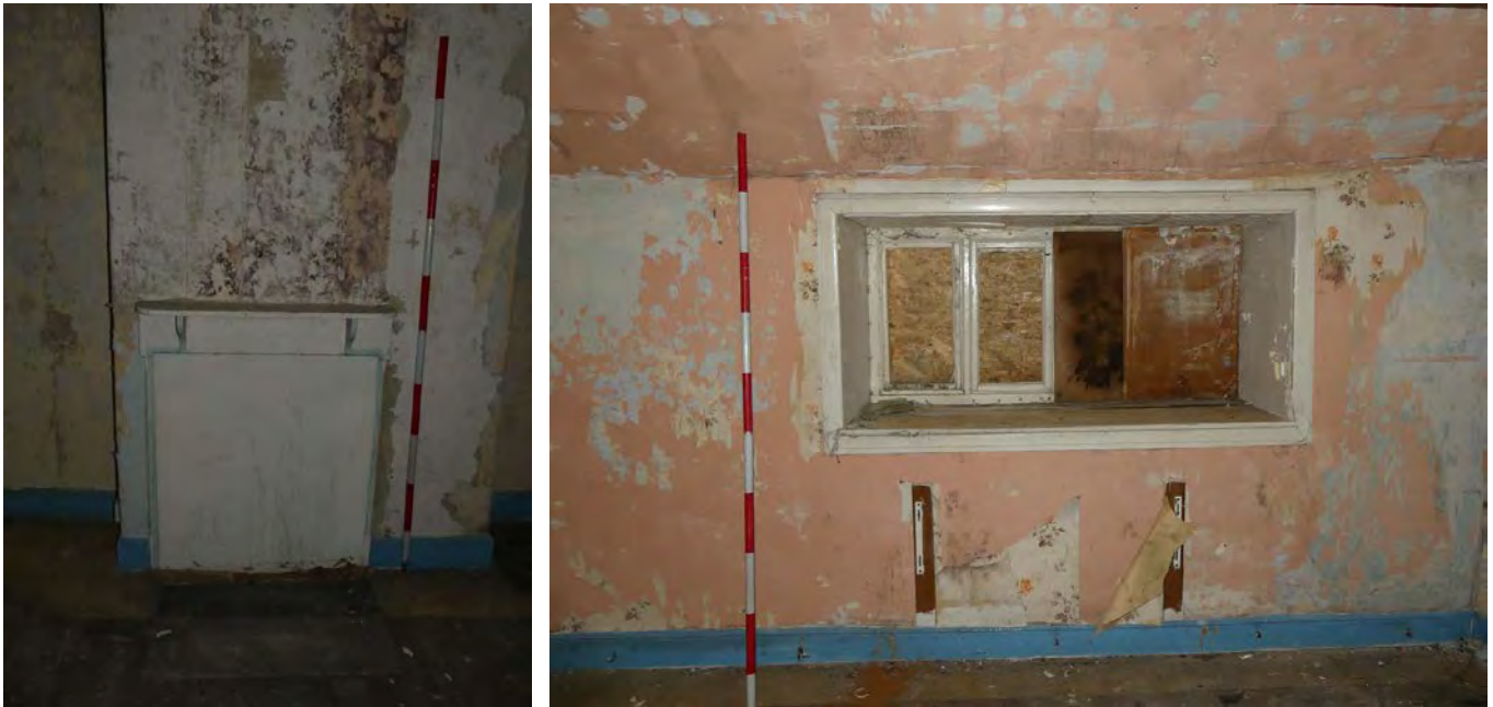
Plate 107 (left): Fireplace in the east elevation of F3, viewed from the west
