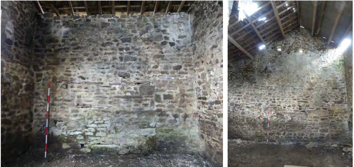
Plate 184 (left): General view of the east side of the north elevation of G3, viewed from the south
