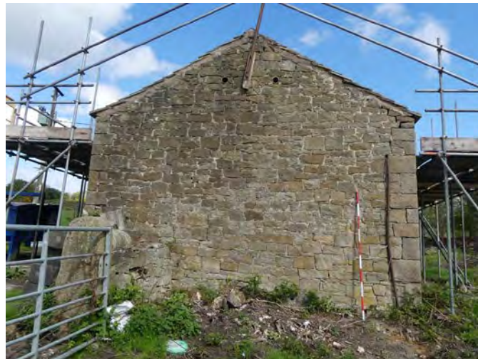
Plate 217: General view of the south external elevation of Outbuilding 1, viewed from the south
