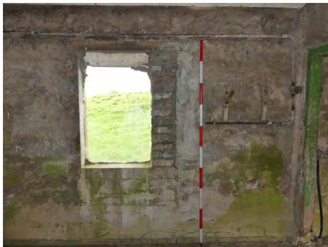
Plate 246: General view of the north side of the west elevation of G2 from the east
