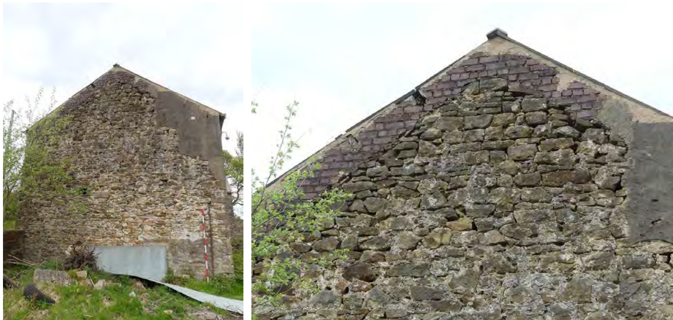
Plate 30 (left): General view of the west external elevation of the farmhouse from the west
