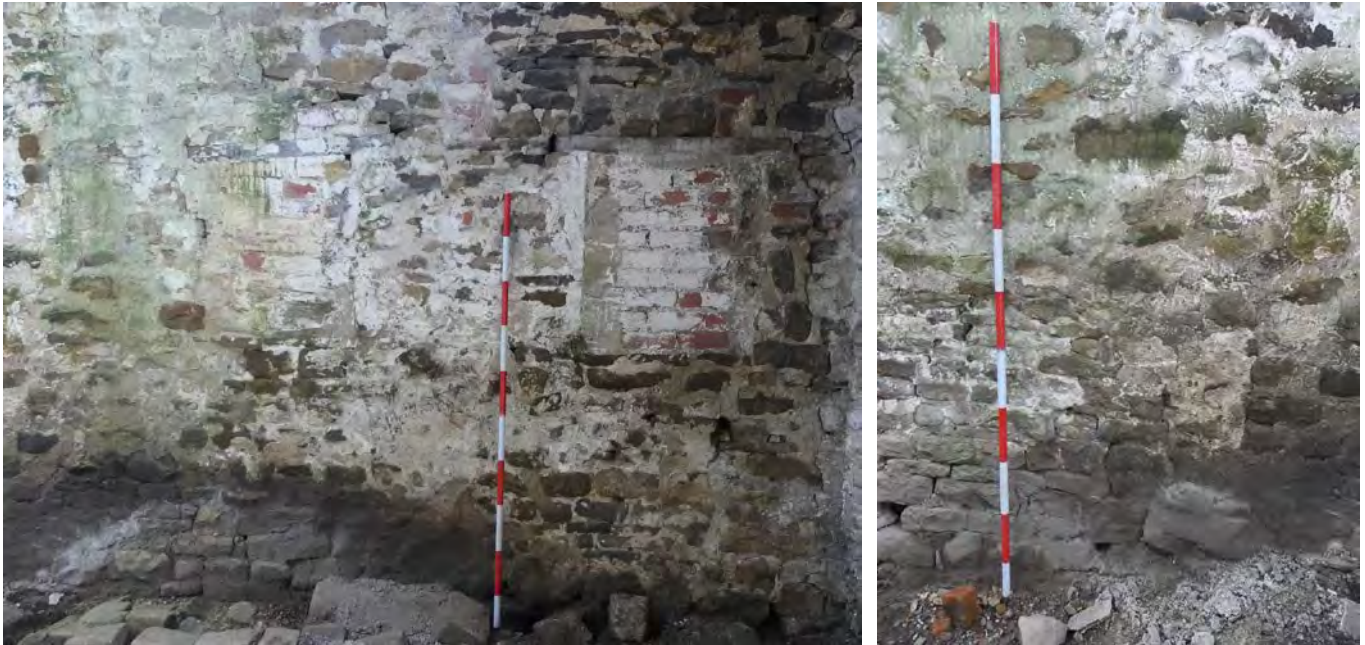
Plate 192 (left): Blocked windows to the south side of south elevation of G3, viewed from the north
