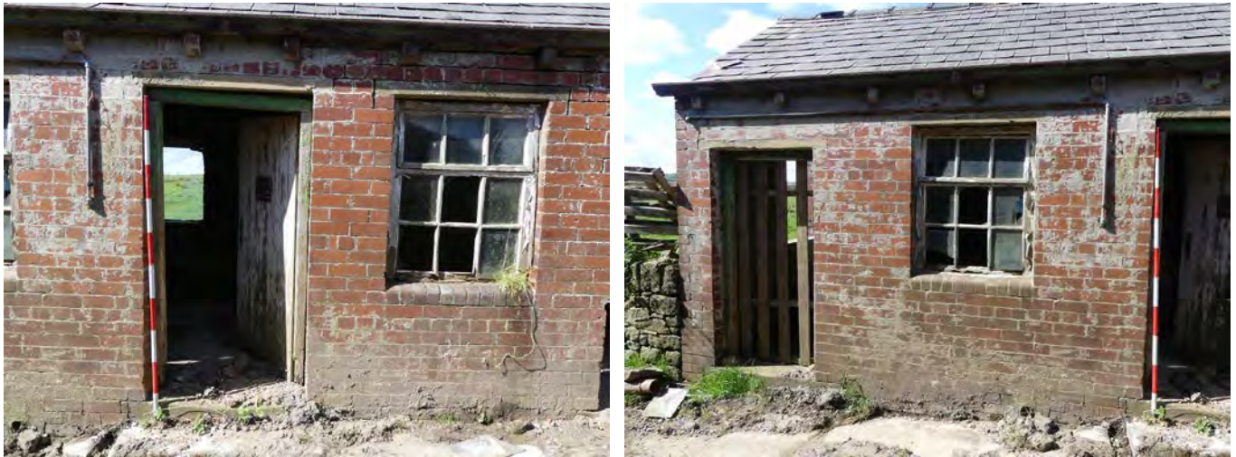
Plate 230 (left): Centre of the east external elevation of Outbuilding 2, viewed from the east
