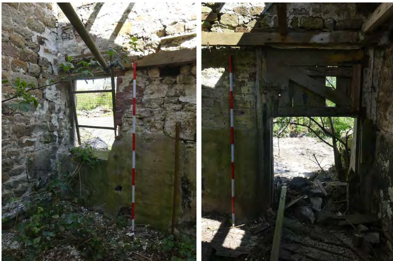
Plate 204 (left): Lower window in the east elevation of G4, viewed from the west
