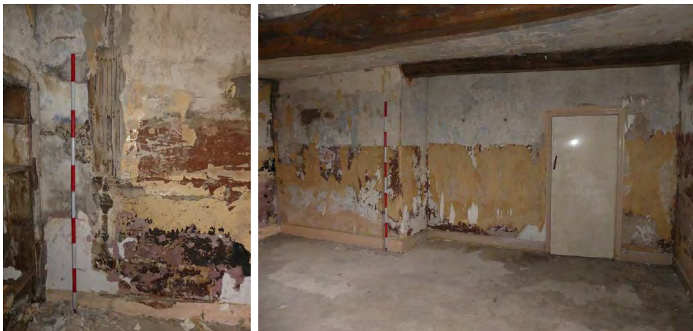
Plate 61 (left): Blocked area in the north elevation of G3, viewed from the south
