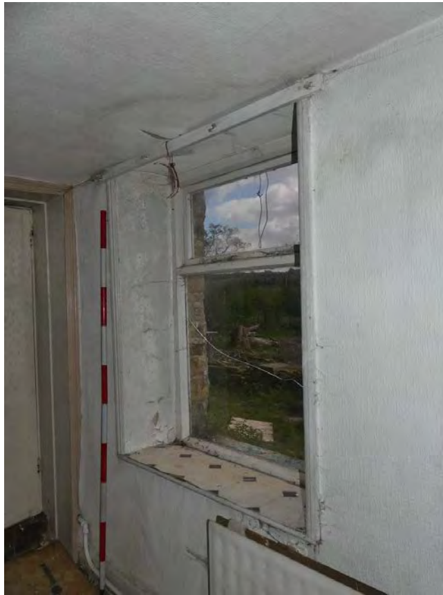
Plate 56: East window in the south elevation of G3, viewed from the north-west
