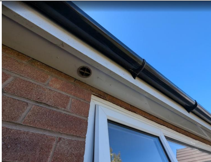
Photo 5. Example of tight-fitting soffits.
