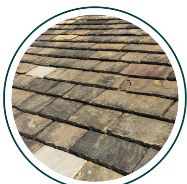
Local stone slate roof
