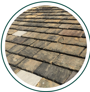
Local stone slate roof
