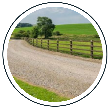
1 Existing permeable access track with soft landscaping
