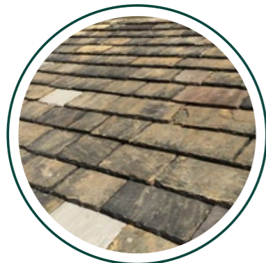
Local stone slate roof
