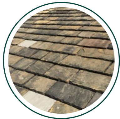
Local stone slate roof
