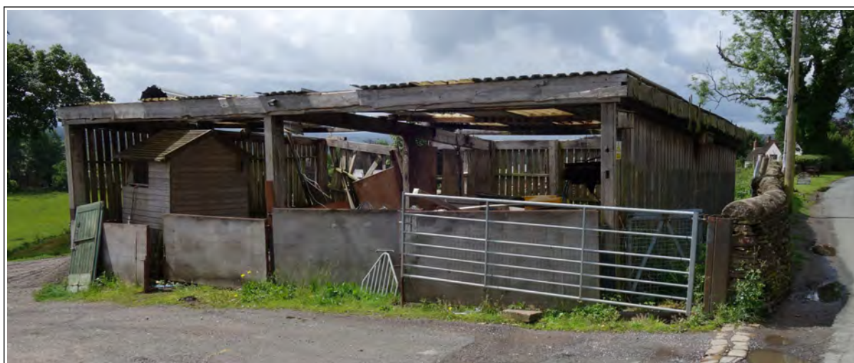
Photo 1: Existing building: north-east end
