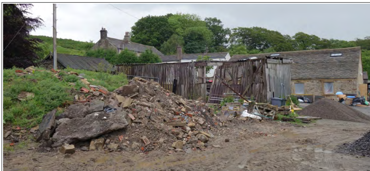
Photo 3: Site of proposed new building, illustrating detachment from settings of barn and listed farmhouse
