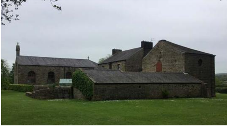
Photo | Reverse view towards Shippen, Piggery, Barn, Presbytery and Church.
