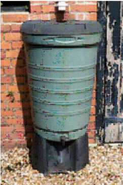
RAINWATER BUTTS FOR GARDEN IRRIGATION
