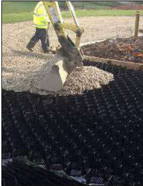
Figure A3.4: Cellweb® geo-cellular confinement sheets being installed.
