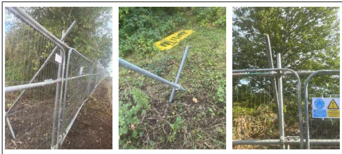
Figure A3.1: Examples of scaffold framework temporary tree protection fencing.
