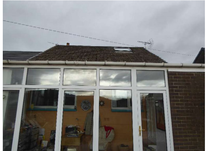
Rear SE elevation, general view.
