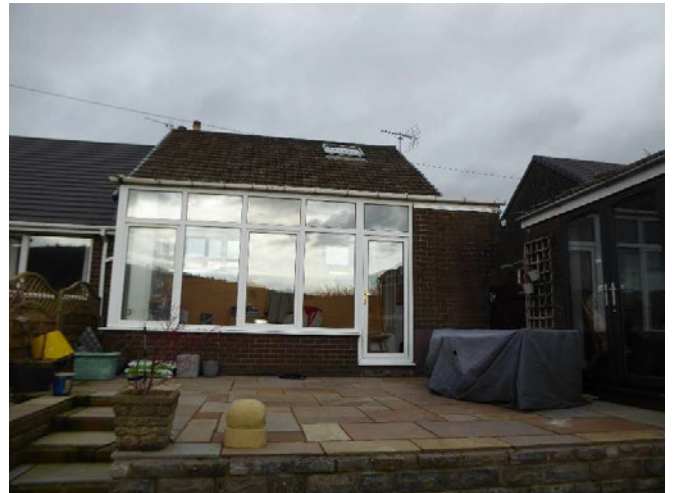
Rear SE elevation, general view.
