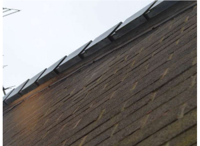
Side NE elevation showing roof ridge overhang sealed tight to brickwork.
