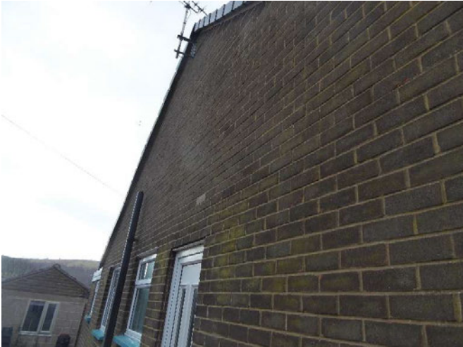
NE side elevation general view.
