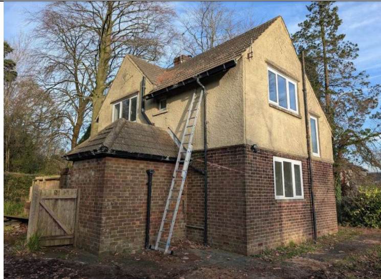
Photo 1. West and south aspects (area of proposed extension).
