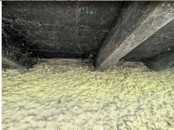
Photo 5. Example of sealed roof eaves on north aspect.
