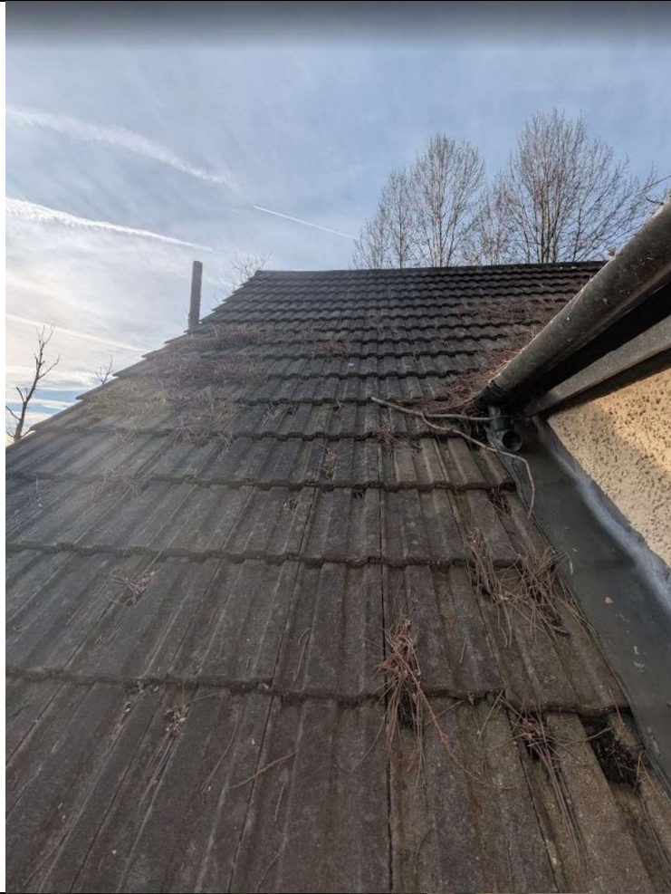
Photo 6. Roof in area of proposed extension.
