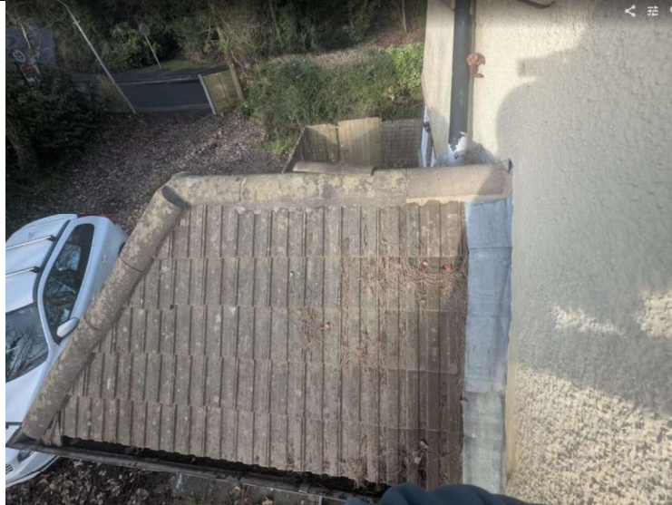
Photo 7. Roof of single storey section on west aspect.
