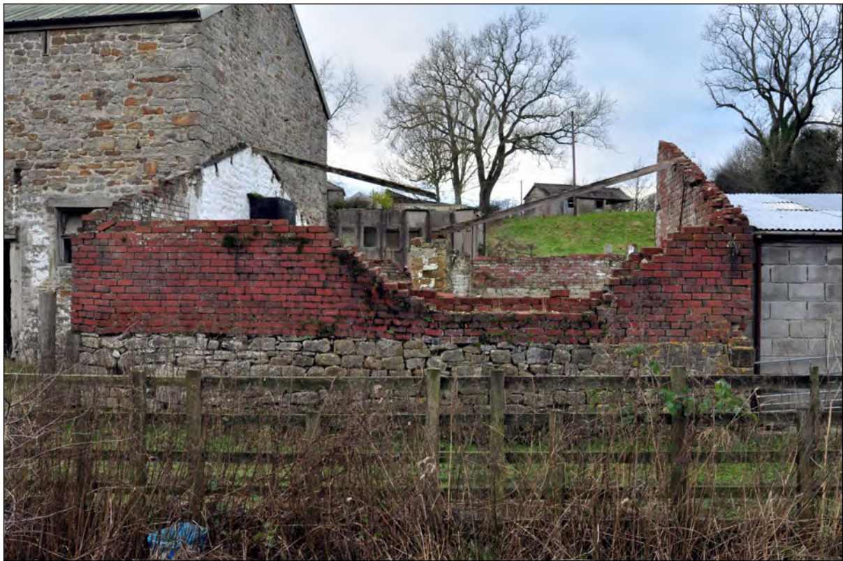
Photo 11: Building C: south-east elevation
