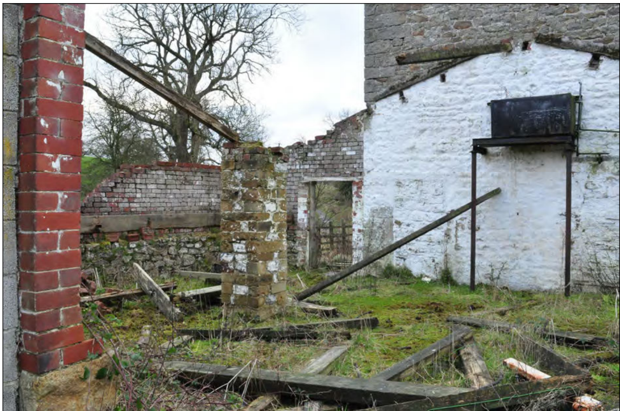
Photo 12: Building C: interior, looking south
