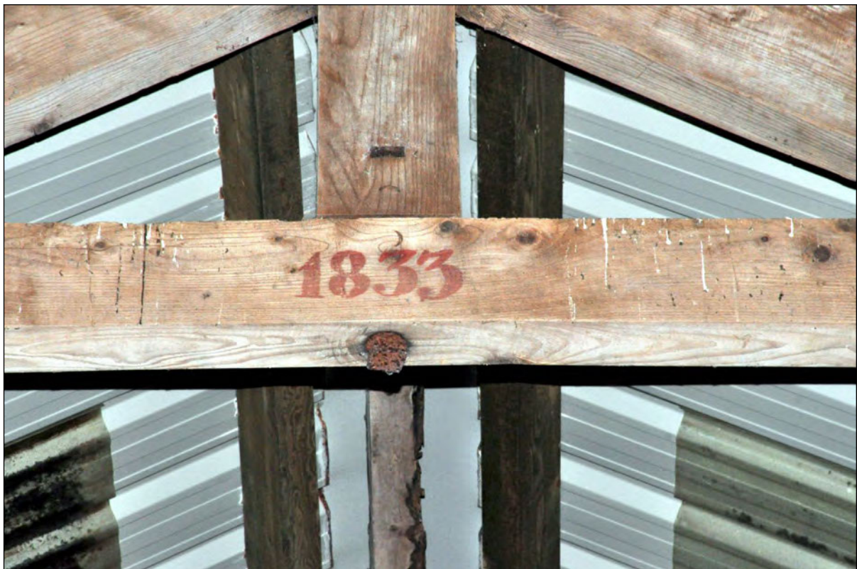
Photo 8: Building A: dated roof timber
