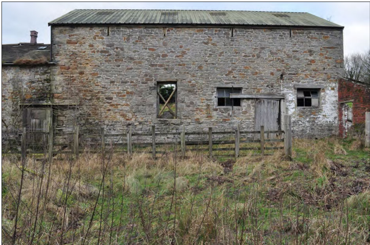
Photo 5: Building A: south-east elevation.
