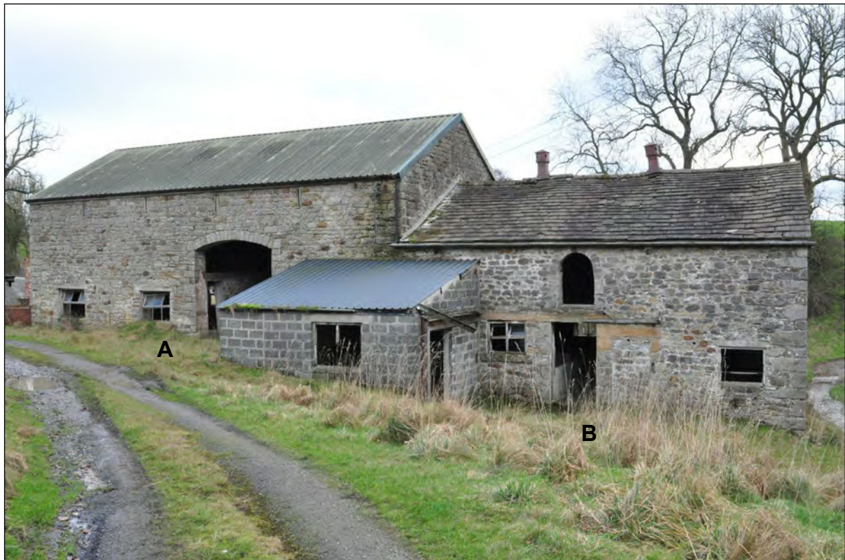
Photo 3: North-west elevations of buildings A (left) and B (right)
