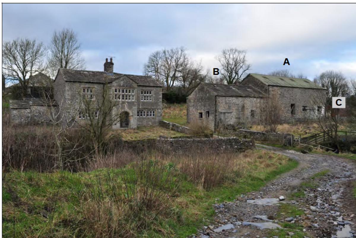
Photo 1: Key view of the Hall, looking north from public footpath. Farm buildings proposed for conversion to right (A, B & C).
