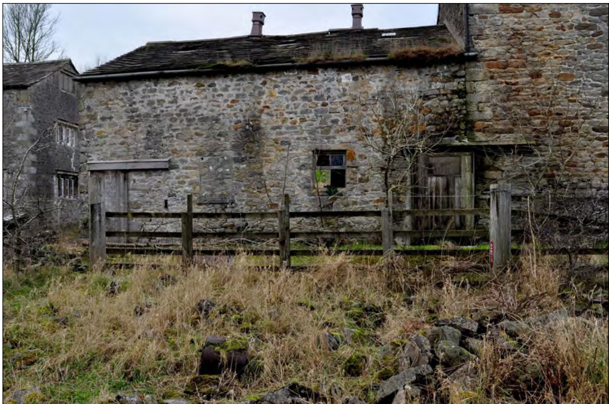
Photo 10: Building B: south-east elevation
