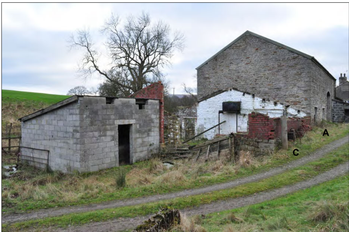
Photo 6: Buildings A & C, looking south. Modern building in foreground would be cleared as part of landscaping
