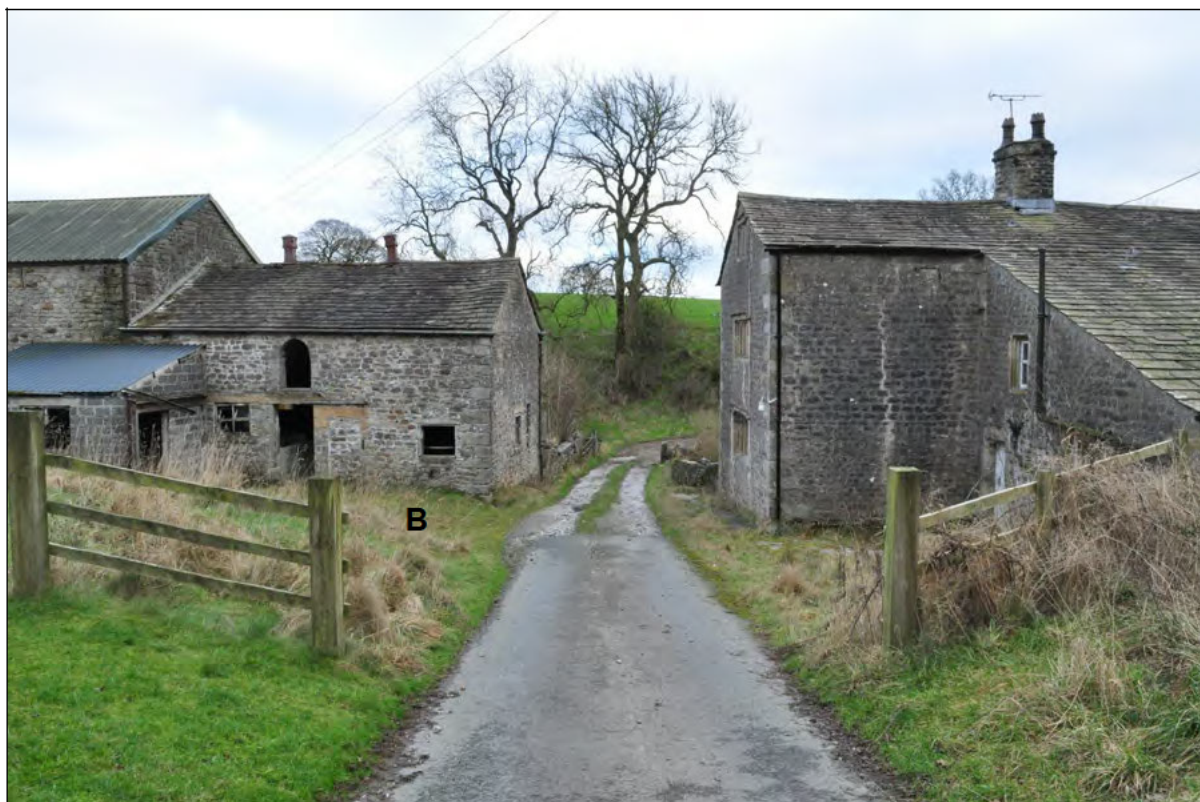
Photo 2: View from the north-west: track separating Fooden Hall (right) from building B (left)
