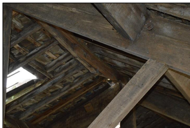
PL23: View of decay and repairs undertaken the ridge beam of the roof to the south addition. It is recommended that these areas are closely inspected on erection of a safe working platform to confirm condition.
