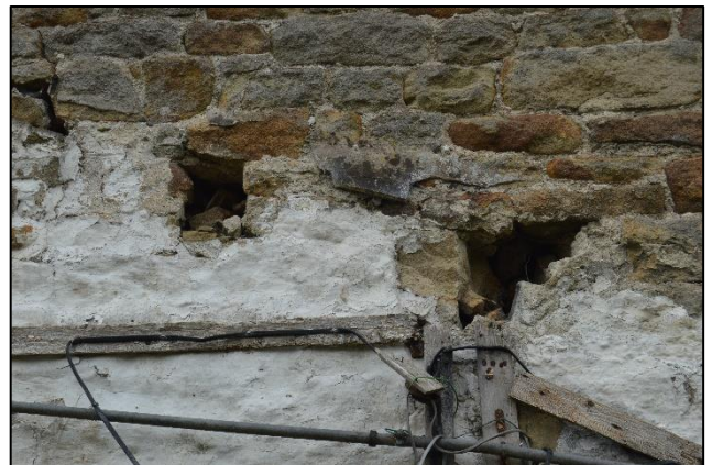
PL40: Loose / unconsolidated masonry noted to the now relict purlin sockets to the north gable of the main core of the barn. Making good is recommended and the sockets infilled with matching stonework.
