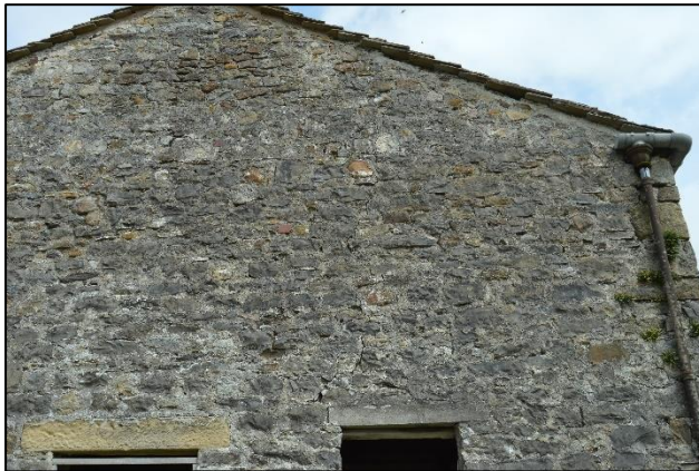
PL48: Isolated vertical cracking was noted over the east window opening to the south gable end of the south addition. The cracking was deemed to be slight (between 1mm and 5mm) to moderate (between 5mm and 15mm). A fall was also noted to the window head at this location. It is recommended that bed joint reinforcement is installed where coursing will allow i.e. stainless steel helical bars and the affected area then repointed using a lime mortar. This should then be monitored for any further evidence / re-occurrence of cracking or movement. Should any further movement / cracking occur then this will require assessment by a Structural Engineer and structural repairs undertaken as required.
