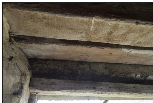
PL51: Minimal end bearings were noted to the internal timber safe lintels over the east opening to the ground floor of the south gable end of the south addition. Evidence of wood-boring insect attack was also noted, i.e. insect flight holes. It is recommended that the lintels are replaced with new lintels with a minimum end bearing of 150mm – 200mm.
