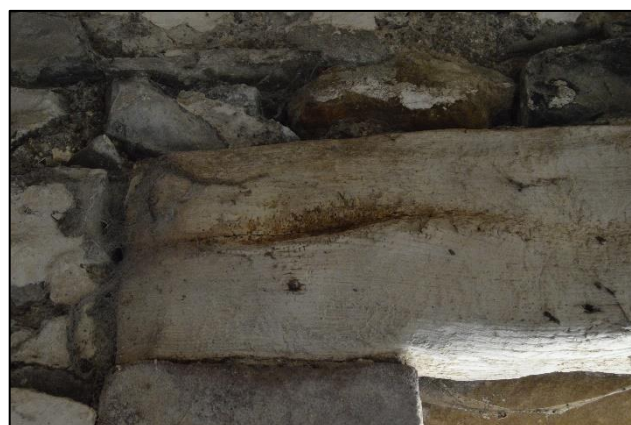
PL52: The timber safe lintel over the west opening to the opening to the ground floor of the south gable end of the south addition was noted as being slender in profile. Evidence of wood-boring insect attack was also noted, i.e. insect flight holes. It is recommended that the timber lintel is replaced.
