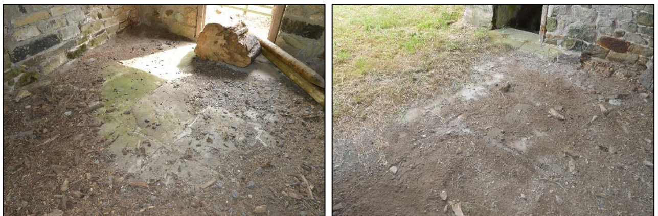
PL80: Views of the remaining stone flag flooring present to the former threshing floor to the main core of the barn.
