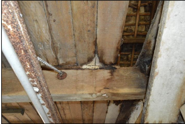
PL86: View of areas of decayed timber floor boards present to the suspended timber floor to the northern half of the south hayloft.
