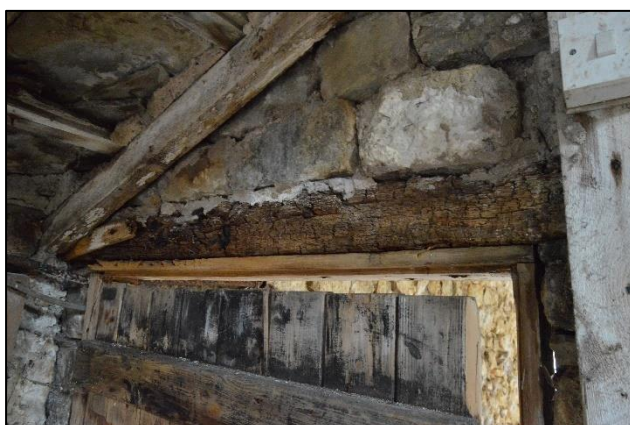
PL70: Decay and fungal growth were noted to the south timber lintel over the internal door opening between the main core of the barn and the hayloft to the south addition. Replacement is recommended.
