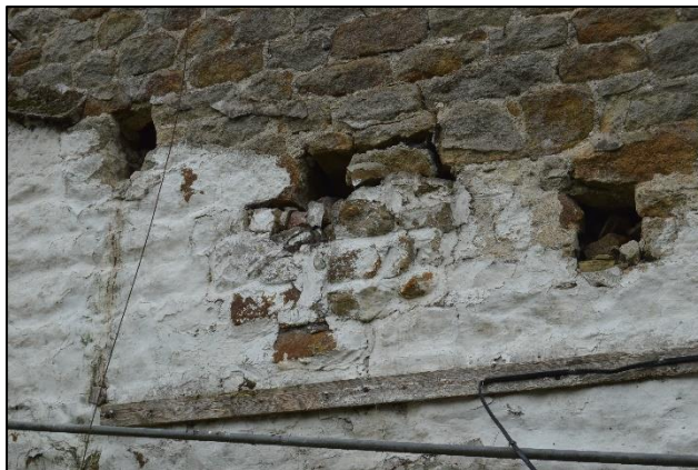
PL40: Loose / unconsolidated masonry noted to the now relict purlin sockets to the north gable of the main core of the barn. Making good is recommended and the sockets infilled with matching stonework.
