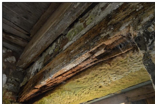
PL57: Decay was noted to the internal timber safe lintel over the external doorway to the north end of the east elevation of the south addition. It is recommended that the lintel is replaced.
