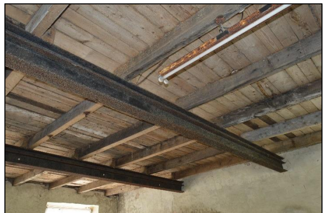
PL88: View of the suspended timber floor structure and steel supporting beams to the north hay loft, likely caused by past water ingress from the roofing above.
