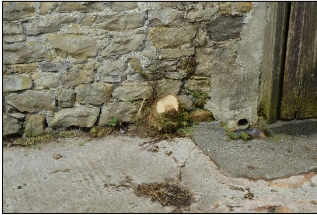
PL47: A number of tree / sapling stumps were noted to the wall base of the east elevation. It is recommended that stumps are fully removed as well as the underlying root matrices.
