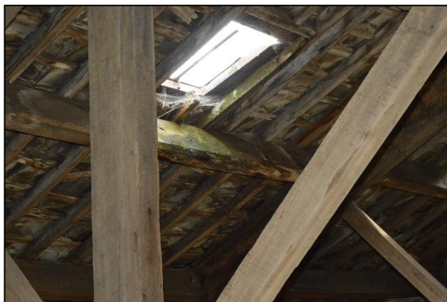
PL22: Staining noted to the timber purlins located beneath the roof lights to the east roof slope of the south addition, suggesting potential water ingress at these locations. This has led to some decay of the timbers below the roof light locations and it is recommended that these areas are closely inspected on erection of a safe working platform to confirm condition and full extent of decay.
