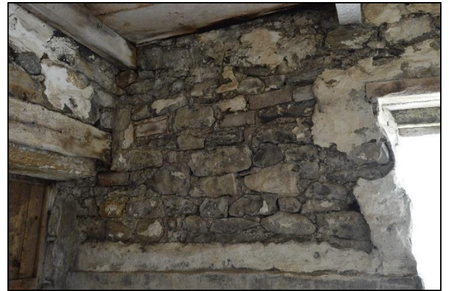
PL74: Areas of perished mortar were widely noted throughout the building and repointing using a lime based mortar is recommended. Any larger voids should be packed with mortar and gallet stones and then repointed.
