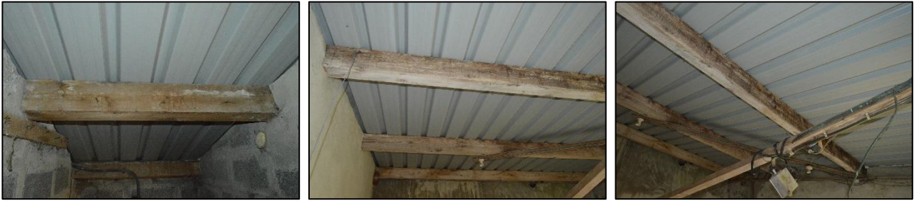
PL09: View of the timber roof structure to the west lean-to structure.
