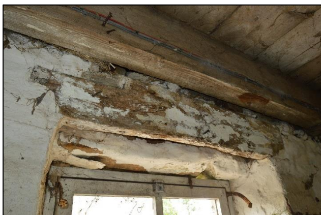
PL58: Minor decay and evidence of wood-boring insect attack was noted, i.e. insect flight holes, to the timber lintel over the ground floor window to the north end of the east elevation of the south addition, adjacent to the west lean-to structure. It is recommended that the lintel is replaced.
