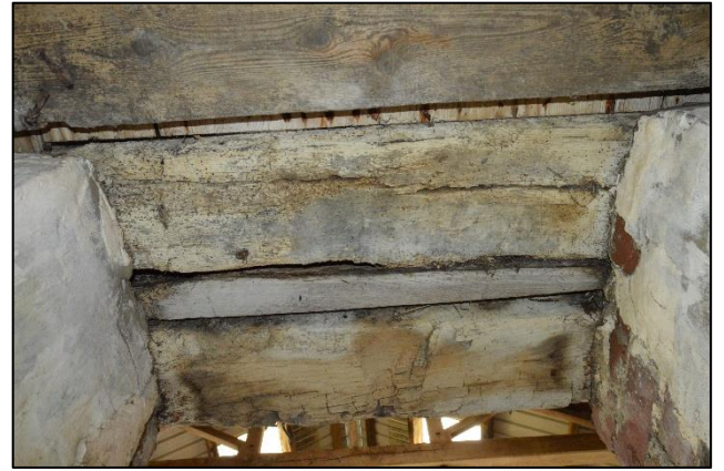
PL73: Decay and evidence of wood-boring insect attack i.e. flight holes, noted to the timber lintels over the wall opening to the north side of the main core of the barn. Replacement of the lintels is recommended.
