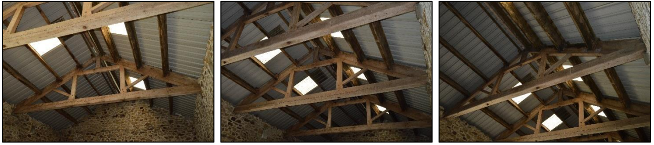
PLI 6: View of the timber queen post roof trusses and associated roof structure to the main core of the barn.
