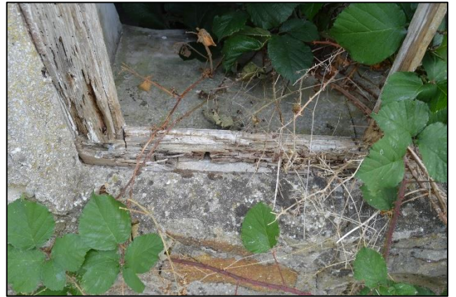
PL90: Evidence of insect attack i.e. insect flight holes and decay noted to joinery items.
