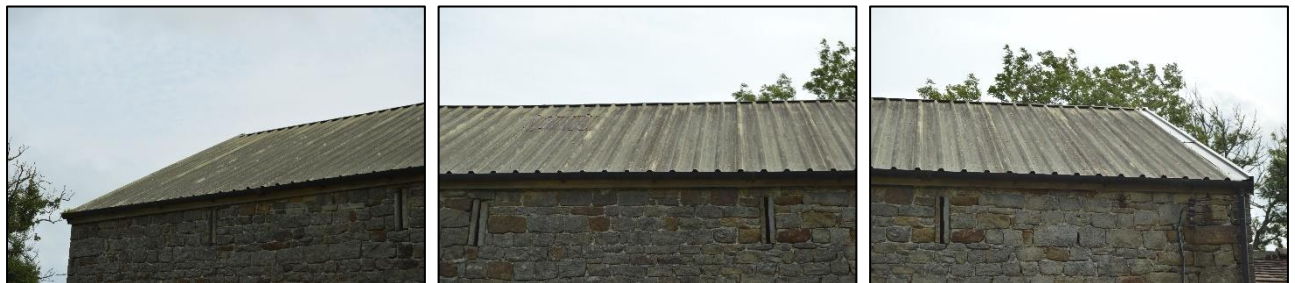
PL14: View of the profiled metal sheet roof covering to the west roof slope of the main core of the barn.
