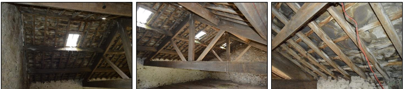
PL21: View of the roof structure to the south addition of the barn.
