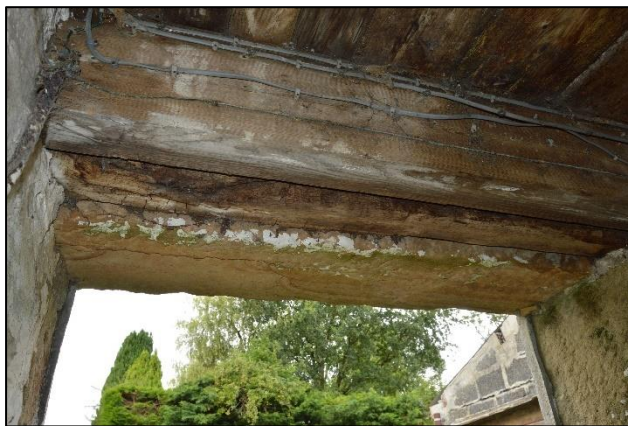
PL54: Decay was noted to the timber safe lintel located over the west elevation personnel door to the south addition. Replacement is recommended.
