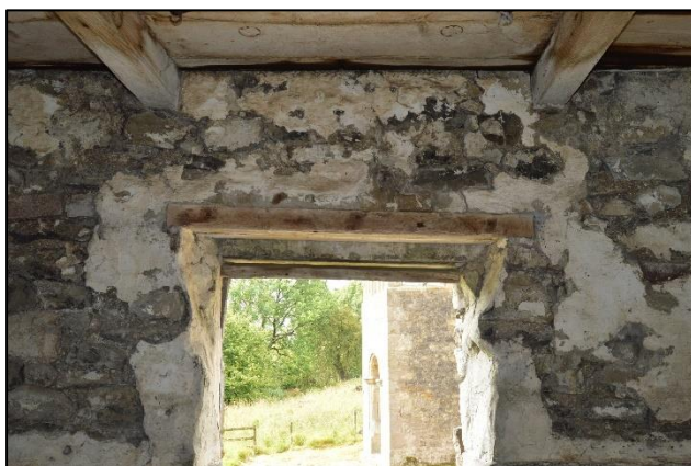
PL69: Poorly consolidated masonry was noted over the head of the east window to the south gable of the south addition. Making good is recommended to consolidate the masonry.
