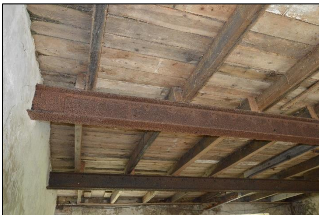
PL88: View of the suspended timber floor structure and steel supporting beams to the north hay loft, likely caused by past water ingress from the roofing above.
