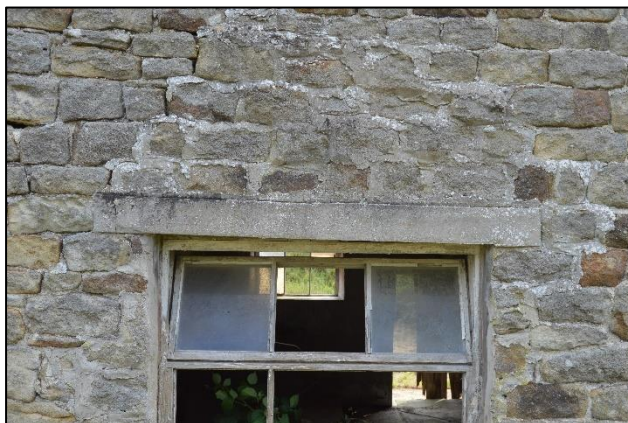
PL41: A crack noted to the lintel to a window to the ground floor of the west elevation of the main core of the barn. The front of the lintel appeared to be comprised of a cement veneer and it could not be confirmed if it was only the veneer was cracked or if the crack was also present the underlying structural support, the type, condition and adequacy of which could not be confirmed at the time of inspection.
