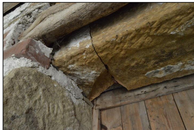
PL50: The stone lintel to the doorway at the south end of the east elevation was cracked and replacement will be required. The internal timber safe lintel was also noted as being slender in profile and was decayed. It also contained evidence of wood-boring insect attack and replacement of the timber lintel is also required.
