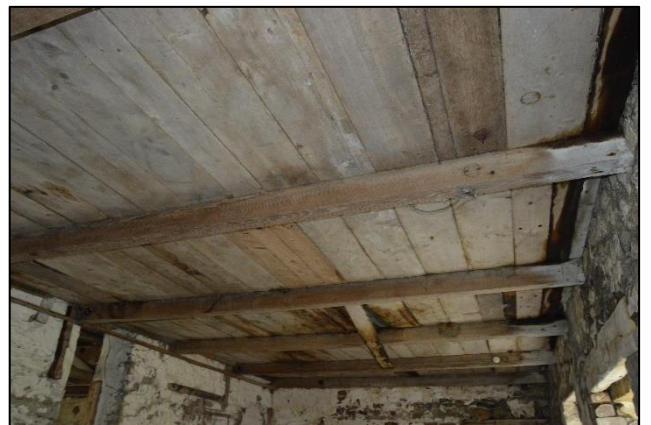
PL83: View of the suspended timber floor structure to the southern half of the south hayloft.
