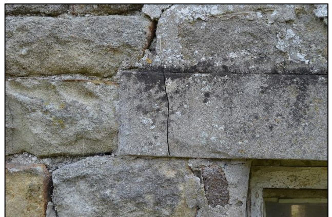
PL41: A crack noted to the lintel to a window to the ground floor of the west elevation of the main core of the barn. The front of the lintel appeared to be comprised of a cement veneer and it could not be confirmed if it was only the veneer was cracked or if the crack was also present the underlying structural support, the type, condition and adequacy of which could not be confirmed at the time of inspection.
