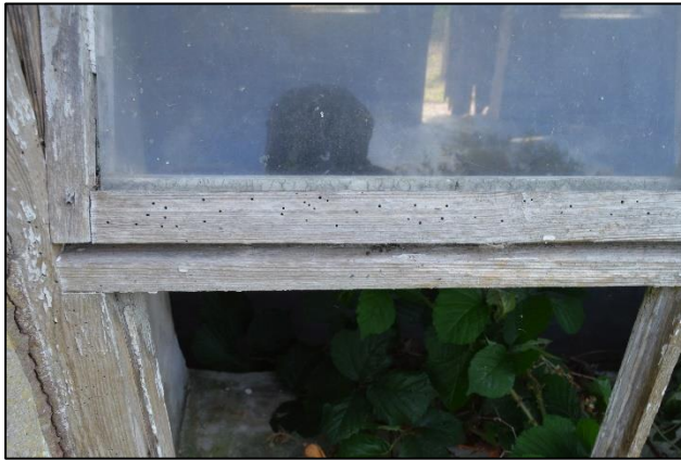
PL90: Evidence of insect attack i.e. insect flight holes and decay noted to joinery items.
