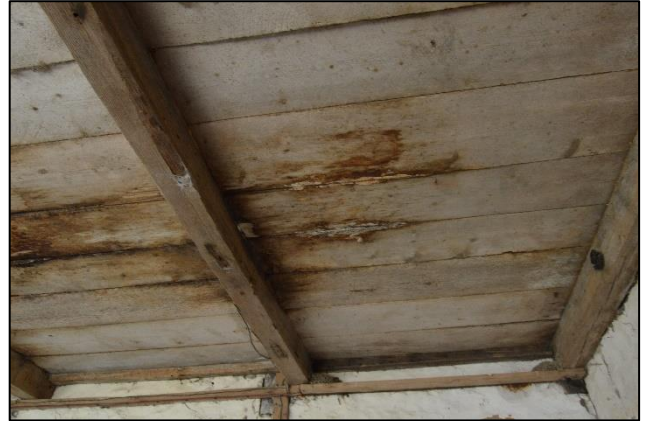
PL84: View of areas of decayed timber floor boards present to the suspended timber floor to the southern half of the south hayloft, likely caused by past water ingress from the roofing above.
