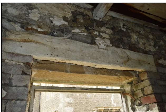
PL52: The timber safe lintel over the west opening to the opening to the ground floor of the south gable end of the south addition was noted as being slender in profile. Evidence of wood-boring insect attack was also noted, i.e. insect flight holes. It is recommended that the timber lintel is replaced.
