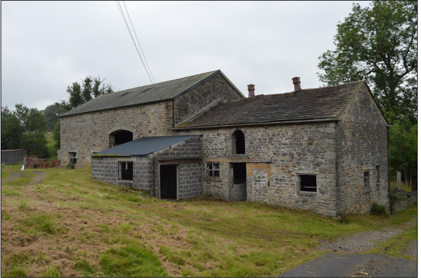
PL01: View of Fooden Hall Farm Barn from the west.
