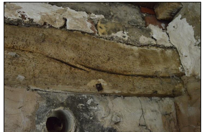
PL55: Evidence of wood-boring insect attack was noted to the internal timber safe lintel over the blocked-up door opening to the west side of the south addition, i.e. insect flight holes. It is recommended that the timber lintel is replaced.
