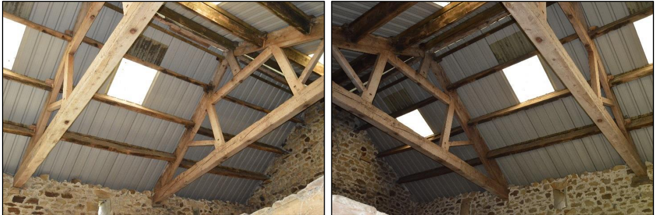
PLI 7: View of timber purlins to the roof of the main core of the barn. It was noted that additional timbers have been installed to the top of the timber purlins to the roof of the main core of the barn. The exact purpose of this could not be confirmed at the time of inspection. It may be that they were installed to facilitate the installation of the sheet roof covering as opposed to any sort of strengthening works, however further investigations are recommended to confirm this.
