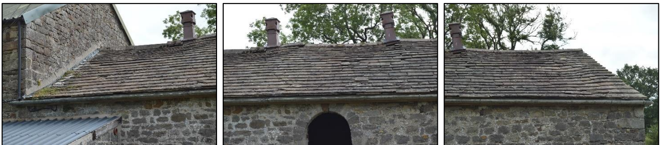
PL19: View of the stone flag roof covering to the west roof slope of the south addition.
