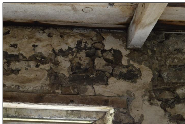
PL69: Poorly consolidated masonry was noted over the head of the east window to the south gable of the south addition. Making good is recommended to consolidate the masonry.
