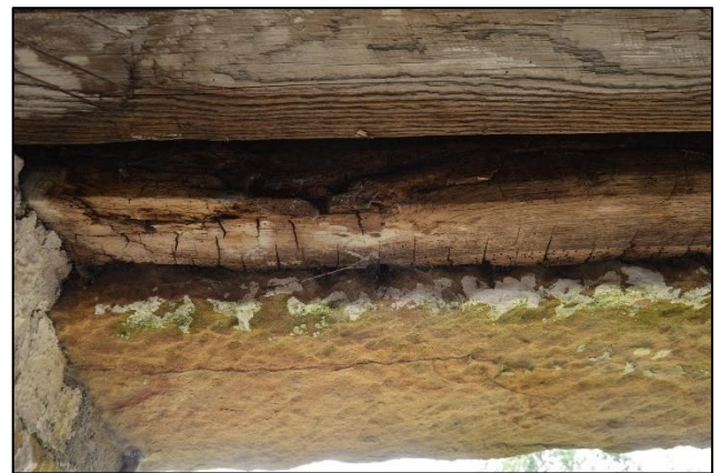
PL54: Decay was noted to the timber safe lintel located over the west elevation personnel door to the south addition. Replacement is recommended.
