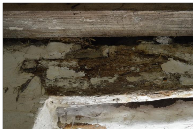
PL58: Minor decay and evidence of wood-boring insect attack was noted, i.e. insect flight holes, to the timber lintel over the ground floor window to the north end of the east elevation of the south addition, adjacent to the west lean-to structure. It is recommended that the lintel is replaced.
