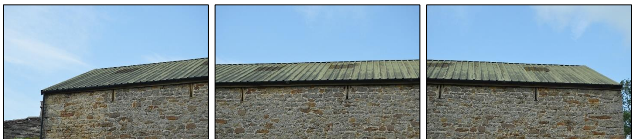
PL15: View of the profiled metal sheet roof covering to the east roof slope of the main core of the barn.
