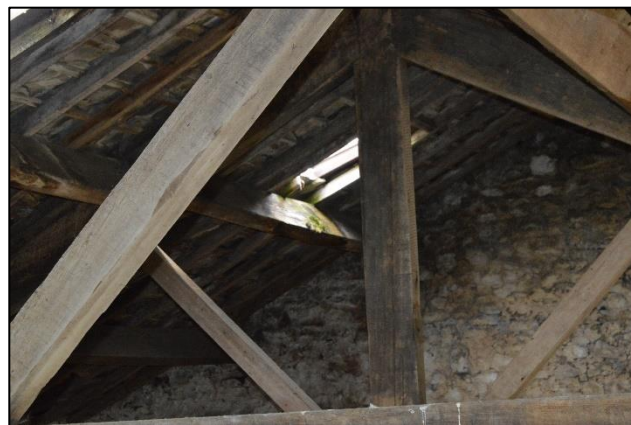
PL22: Staining noted to the timber purlins located beneath the roof lights to the east roof slope of the south addition, suggesting potential water ingress at these locations. This has led to some decay of the timbers below the roof light locations and it is recommended that these areas are closely inspected on erection of a safe working platform to confirm condition and full extent of decay.
