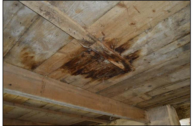
PL86: View of areas of decayed timber floor boards present to the suspended timber floor to the northern half of the south hayloft.
