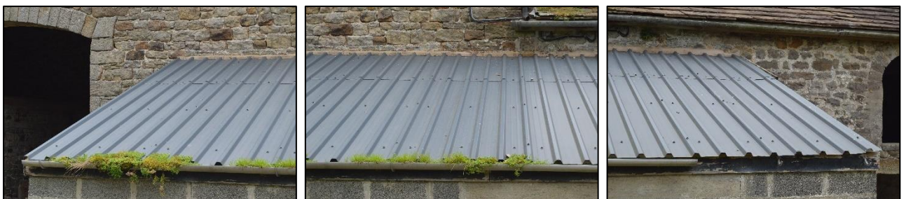
PL08: View of the profiled sheet roof covering to the west lean-to structure.
