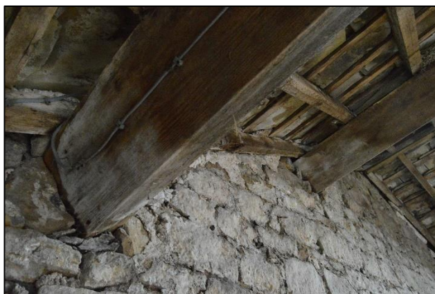
PL24: View of staining noted to the roof timbers of the south addition where the timbers are built into the stone wall fabric.
