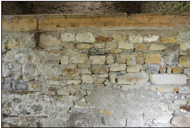
PL74: Areas of perished mortar were widely noted throughout the building and repointing using a lime based mortar is recommended. Any larger voids should be packed with mortar and gallet stones and then repointed.
