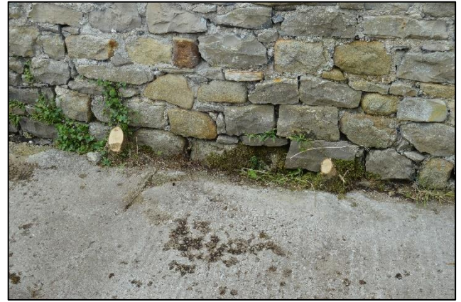
PL47: A number of tree / sapling stumps were noted to the wall base of the east elevation. It is recommended that stumps are fully removed as well as the underlying root matrices.
