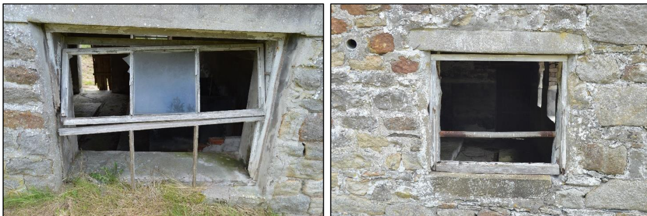
PL92: Examples of windows present to the building at the time of inspection.
