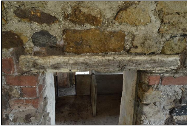
PL73: Decay and evidence of wood-boring insect attack i.e. flight holes, noted to the timber lintels over the wall opening to the north side of the main core of the barn. Replacement of the lintels is recommended.
