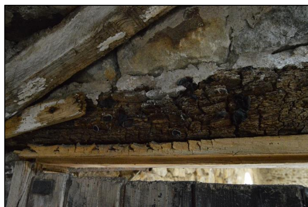
PL70: Decay and fungal growth were noted to the south timber lintel over the internal door opening between the main core of the barn and the hayloft to the south addition. Replacement is recommended.
