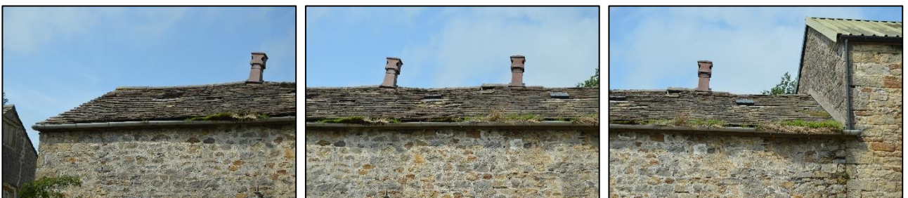
PL20: View of the stone flag roof covering to the east roof slope of the south addition.
