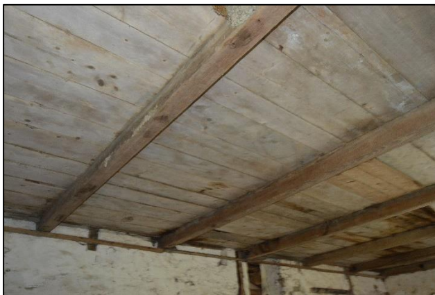
PL83: View of the suspended timber floor structure to the southern half of the south hayloft.
