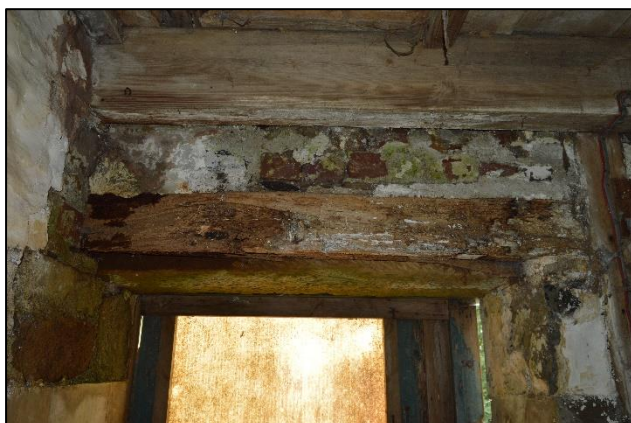
PL57: Decay was noted to the internal timber safe lintel over the external doorway to the north end of the east elevation of the south addition. It is recommended that the lintel is replaced.
