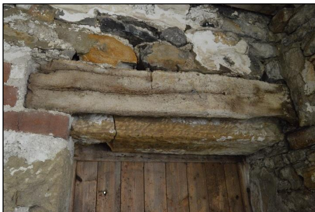
PL50: The stone lintel to the doorway at the south end of the east elevation was cracked and replacement will be required. The internal timber safe lintel was also noted as being slender in profile and was decayed. It also contained evidence of wood-boring insect attack and replacement of the timber lintel is also required.
