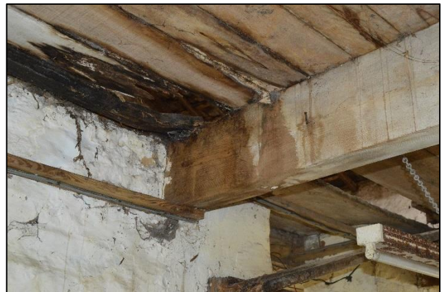
PL87: View of staining noted to isolated floor joists to the northern half of the south hay loft.
