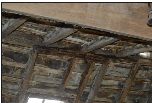
PL23: View of decay and repairs undertaken the ridge beam of the roof to the south addition. It is recommended that these areas are closely inspected on erection of a safe working platform to confirm condition.
