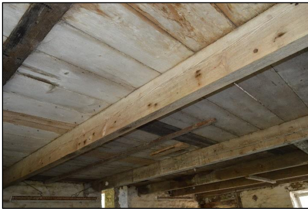
PL85: View of the suspended timber floor to the north half of the southern hay loft.
