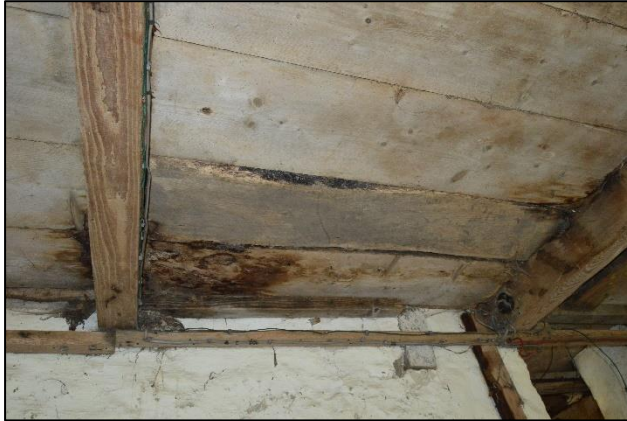
PL84: View of areas of decayed timber floor boards present to the suspended timber floor to the southern half of the south hayloft, likely caused by past water ingress from the roofing above.
