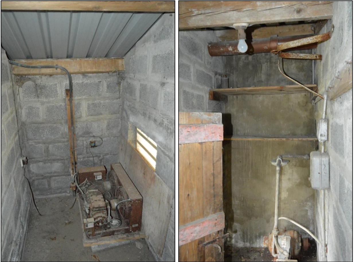
PL64: Internal views within the north unit of the west lean-to.
