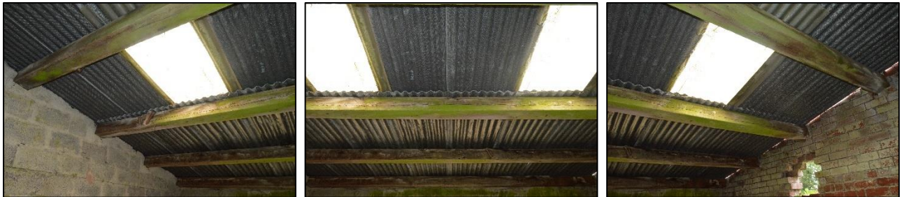
PL06: View of the timber roof structure to the roof of the north lean-to structure.
