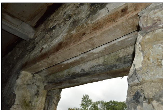
PL51: Minimal end bearings were noted to the internal timber safe lintels over the east opening to the ground floor of the south gable end of the south addition. Evidence of wood-boring insect attack was also noted, i.e. insect flight holes. It is recommended that the lintels are replaced with new lintels with a minimum end bearing of 150mm – 200mm.
