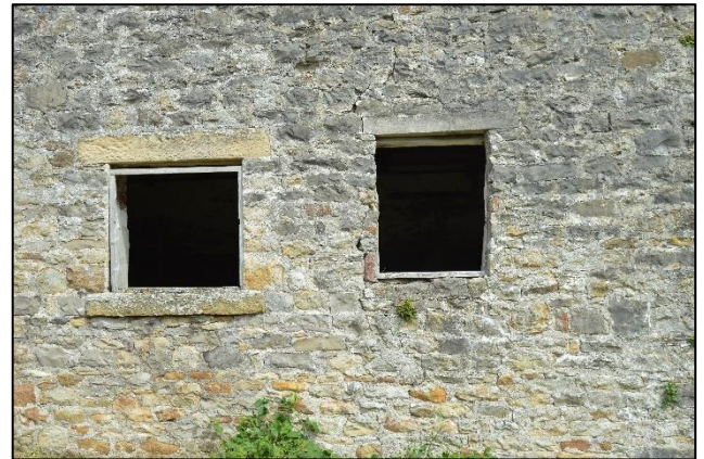
PL48: Isolated vertical cracking was noted over the east window opening to the south gable end of the south addition. The cracking was deemed to be slight (between 1mm and 5mm) to moderate (between 5mm and 15mm). A fall was also noted to the window head at this location. It is recommended that bed joint reinforcement is installed where coursing will allow i.e. stainless steel helical bars and the affected area then repointed using a lime mortar. This should then be monitored for any further evidence / re-occurrence of cracking or movement. Should any further movement / cracking occur then this will require assessment by a Structural Engineer and structural repairs undertaken as required.
