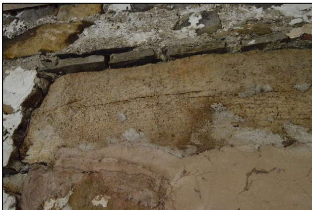
PL55: Evidence of wood-boring insect attack was noted to the internal timber safe lintel over the blocked-up door opening to the west side of the south addition, i.e. insect flight holes. It is recommended that the timber lintel is replaced.
