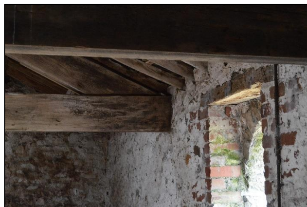
PL24: View of staining noted to the roof timbers of the south addition where the timbers are built into the stone wall fabric.
