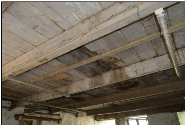
PL87: View of staining noted to isolated floor joists to the northern half of the south hay loft.
