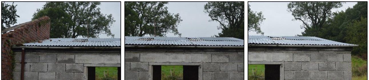
PL05: View of the metal profiled sheet roof covering to the north lean-to structure.
