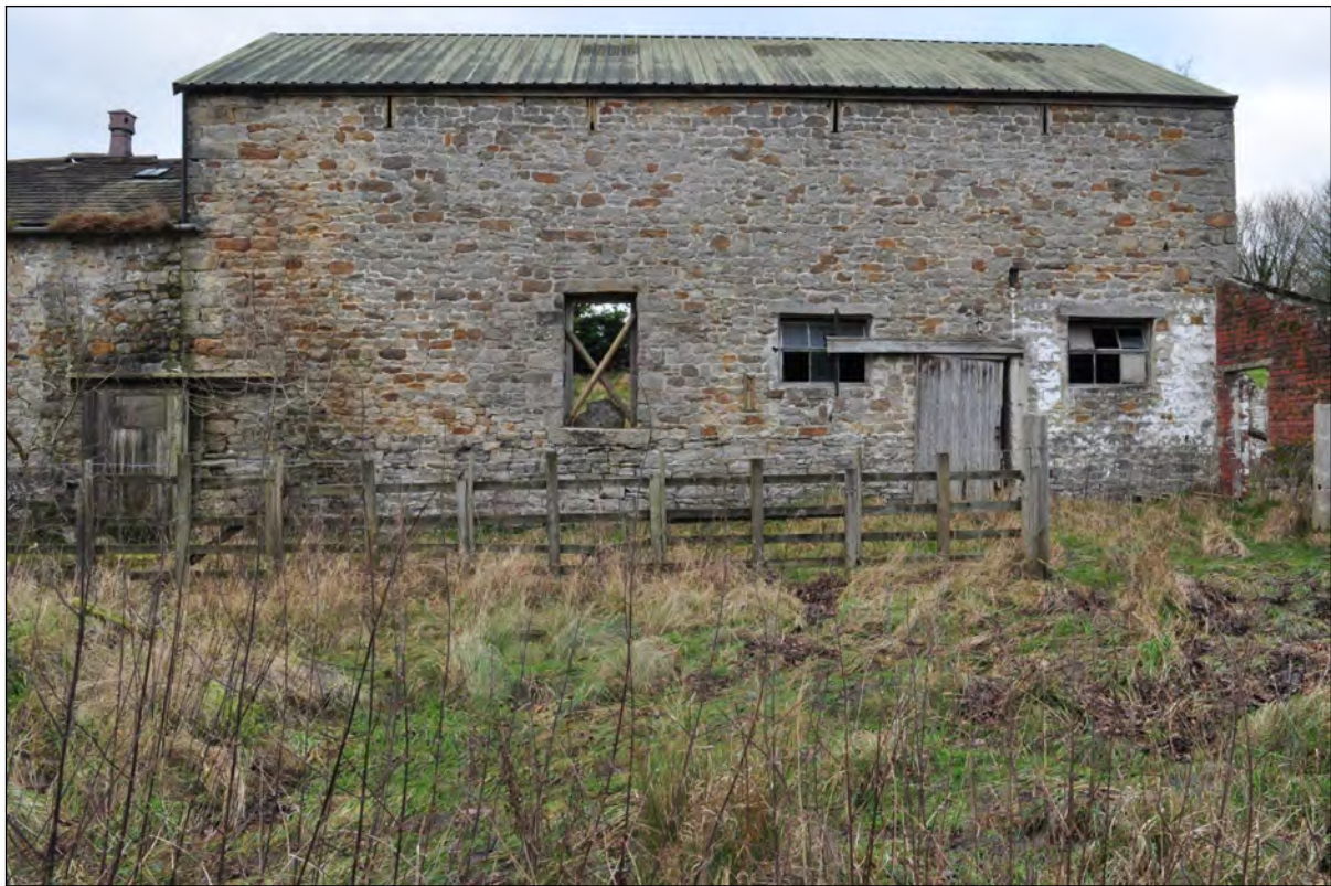
Photo 5: Building A: south-east elevation.
