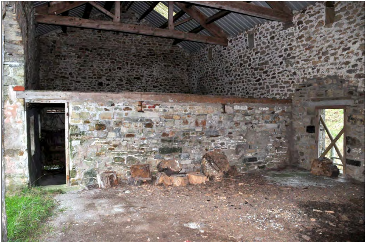
Photo 7: Building A interior: 20th century cross-wall enclosing shippon in north-east end
