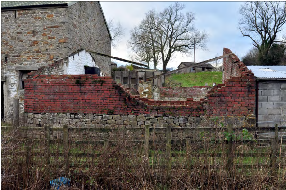
Photo 11: Building C: south-east elevation
