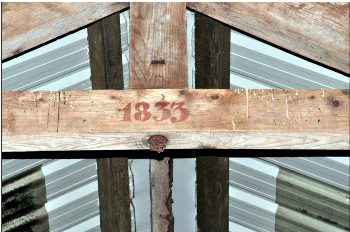
Photo 8: Building A: dated roof timber
