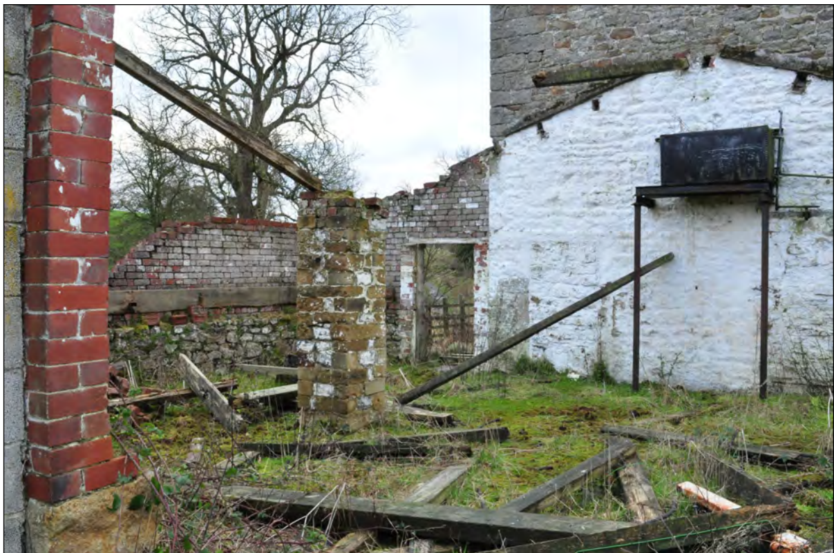
Photo 12: Building C: interior, looking south
