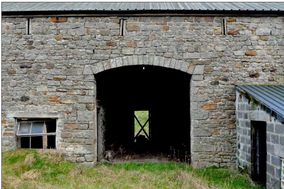
Photo 4: Arched entrance and ventilation slits in north-west elevation of building A
