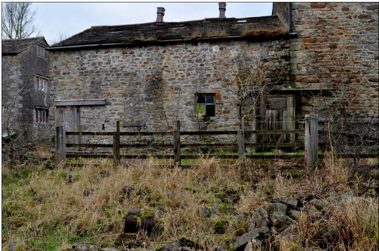
Photo 10: Building B: south-east elevation
