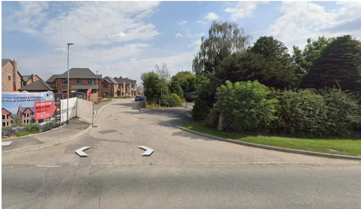
Figure 2: Street View image of the access to the site (Google Earth)
