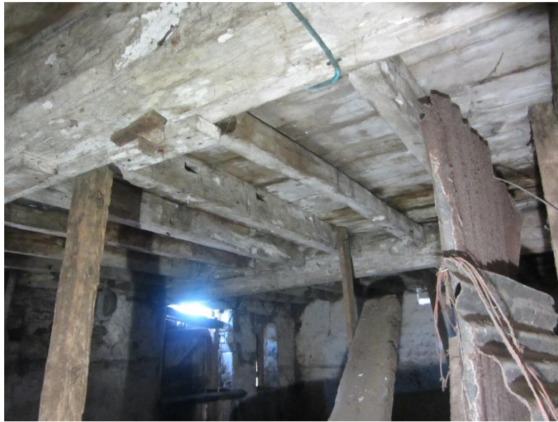
Photo 7 – Timber loft floor (front)
