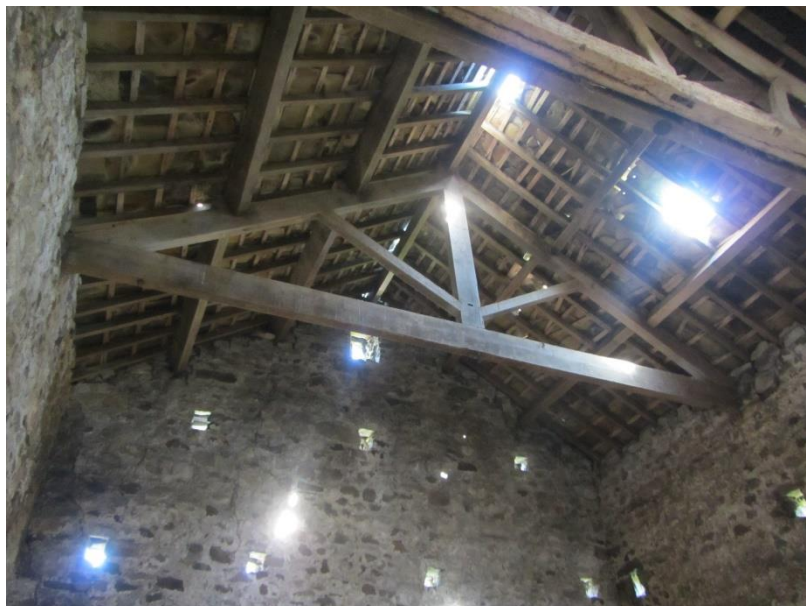
Photo 4 – Internal view, looking north west
