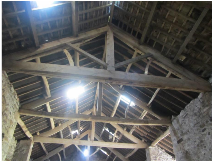
Photo 5 – Internal view – looking south east
