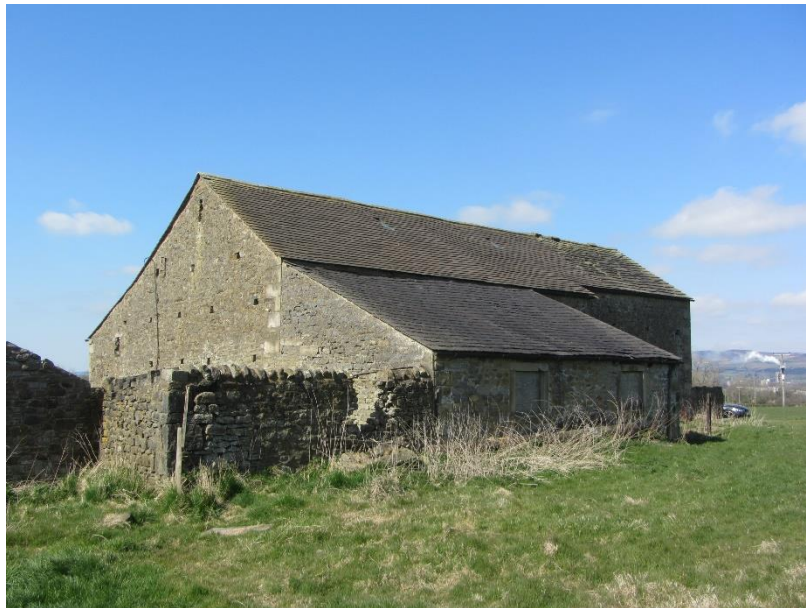
Photo 3 – View of barn from east
