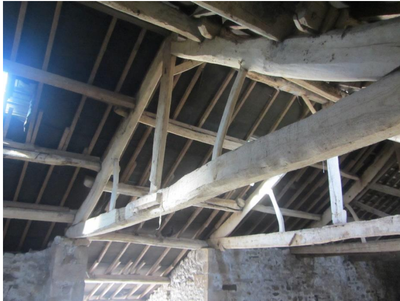
Photo 11 – Oak roof trusses
