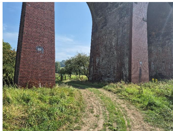
Photo 18: Viaduct pillars each side of the access track
