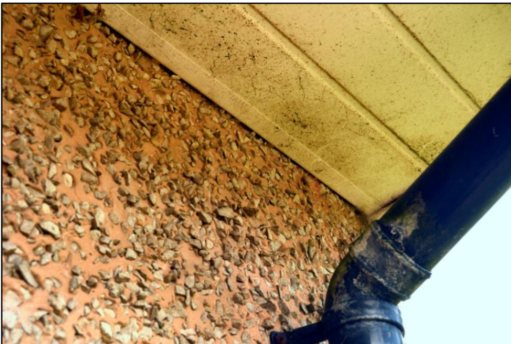
Close up image showing sealed upvc soffit on pebble dashed rendered walls of bungalow, June 2026.
