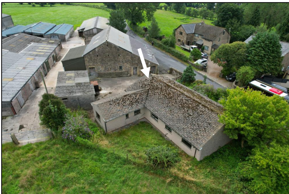
Oblique aerial taken in 2025 showing bungalow building (white arrow).
