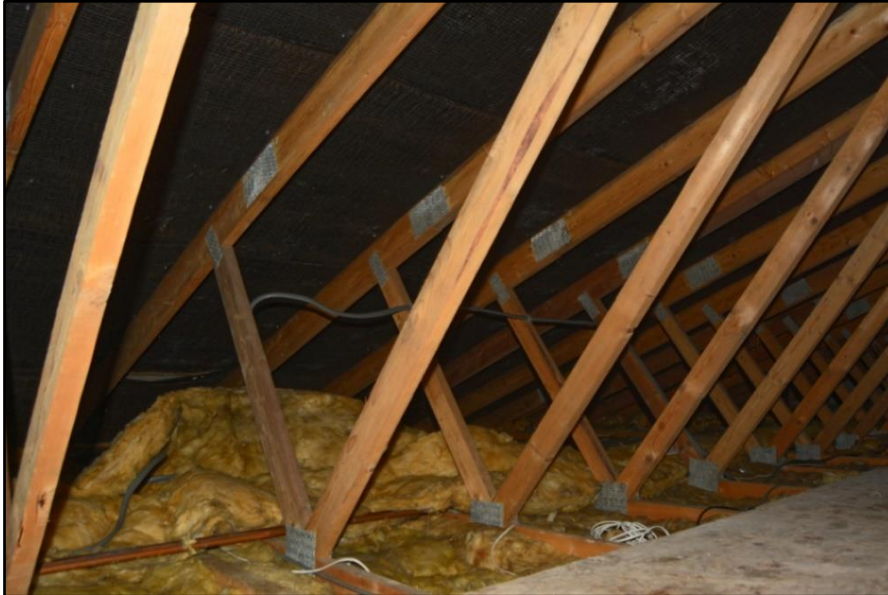
Image showing bungalow roof void, cluttered with roof trusses.
