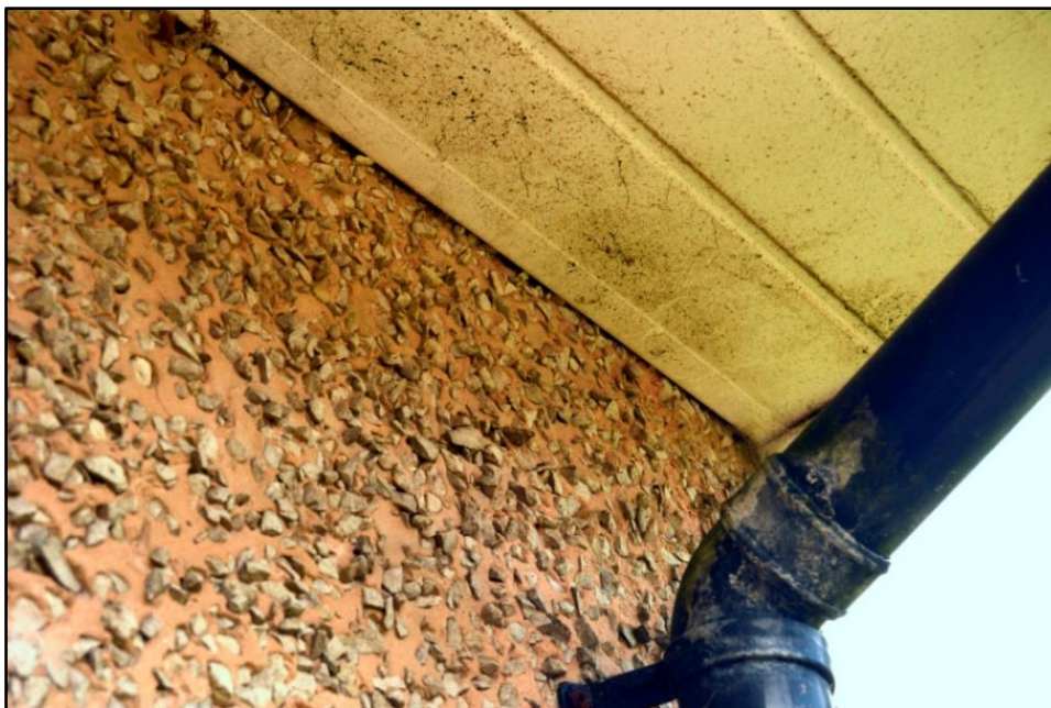
Close up image showing sealed upvc soffit on pebble dashed rendered walls of bungalow
