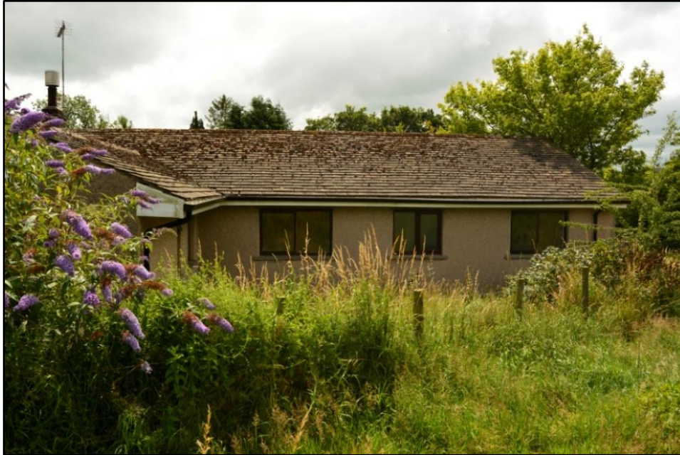
Image showing north (rear) elevation of bungalow (B1)
