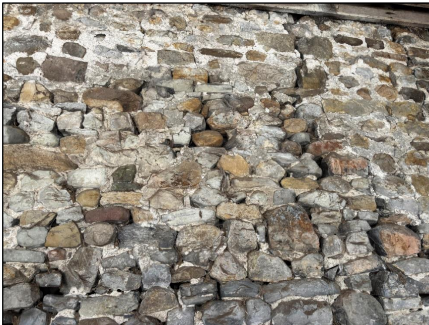
Example of wall cavities (PRFs) in barn
