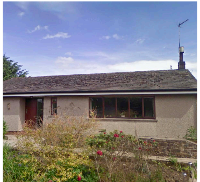
View of existing bungalow from the road
