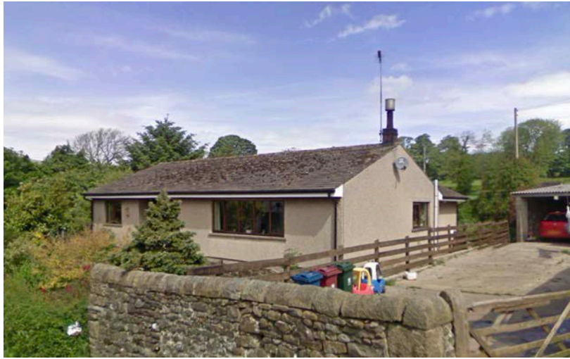
Picture of the front of the existing dwelling from the road.
