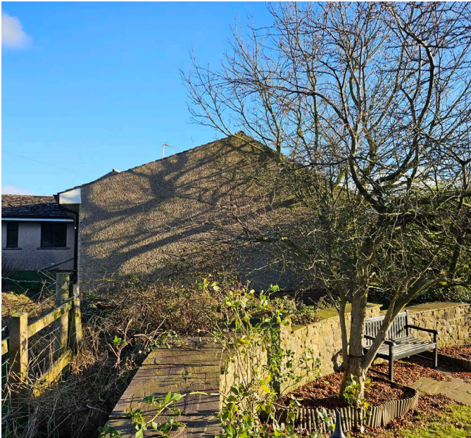
West elevation of the existing bungalow looking from the war memorial
