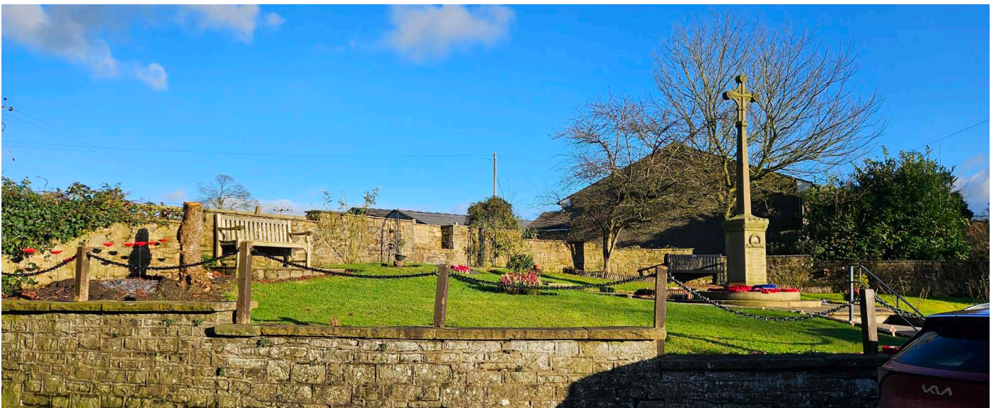
View of the west elevation of the bungalow when standing in front of the war memorial
