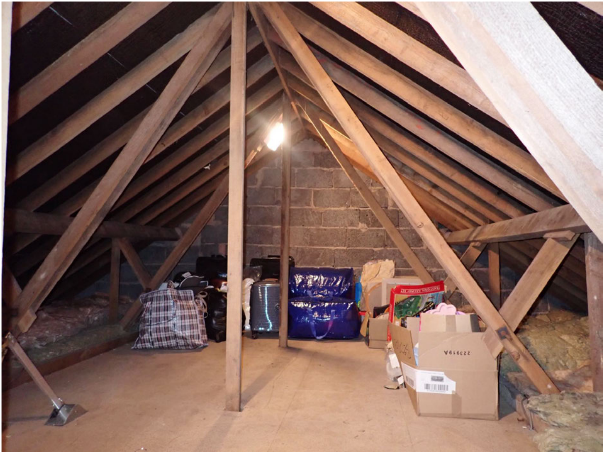
3.2a – The roof void.
