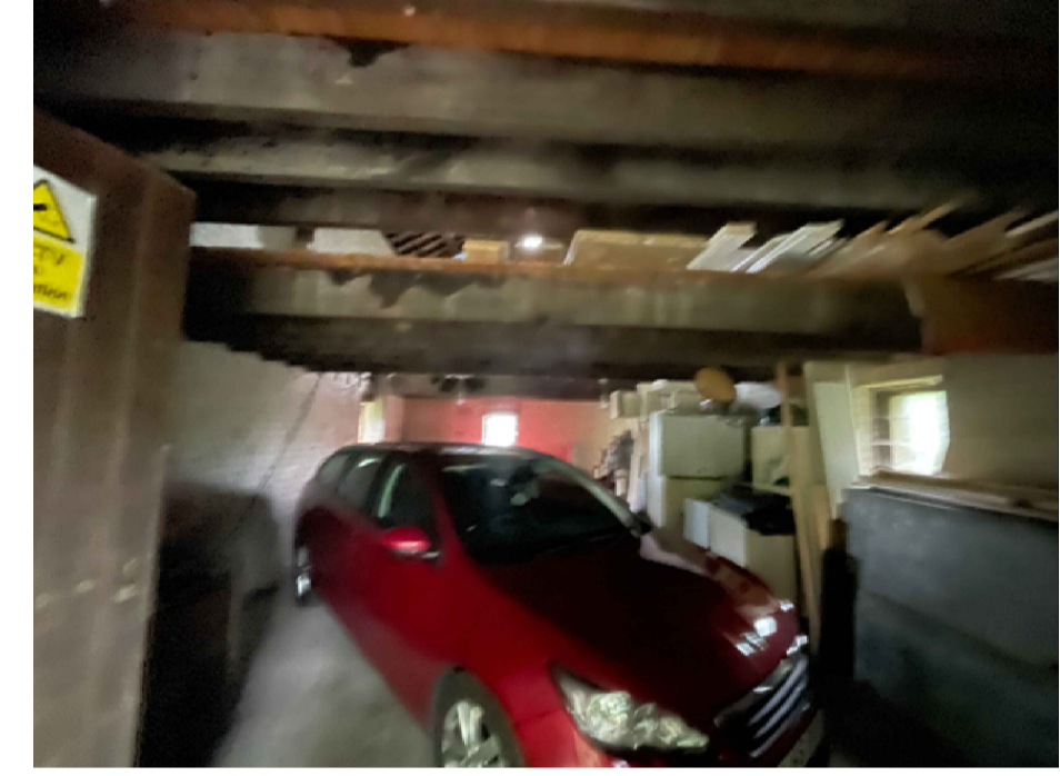
INTERNAL IMAGE IN GARAGE - GROUND FLOOR
