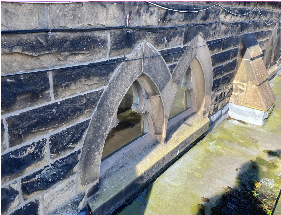
Photo 4: Showing existing stone window reveal with very low upstand beneath which is resulting in water ingress (roof 1)
