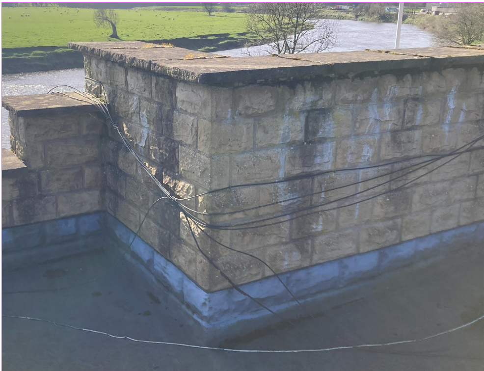
Photo 2: Showing existing surface faced upstanding which is resulting in water ingress (roof 2)
