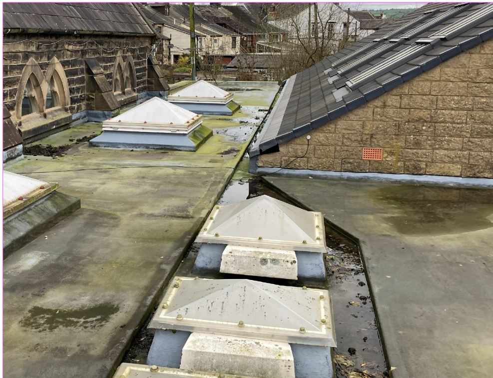
Photo 1: Showing existing rooflights and liquid plastic flat roof covering (roof 2)
