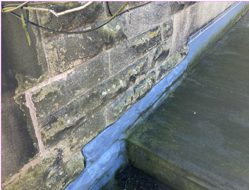
Photo 5: Showing existing surface faced upstand which is resulting in water ingress (roof 1)
