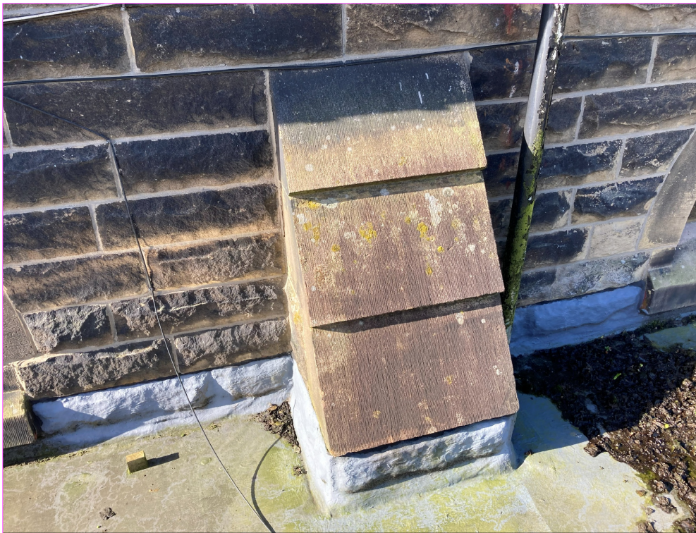
Photo 3: Showing existing surface faced upstand which is resulting in water ingress (roof 2)
