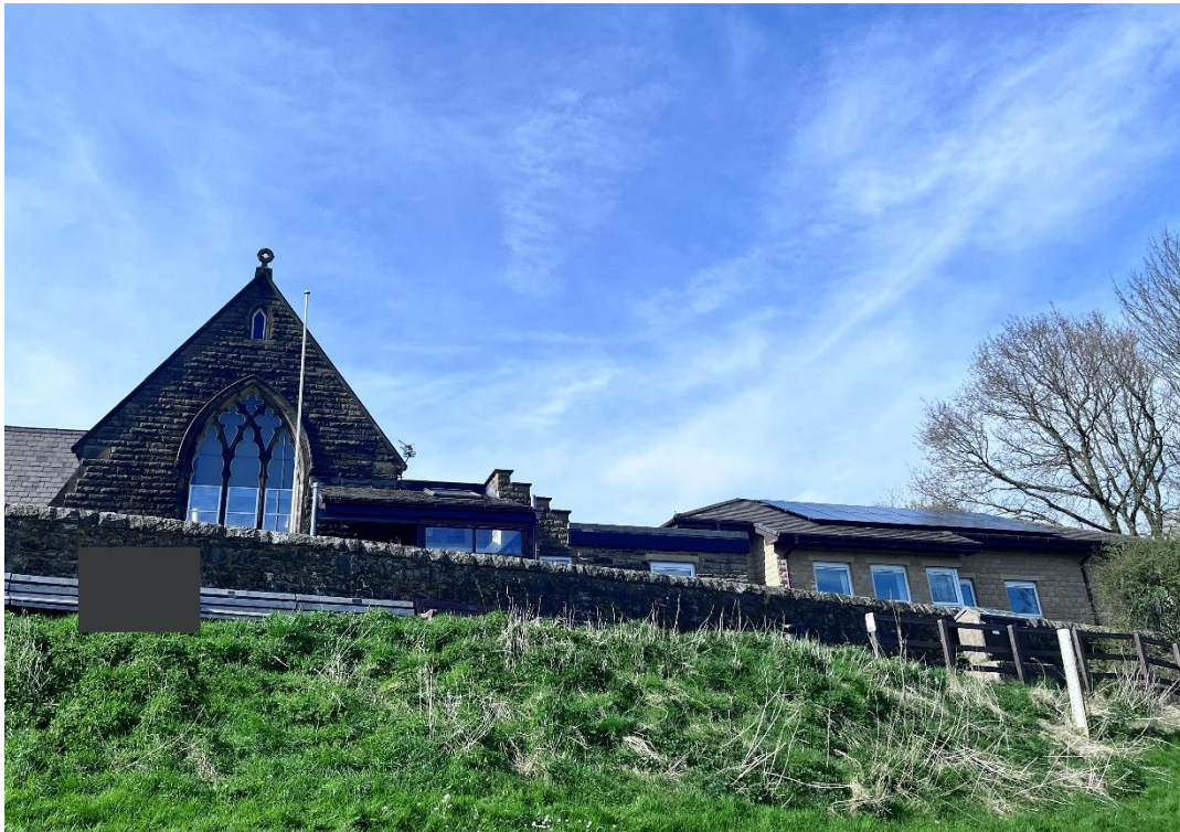
Figure 4. Photograph of St Wilfrid's Primary School taken from the riverside [Source: C+A]
