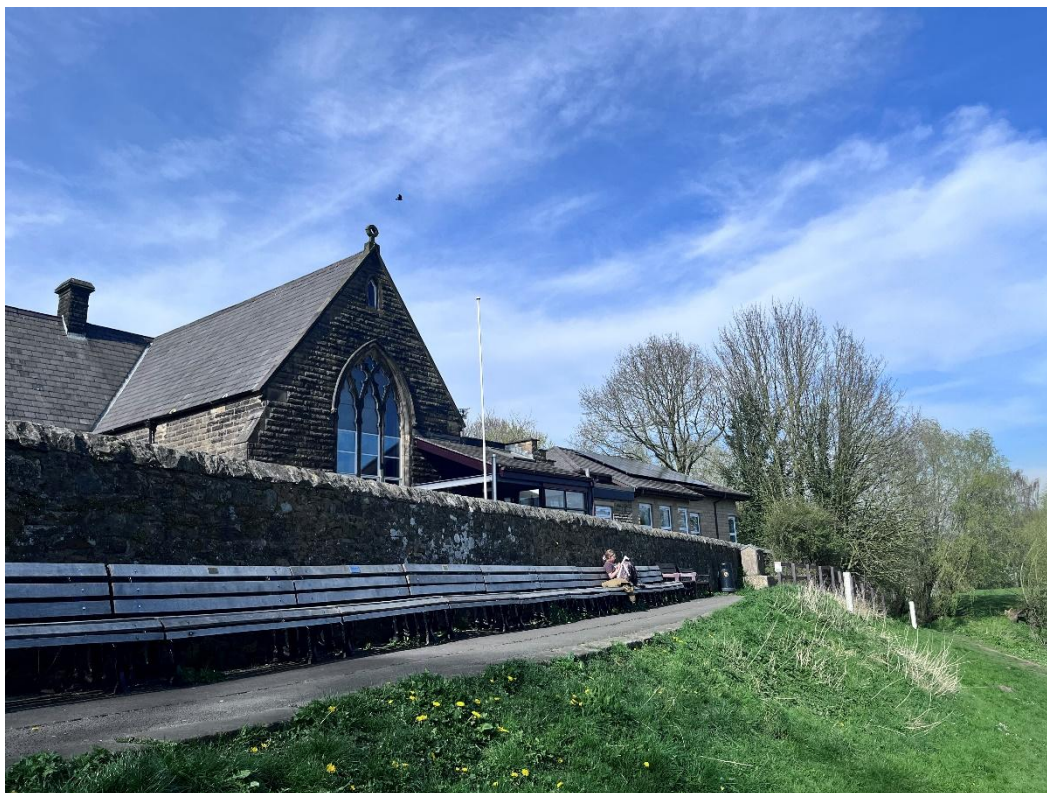
Figure 3. Side elevation of St Wilfrid's Primary School taken from the riverside [Source: C+A]
