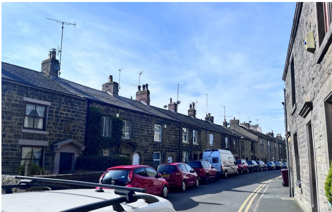
Figure 7. Photograph of 8-15 Church Street [Source: C+A]
