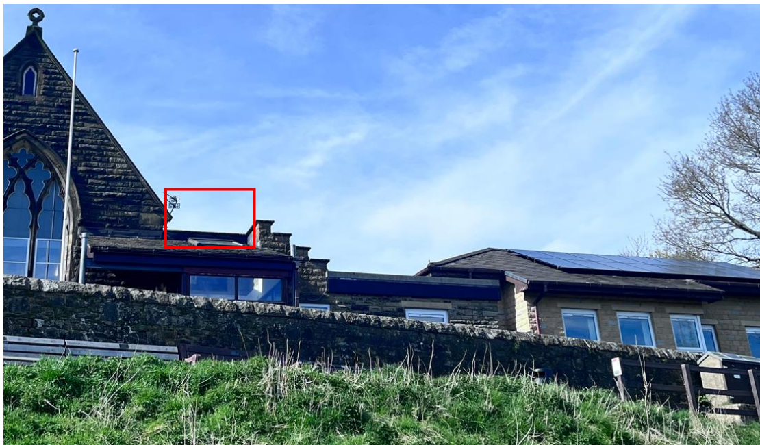
Figure 8. Photograph of proposed location of air source heat pump on the south elevation of the school
