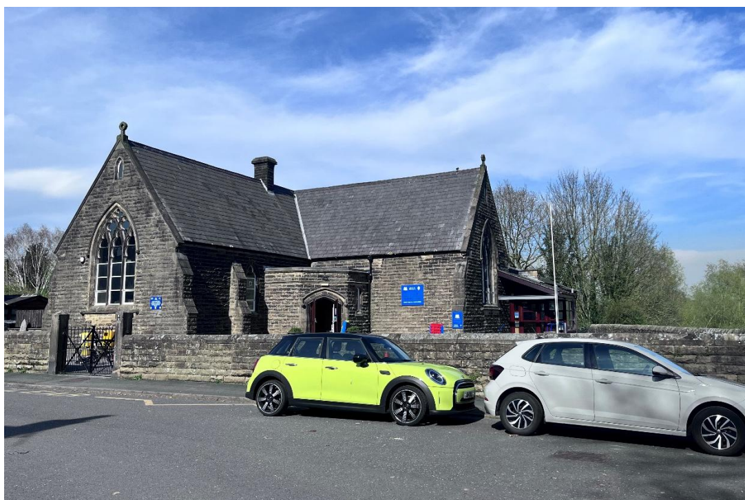
Figure 4. Front elevation of St Wilfrid's Primary School taken from the southwest [Source: C+A]
