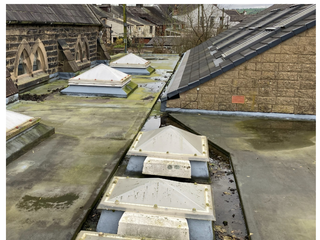
Photo 1: Showing existing rooflights and liquid plastic flat roof covering (roof 2)
