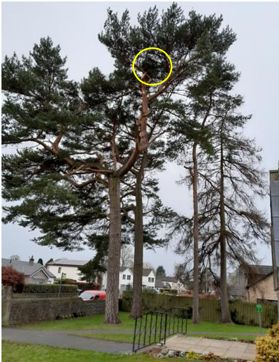
The trees and wind damage (looking west)
