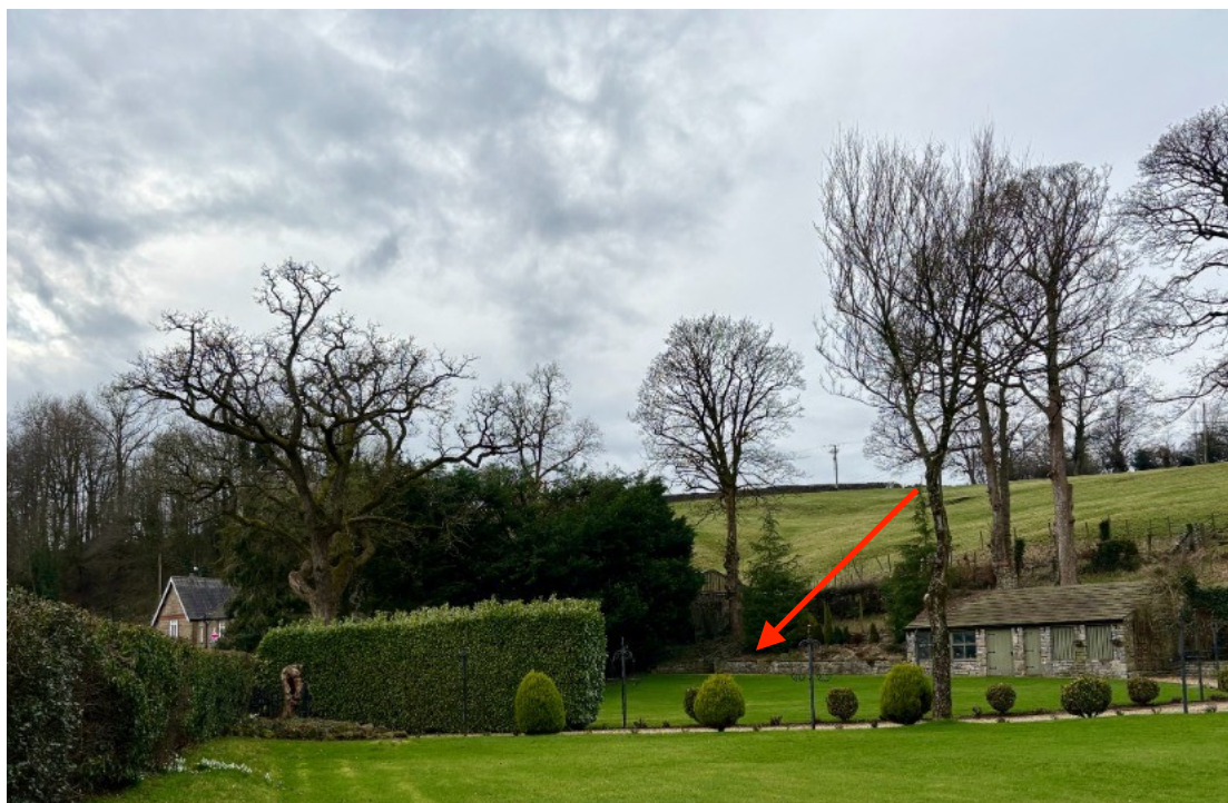
Photo 1: photo of the site
