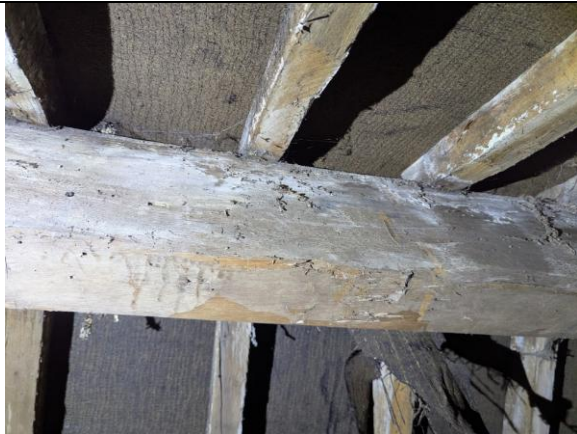
Photograph 21: Clean and clear beams above dropping pile
