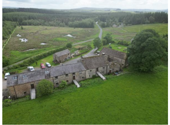
Photograph 8: Aerial view, looking south
