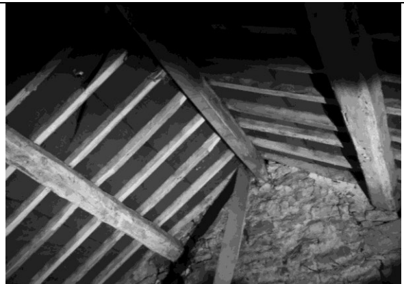
Photograph 24: Example infrared image from within the roof void
