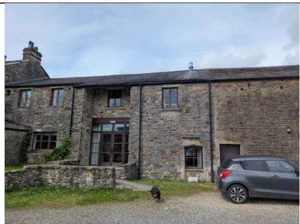
Photograph 6: Southern elevation of barn conversion
