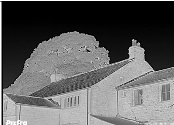
Photograph 23: Example of thermal image of southern elevation of property
