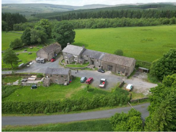
Photograph 7: Aerial view, looking north
