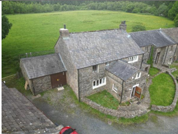
Photograph 9: Aerial view of southern elevation
