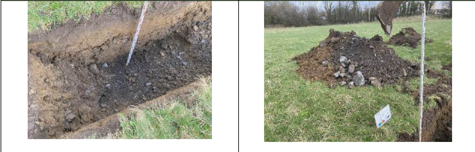
P27: Trial Pit 10 P28: Trial Pit 10 Arisings
