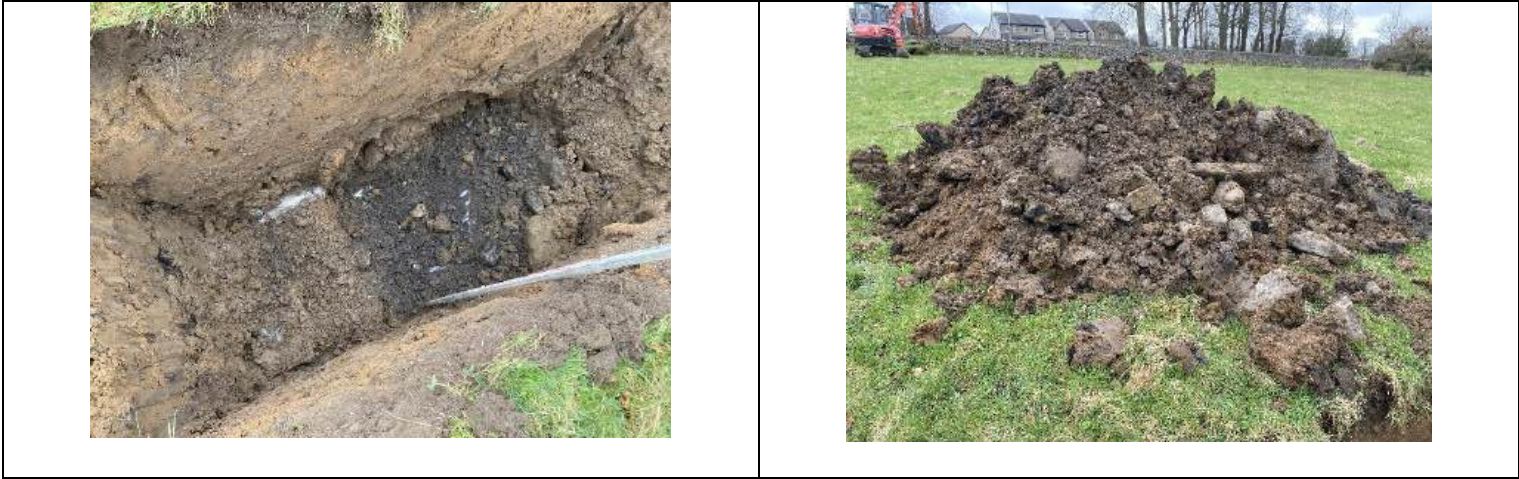
P13: Trial Pit 5 P14: Trial Pit 5 Arisings
