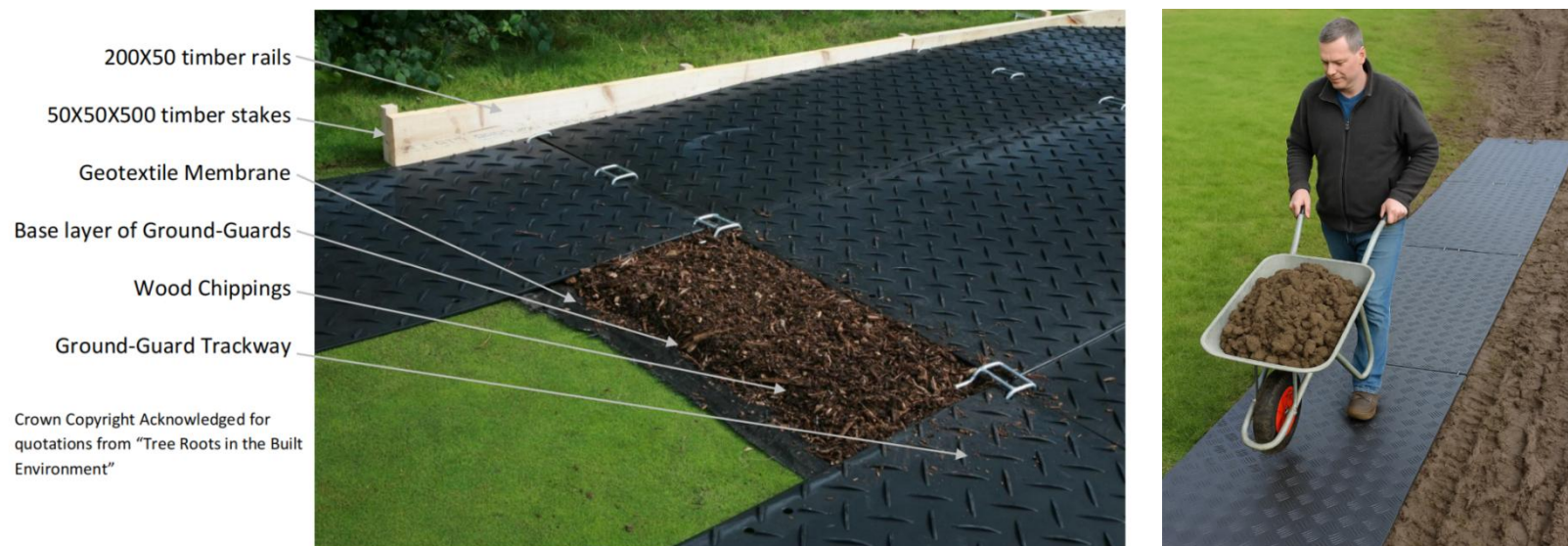
Figure 2: Example of suitable ground protection
