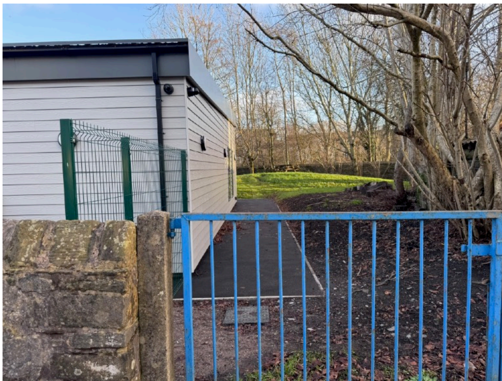
Photo 5: the end of the footpath will be on the back street of Woone Lane at the side of the new nursery building
