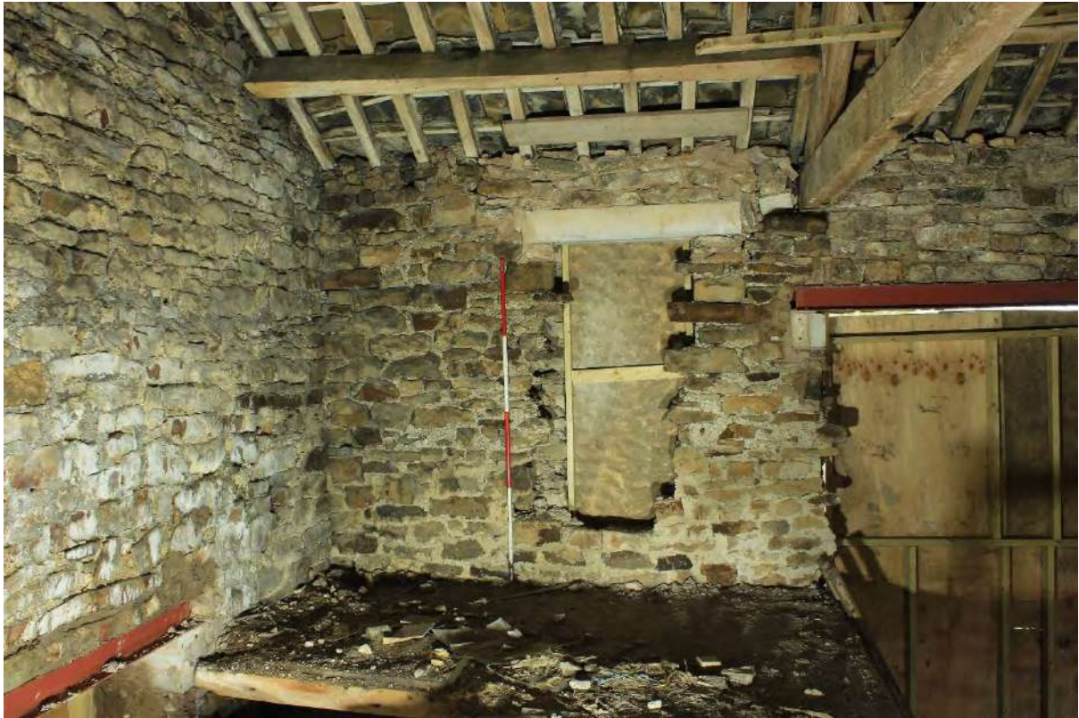
Plate 33 West and north walls of the hay loft over the byre with pitching loft opening (centre) and north wagon doorway (right), looking north
