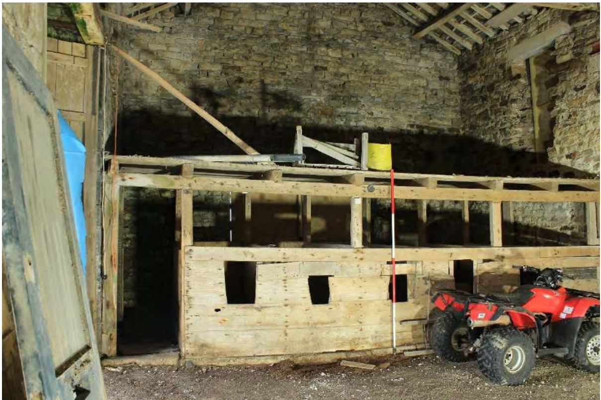
Plate 30 20 th century animal stalls in Bay 1 at the west end of Building A
