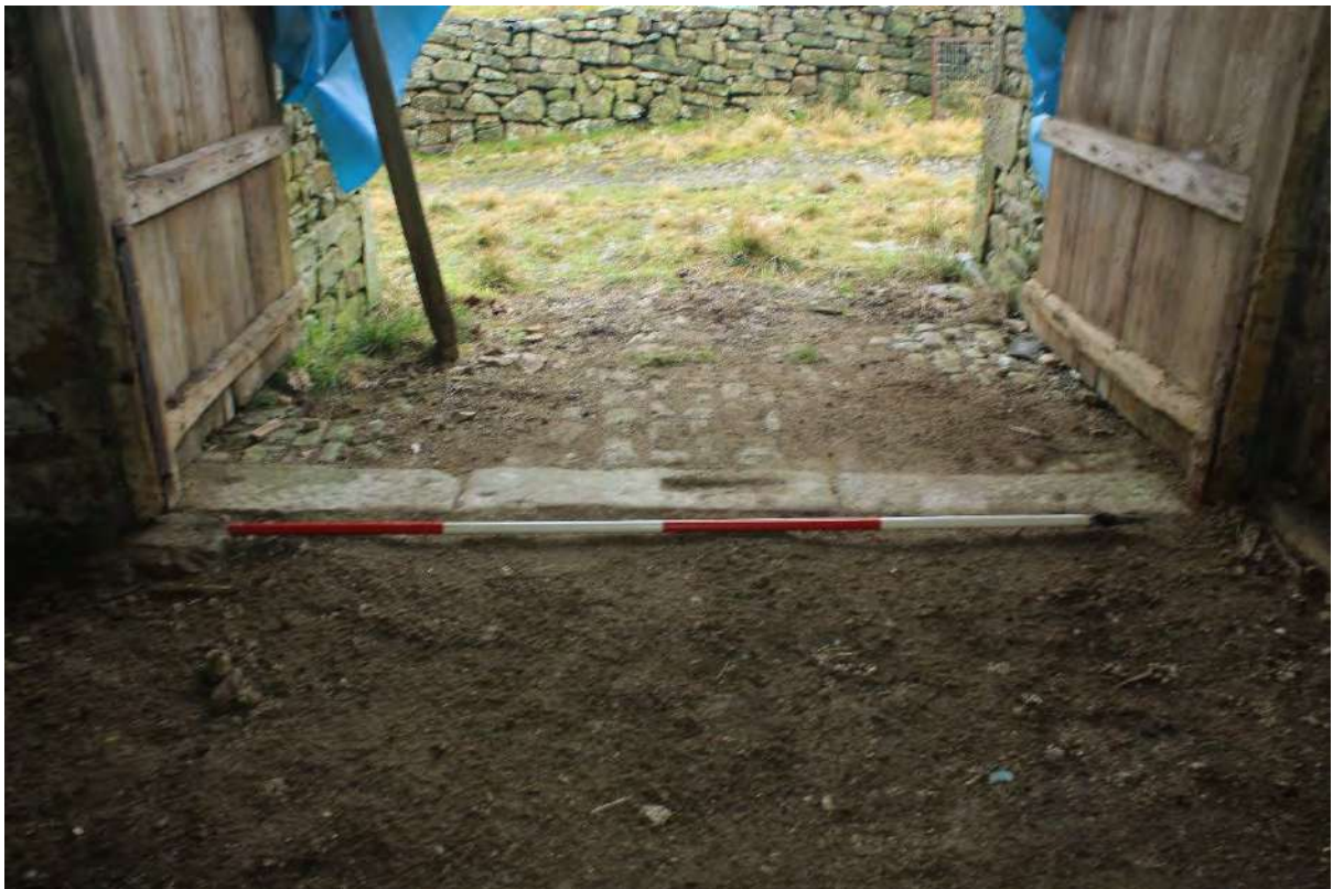
Plate 26 Stone threshold of the south cart-entrance
