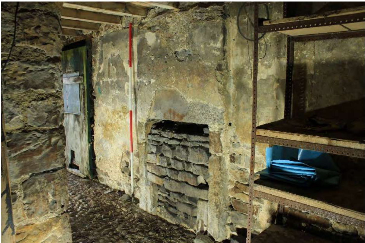
Plate 32a Blocked fireplace in the west wall of Bay 4 of Building A
