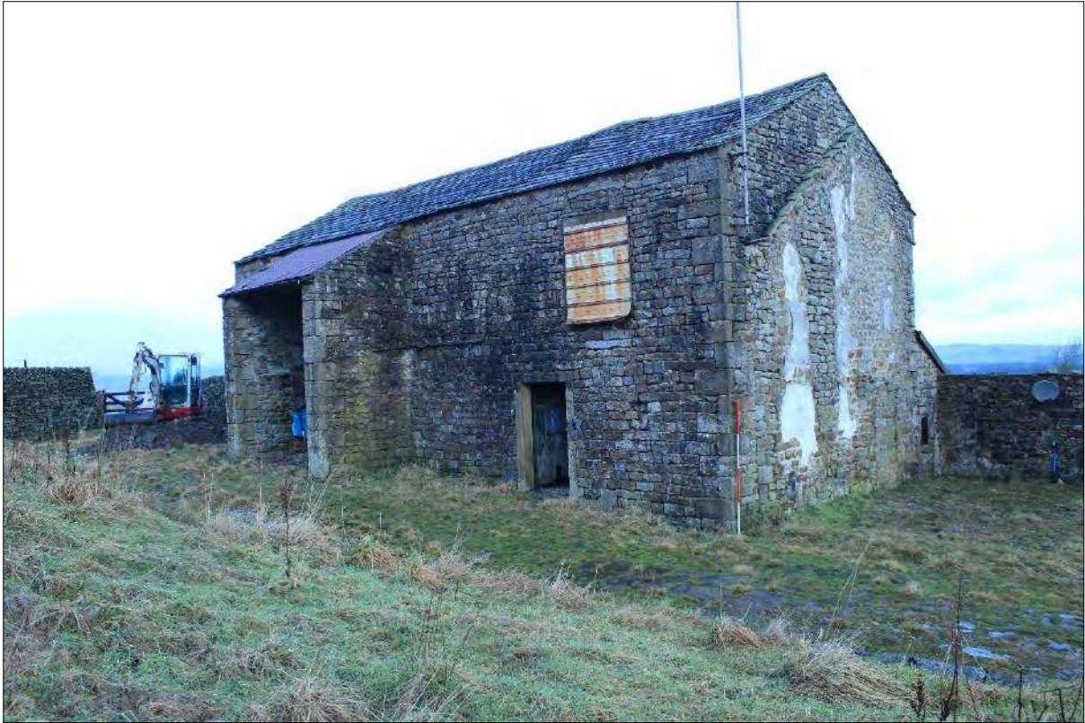
Plate 15 South and east elevations, looking north-west
