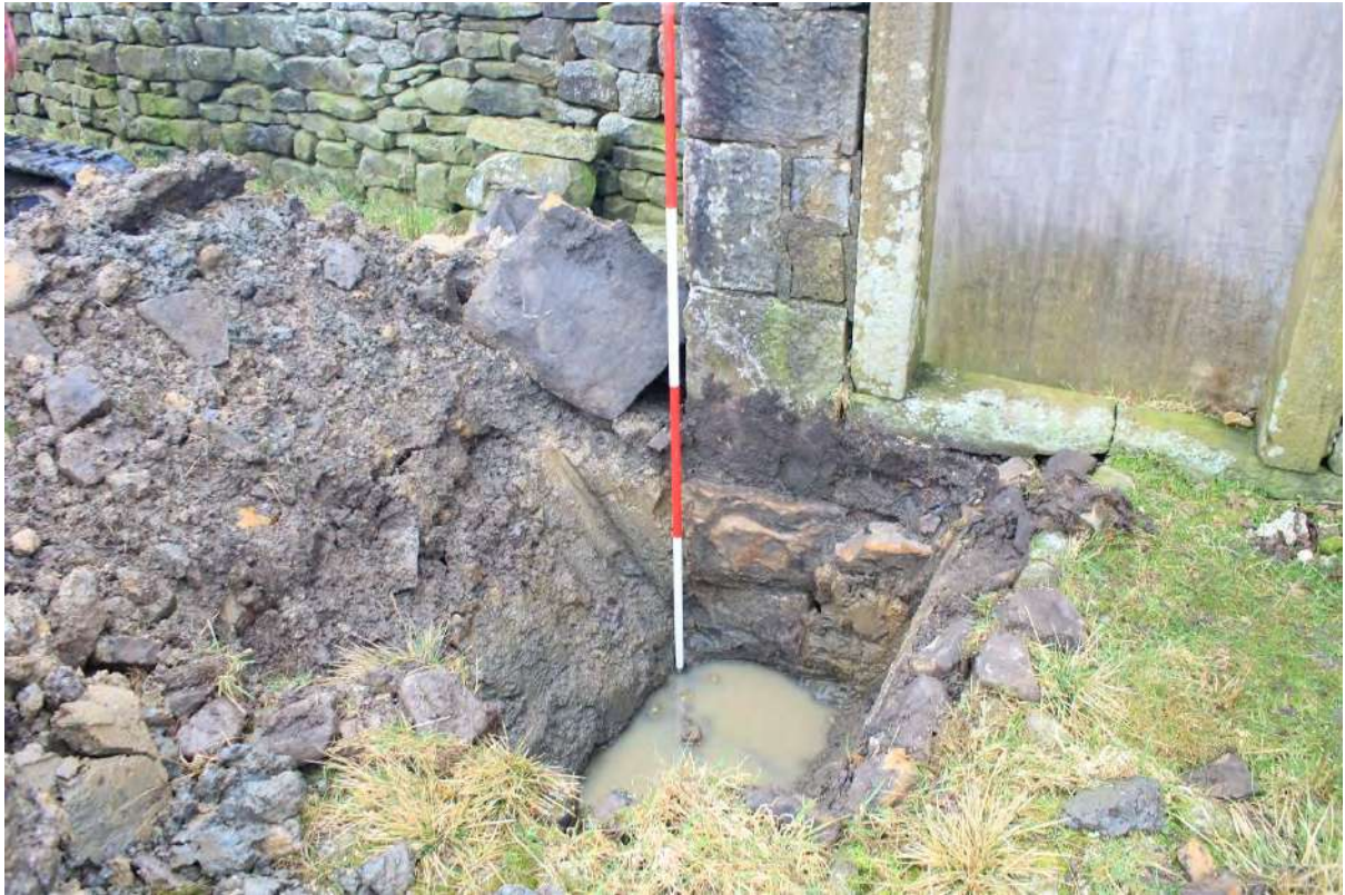
Plate 21 Test pit uncovering the stepped stone foundation of the south wall of Building A at the south-west corner
