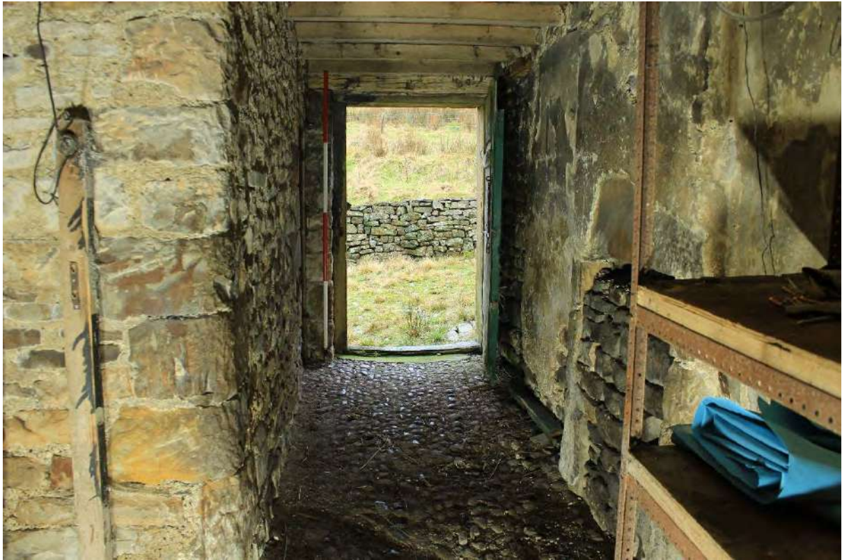
Plate 32 South doorway in Bay 4 of Building A, looking south
