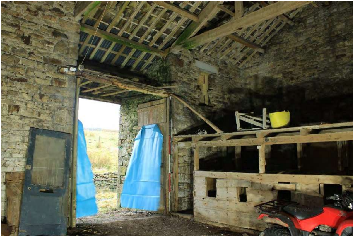
Plate 24 South cart-entrance doorway, looking south-west
