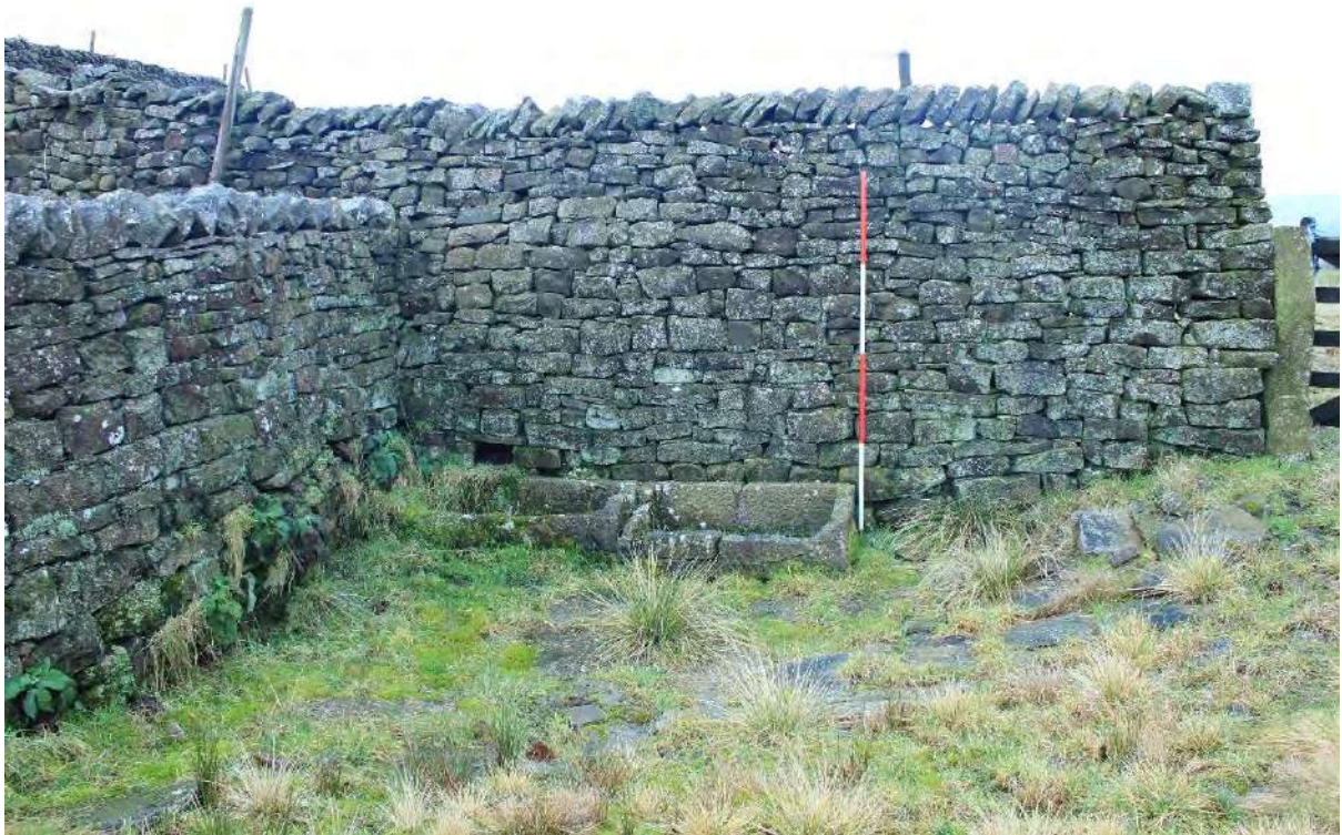
Plate 22 Curtilage walls at the east end of the farmstead range, enclosing the foldyard, with stone trough
