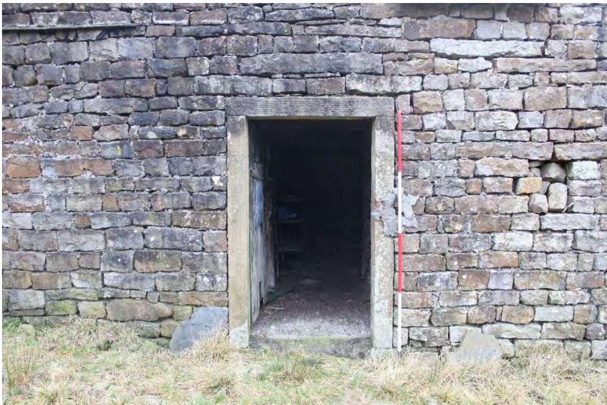
Plate 16 Doorway towards the east end of the south elevation
