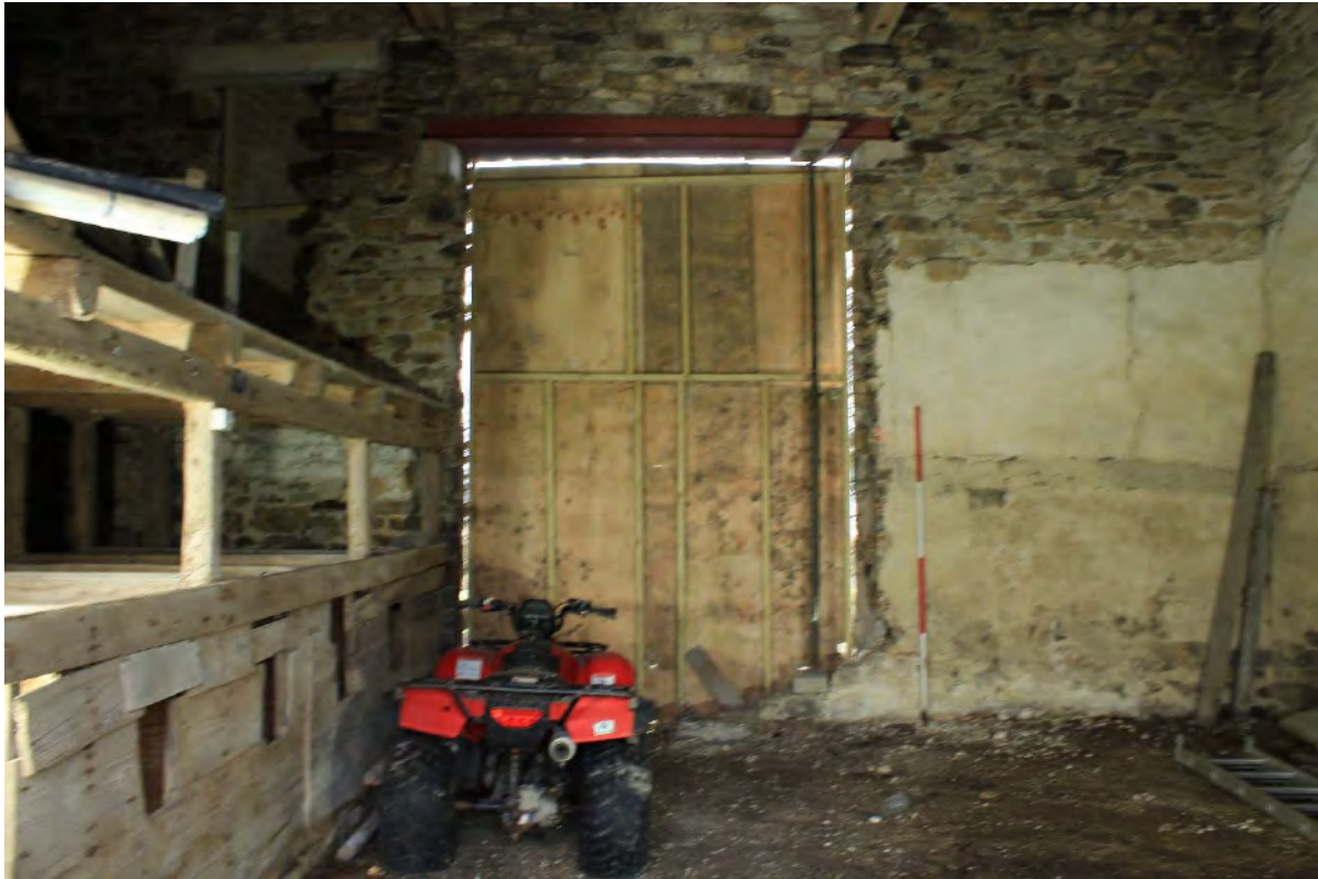
Plate 27 Boarded north wagon doorway of Building A
