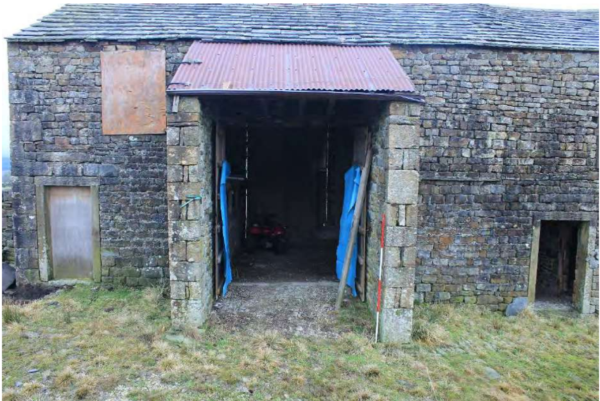
Plate 18 Looking north towards the porched cart-entrance doorway
