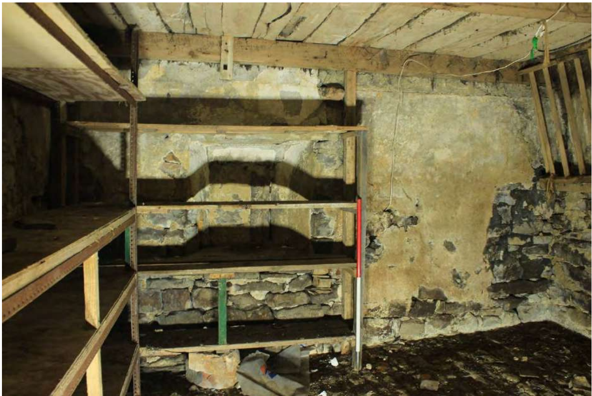
Plate 32e North wall of Bay 4 of Building A
