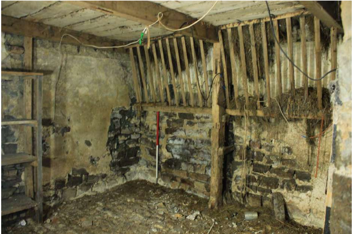
Plate 31 North (left) and east (right) walls in Bay 4 of Building A
