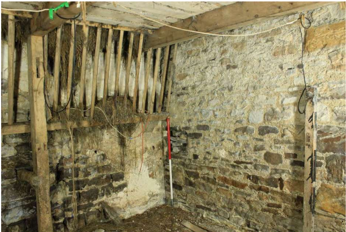
Plate 31a East (left) and dividing walls in Bay 4 of Building A
