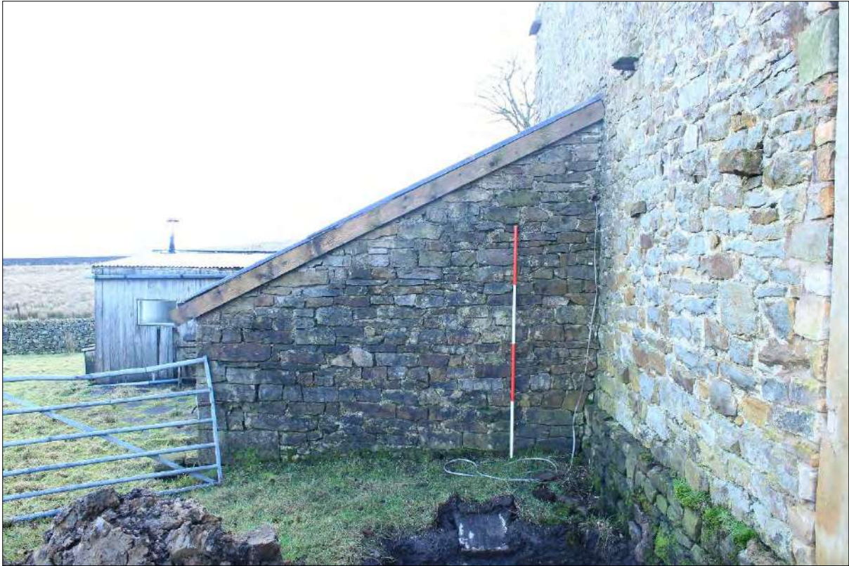
Plate 5 West elevation of the outshot extension
