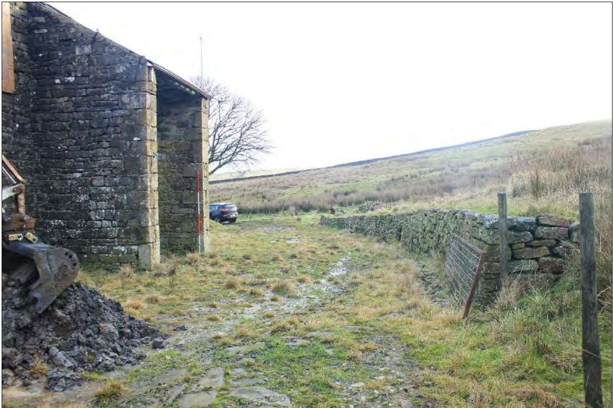
Plate 19 Looking east towards the west wall of the porched cart-entrance
