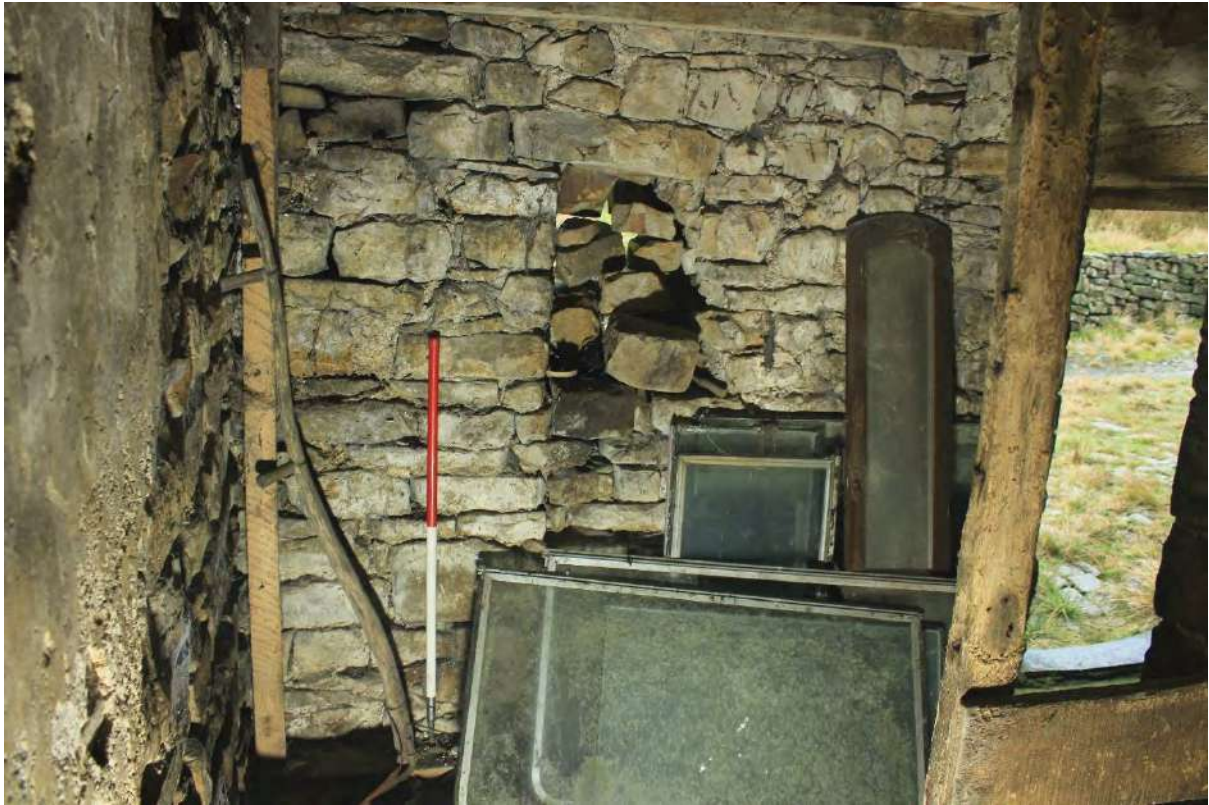
Plate 32f South wall of Bay 4 of Building A
