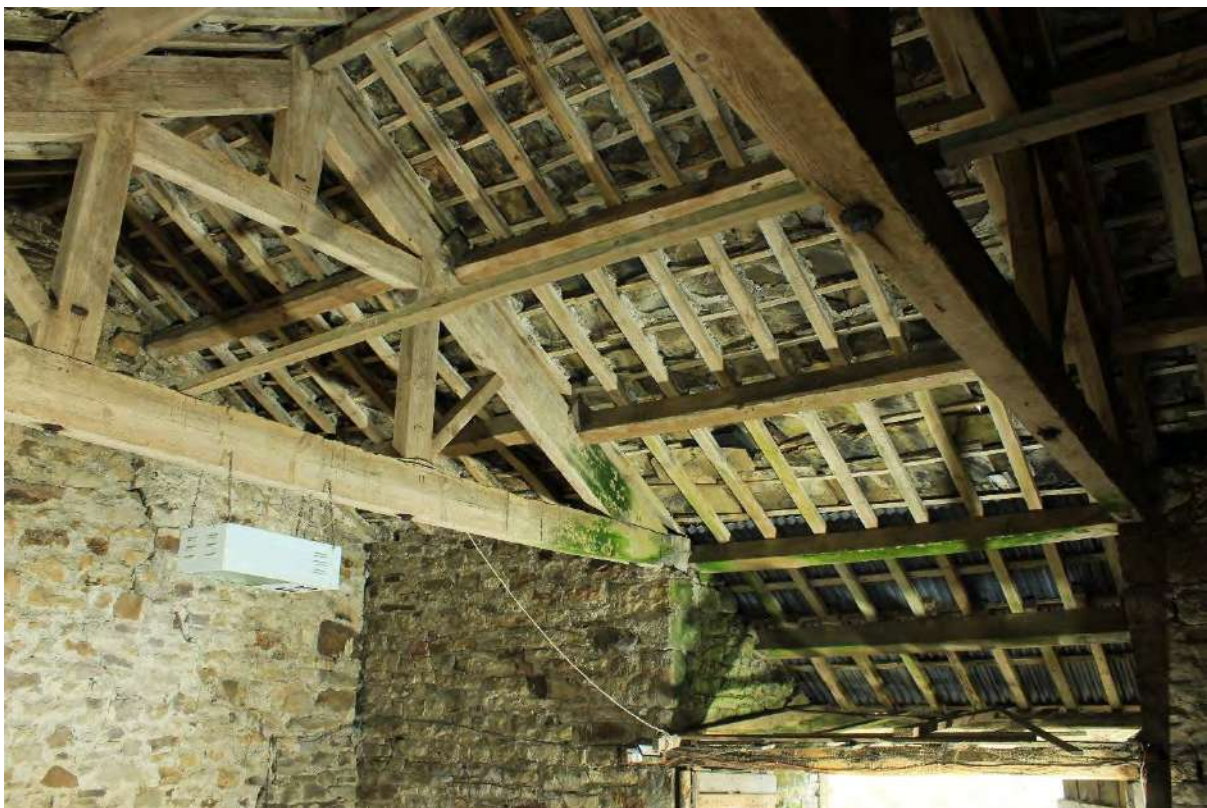
Plate 46 East roof truss in Building A, looking south-east
