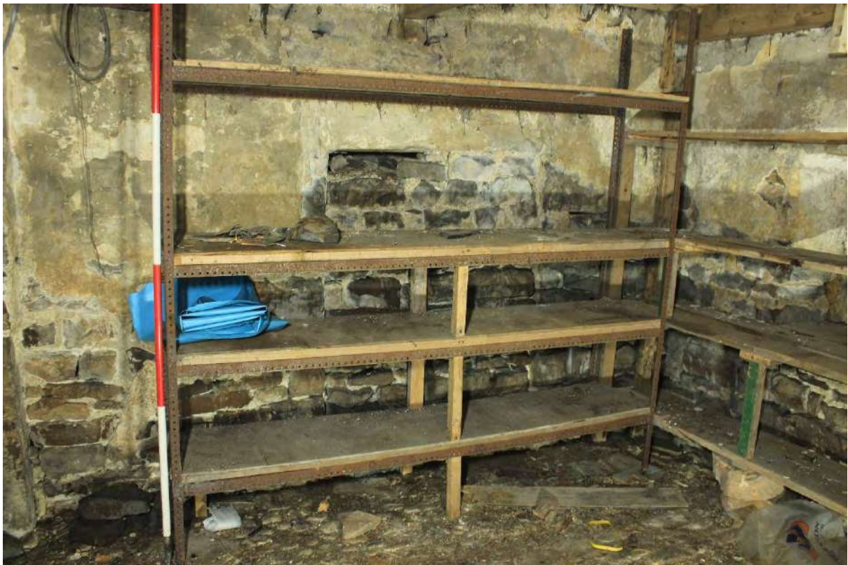
Plate 32c Blocked opening in the west wall of Bay 4 of Building A
