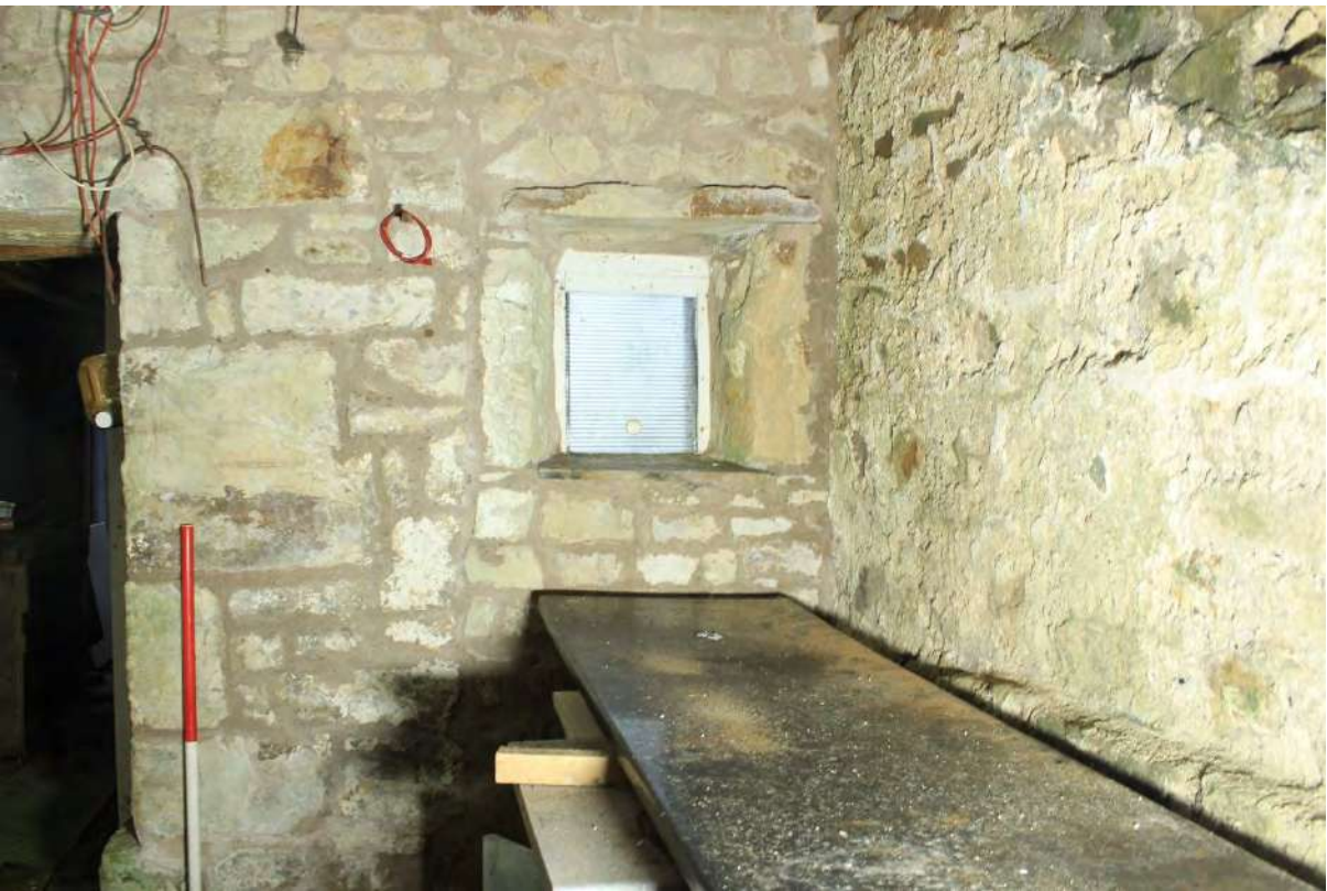
Plate 37a East and south walls of the outshot extension
