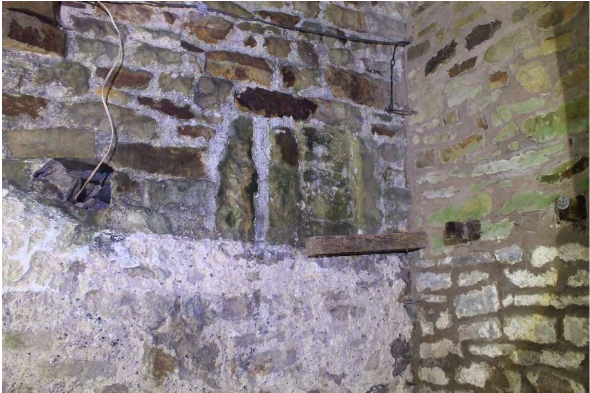
Plate 38 Infilled window opening in the south wall of the outshot extension
