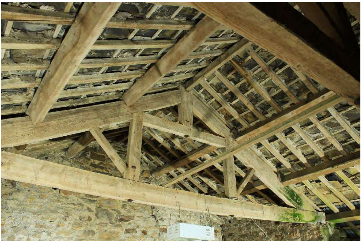
Plate 28 Queen post roof truss
