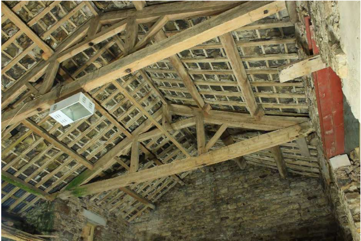
Plate 29 Queen post roof trusses
