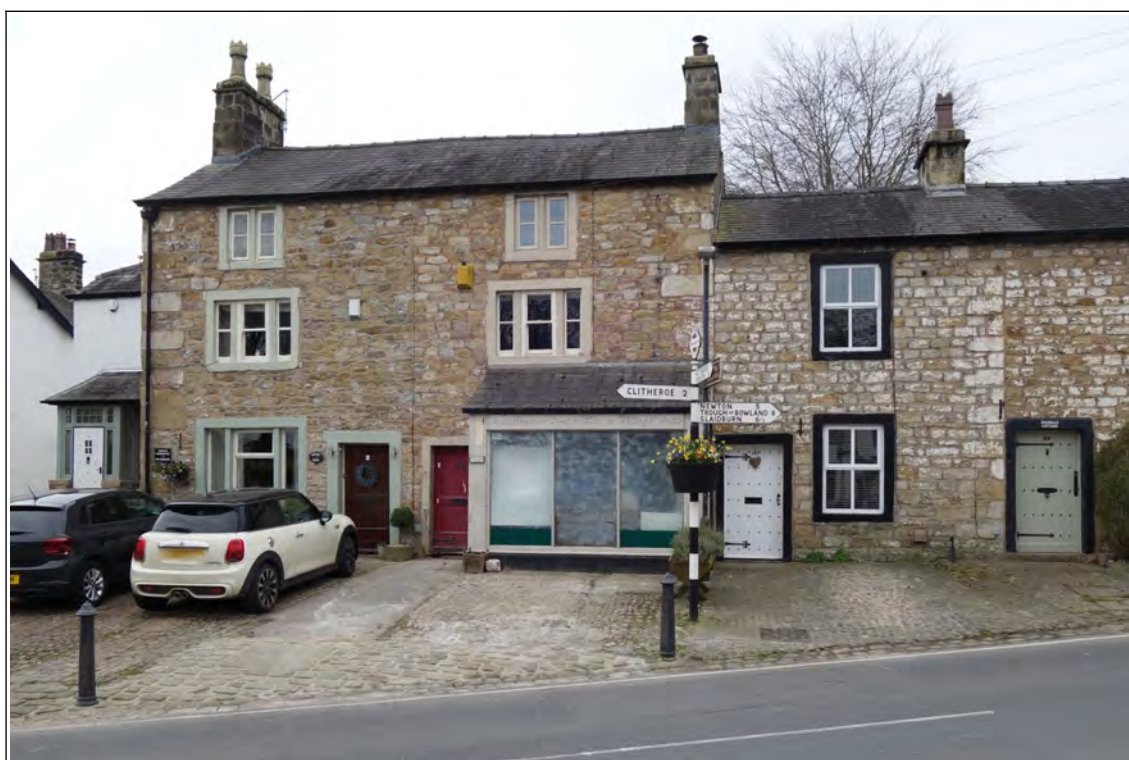
83 The Square (centre), in its immediate setting
