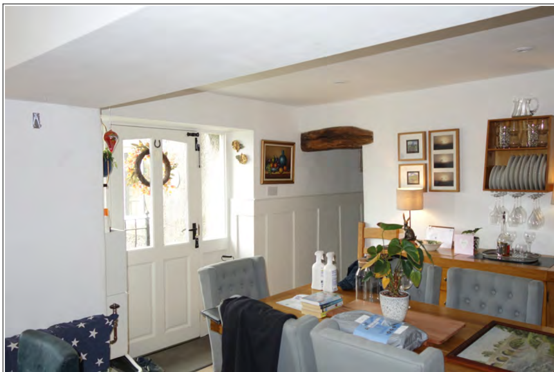
First floor, back room, looking north; beam immediately overhead carries original back wall
