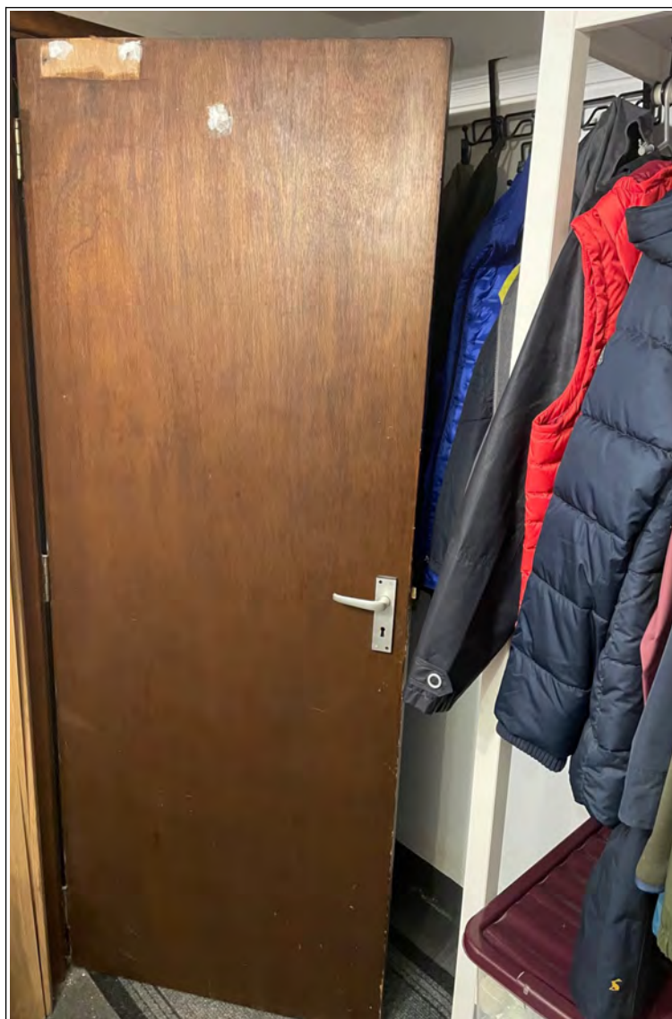
1980s ground floor door, to rear of shop
