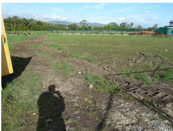
Photograph 6: Looking north-west from the site entrance, with the re-sown area and access track visible.
