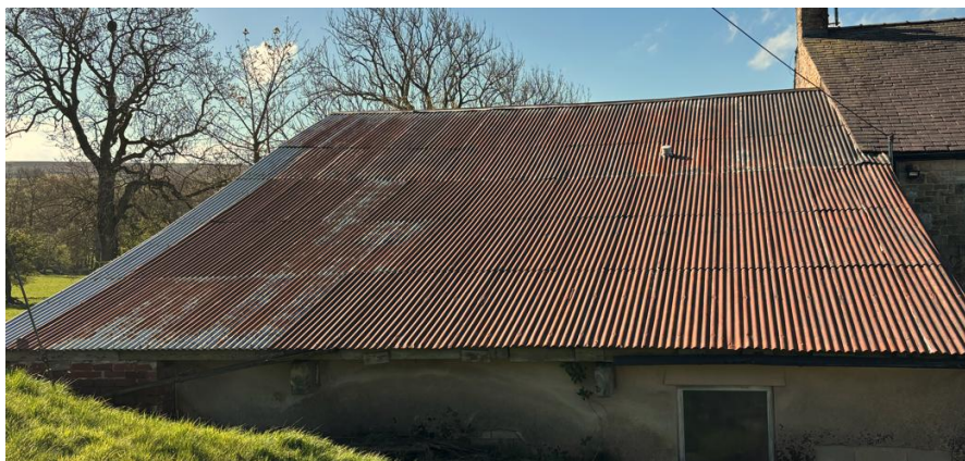
Photograph (6) – North elevation roof condition
