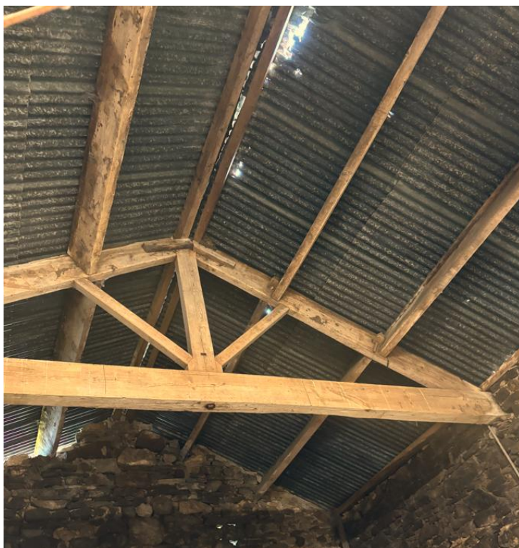
Photograph (7) – Showing the condition of the roof structure
