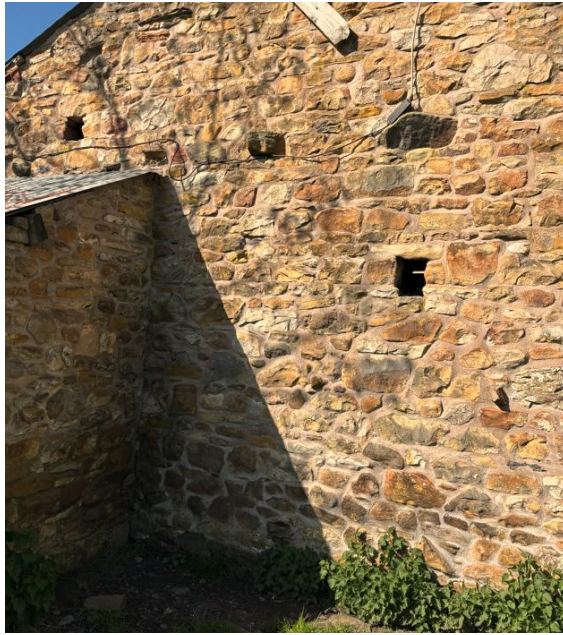
Photograph (2) – East elevation wall
