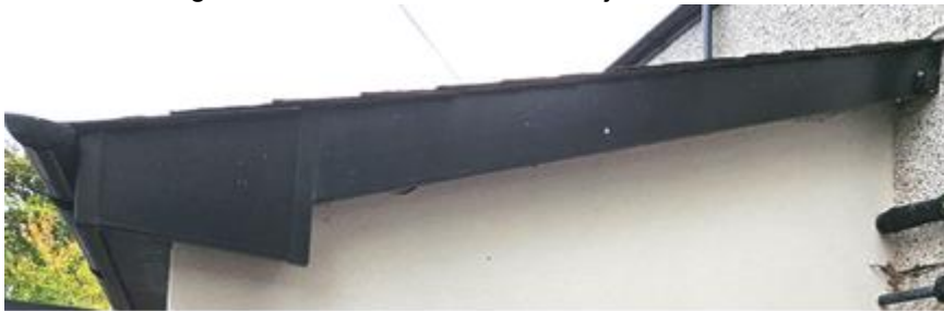
The main roof is a hipped blue slate structure. With a dormer formed in the hipped side of the roof.
