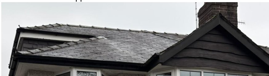
The overhang to the eaves has timber fascia's with boarded soffits.
