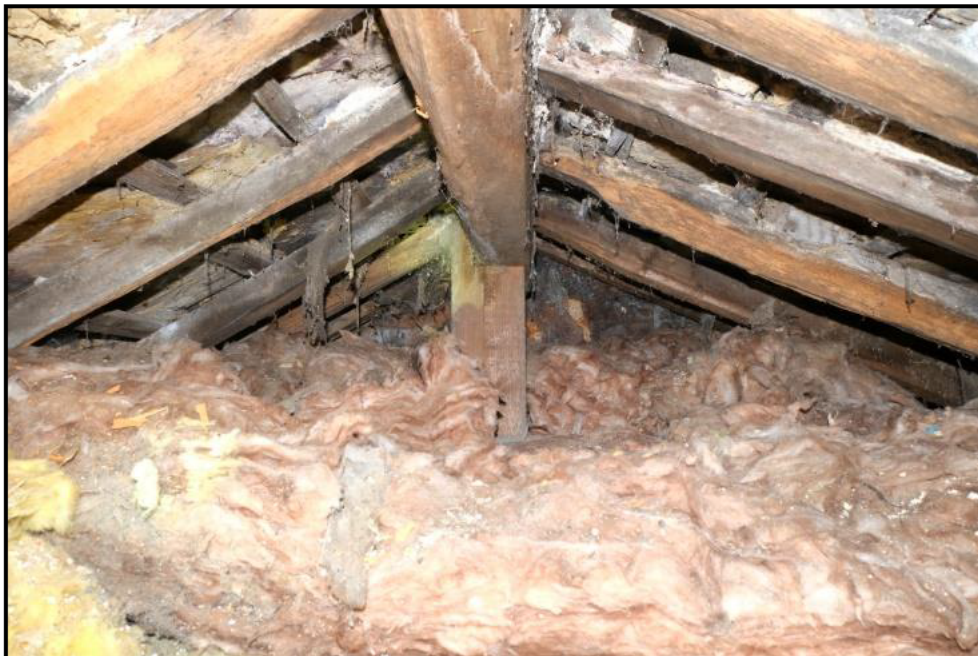
Image showing shallow roof void, no liner and deep rock wool present.
