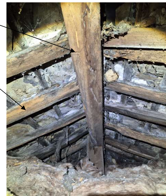
EXISTING RIDGE BEAM AND RAFTER
