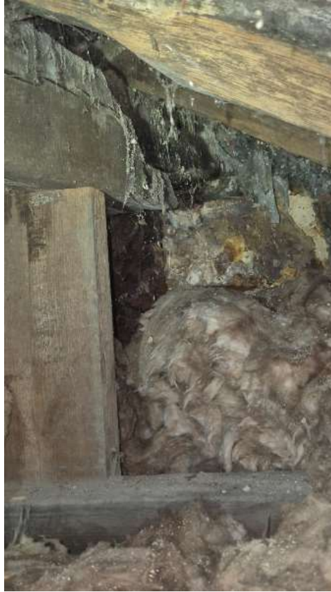
Figure 2: Ridge beam support installed by others.
