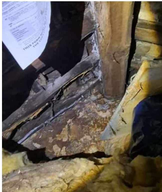
Figure 3: ridge beam supported by party wall.
