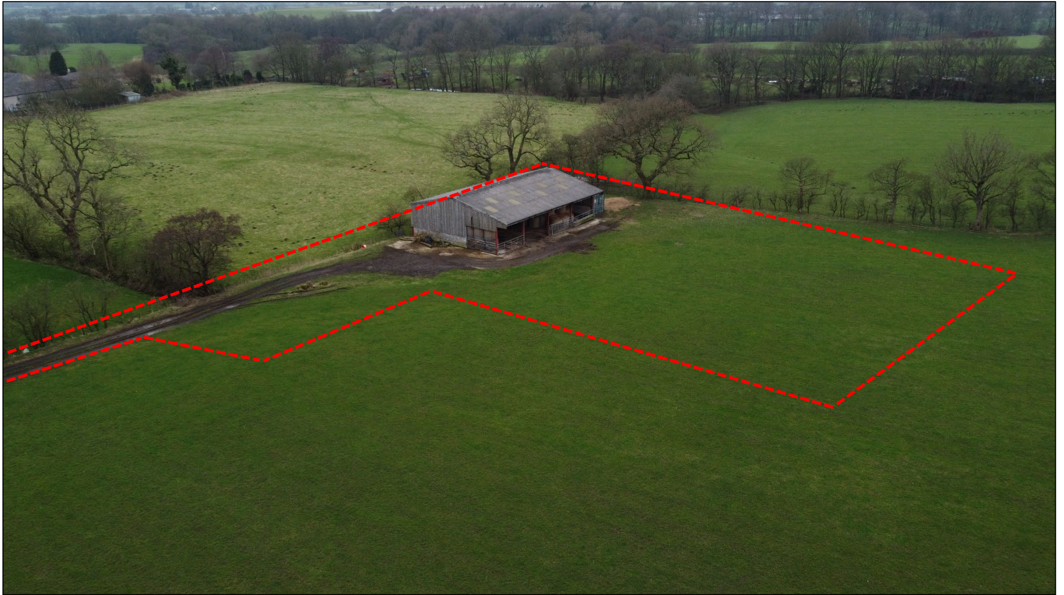
Figure 5b- Aerial view of the core development area (looking south-west)
