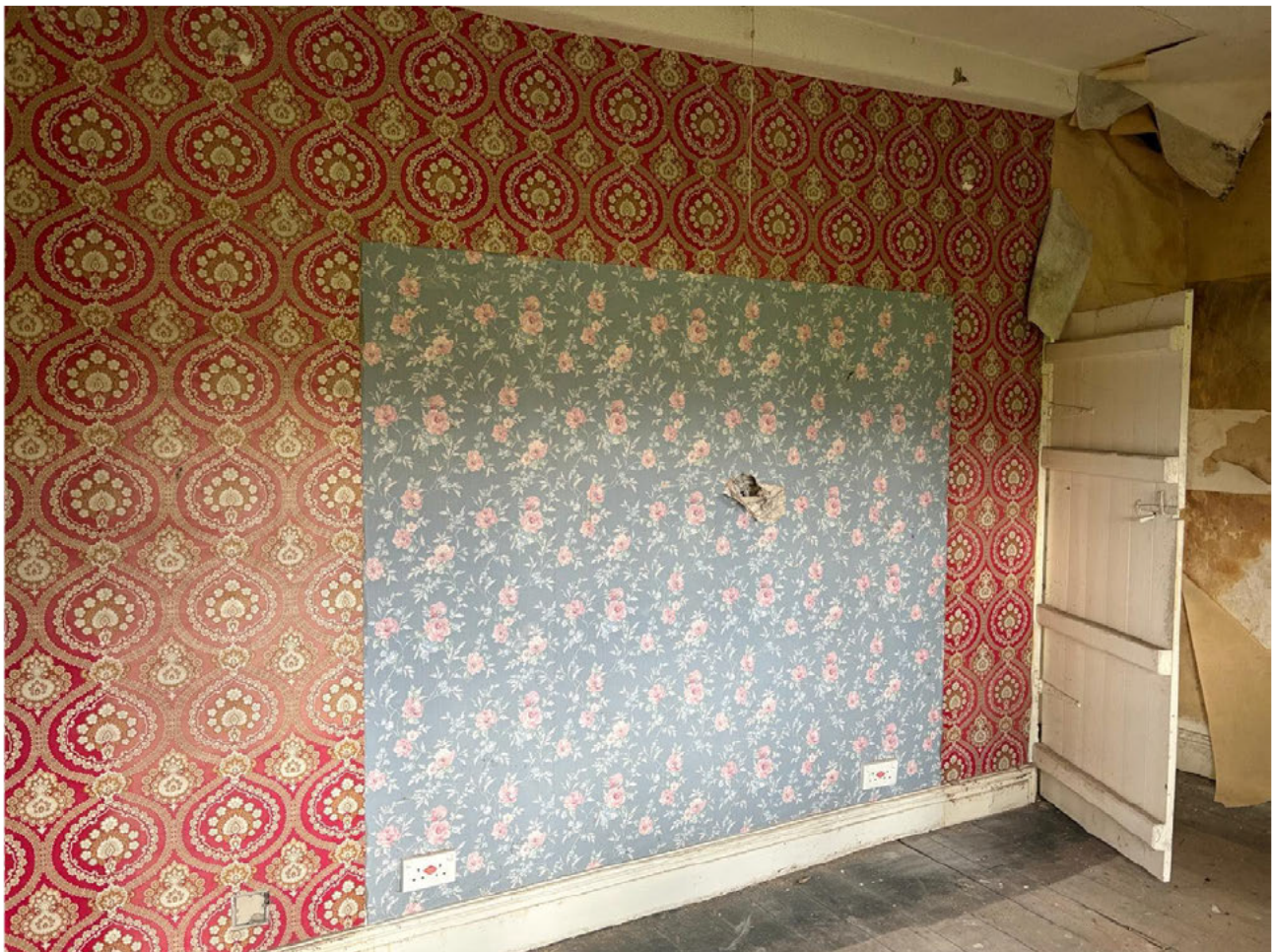
Plate 9 - Internal ground floor partition wall
