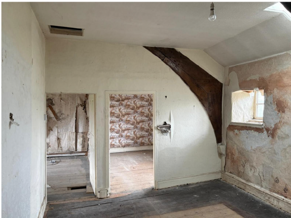
Plate 12 - Roof structure visible within first floor hall
