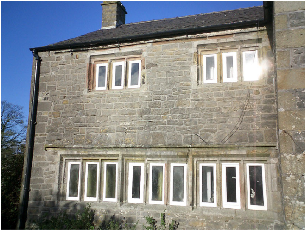
Plate 6 - Windows on the front elevation, left of the porch. The continuous horizontal banding evident above the windows. The king mullions can be seen dividing the 9-lights on the ground floor
