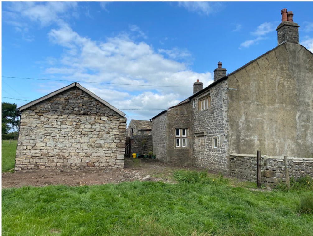
Plate 2: The rear of Park House Farm from the west, the garage building is to the left
