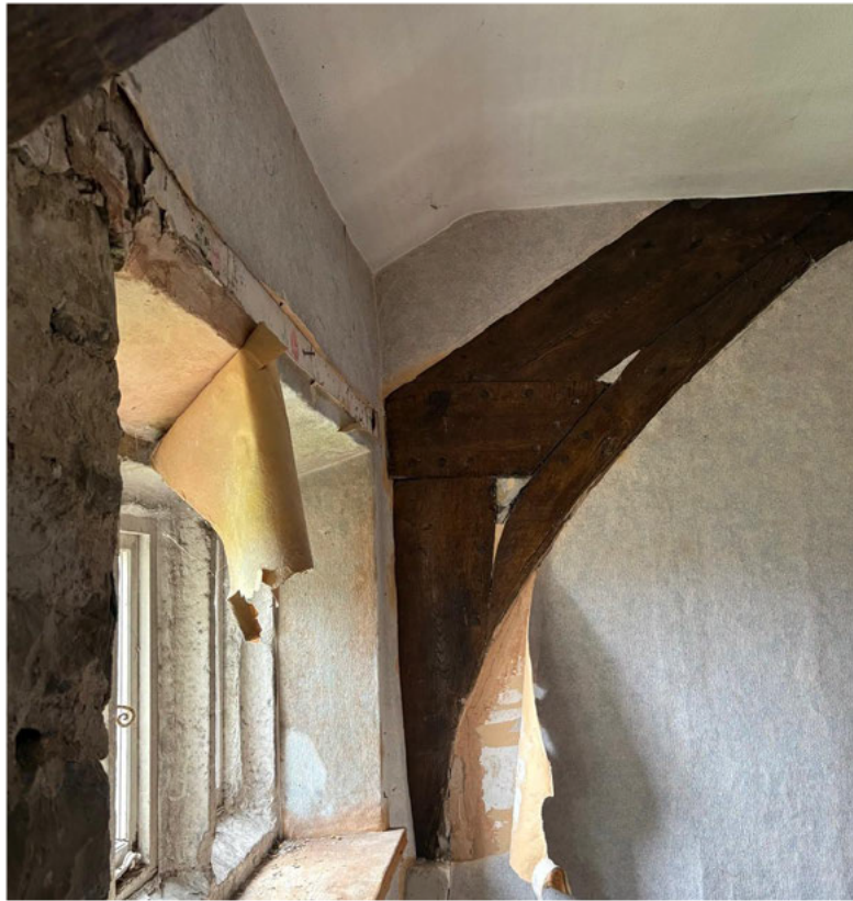
Plate 11 – Roof structure, principal rafter with bracing visible
