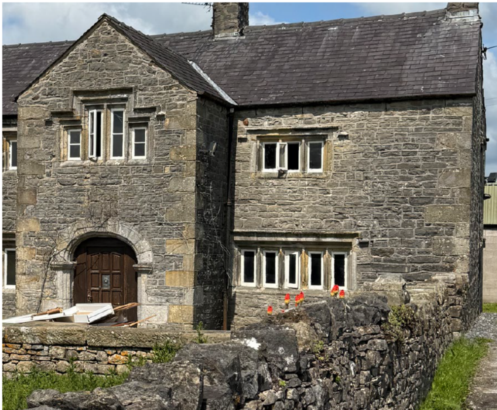
Plate 7 - The porch and right-hand side of the front elevation. The hood moulding with returned ends is clear above the windows
