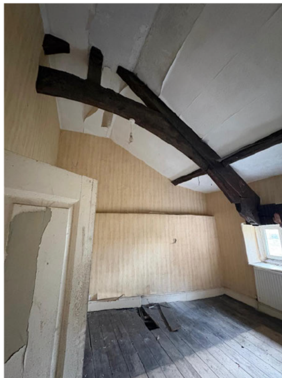
Plate 14 – Room in context with the truss has been cut to accommodate window
