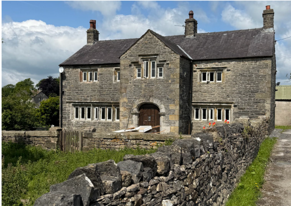
Plate 5 - Park Farm House, front (south) elevation
